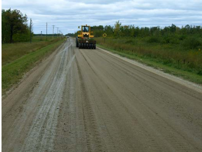
Figure 4 Rolling treated aggregate surface, Pennington 72.
