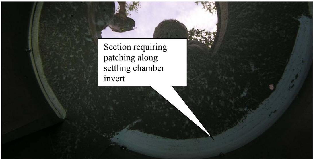
**Figure C.16:** View of the base of the stainless steel cylinder serving as a swirl chamber and new sealant applied (thicker section along lower right) to minimize improper hydraulics.
