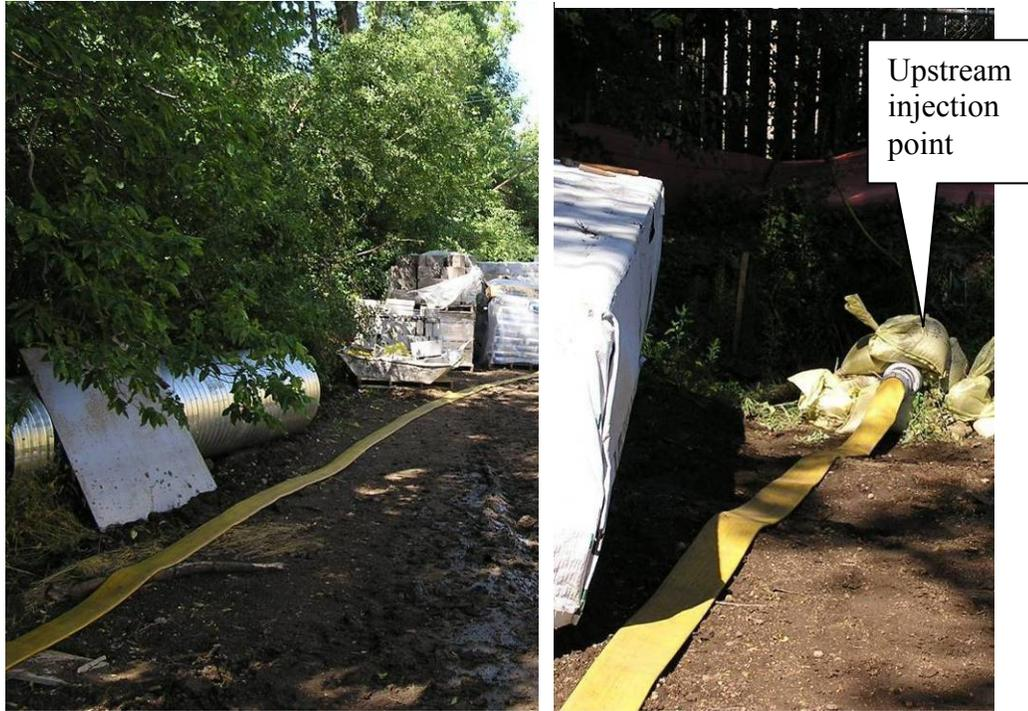
**Figure C.12:** Depiction of 4 inch fire hose used to span about 150 feet from the hydrant (not shown, see Figure C.11) to the influent injection point (right).
