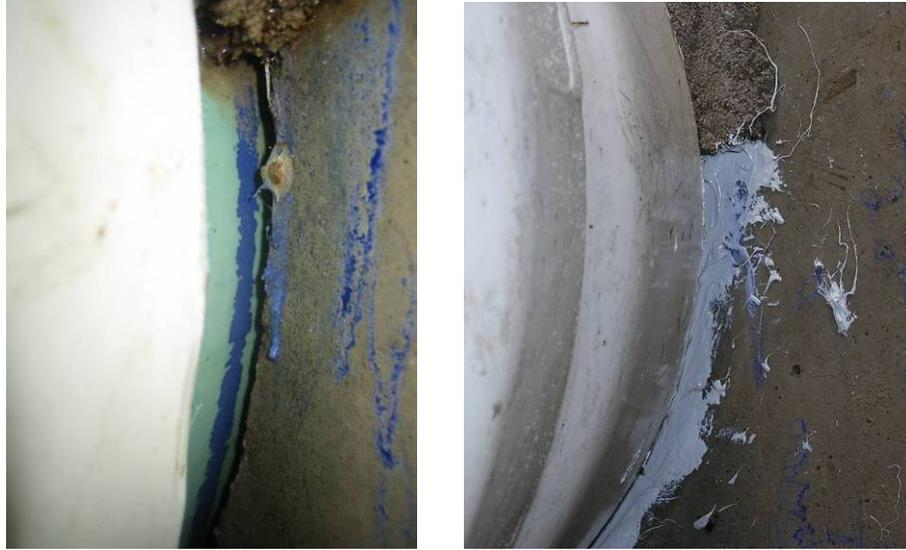
**Figure C.8:** (Left) Water was initially able to flow between treatment manholes through an approximate 1.3 cm ( ½ in) gap between the PVC pipe and concrete manhole wall. (Right) The leaking gap was patched with Vulcum polyurethane to ensure proper system hydraulics.
