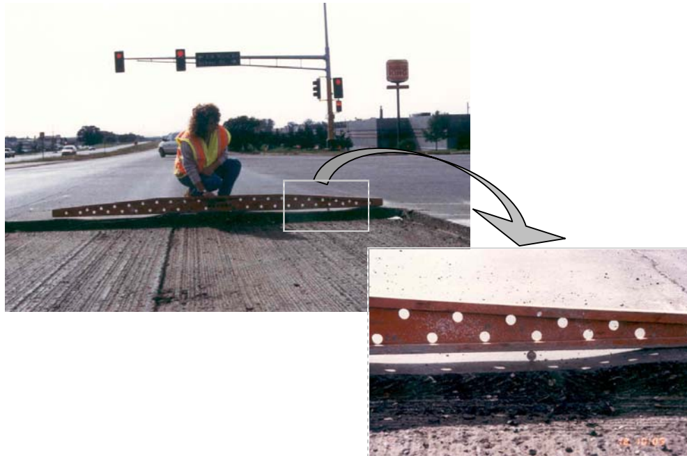
Figure 2.1. Ruts at the Jackson Street intersection prior to the UTW overlay.
