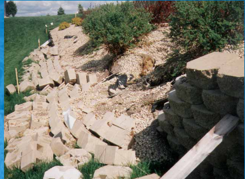
Incorrect reinforcement
