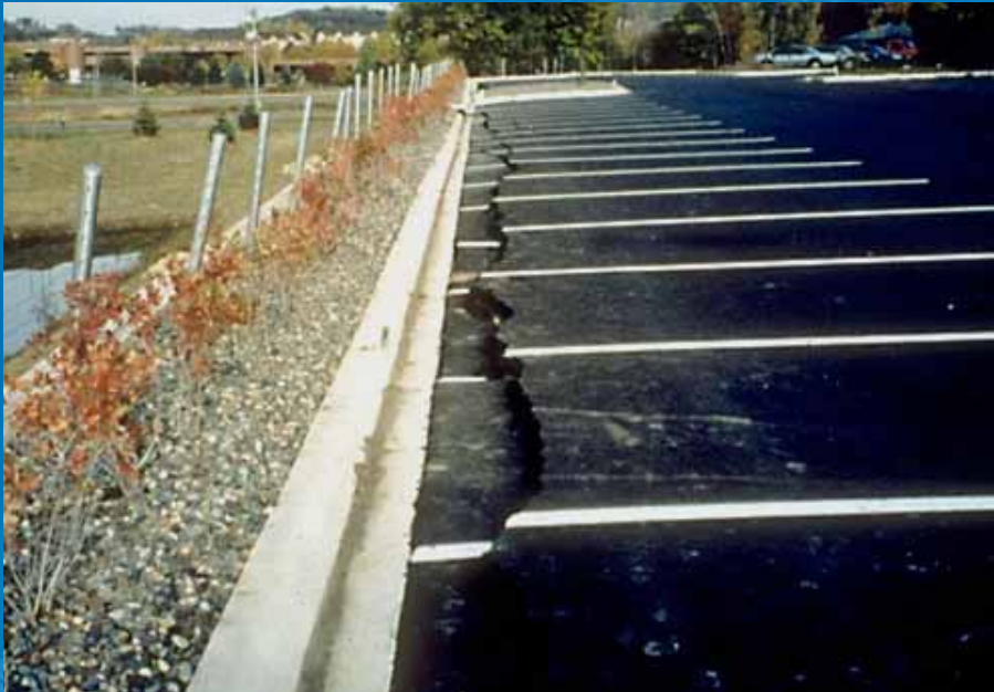
Poor Compaction
