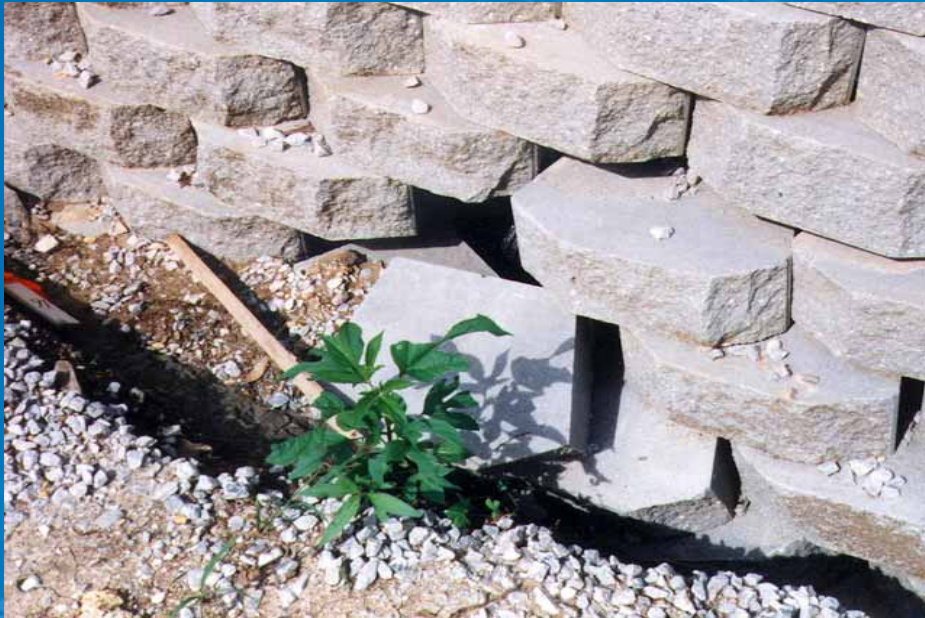
Incorrect drainage
