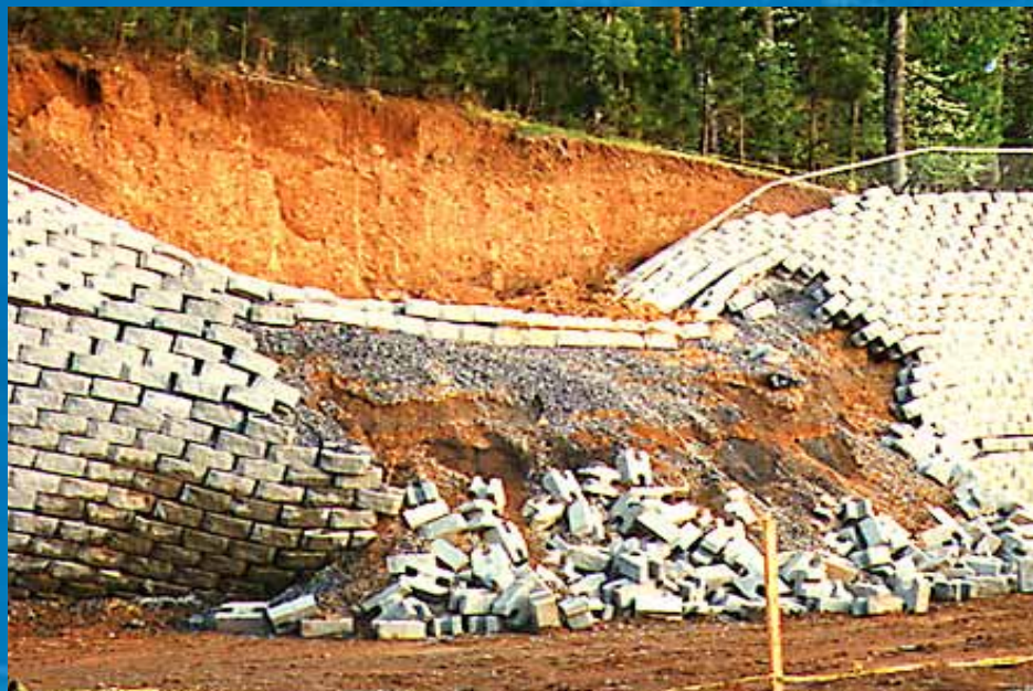
No reinforcement
