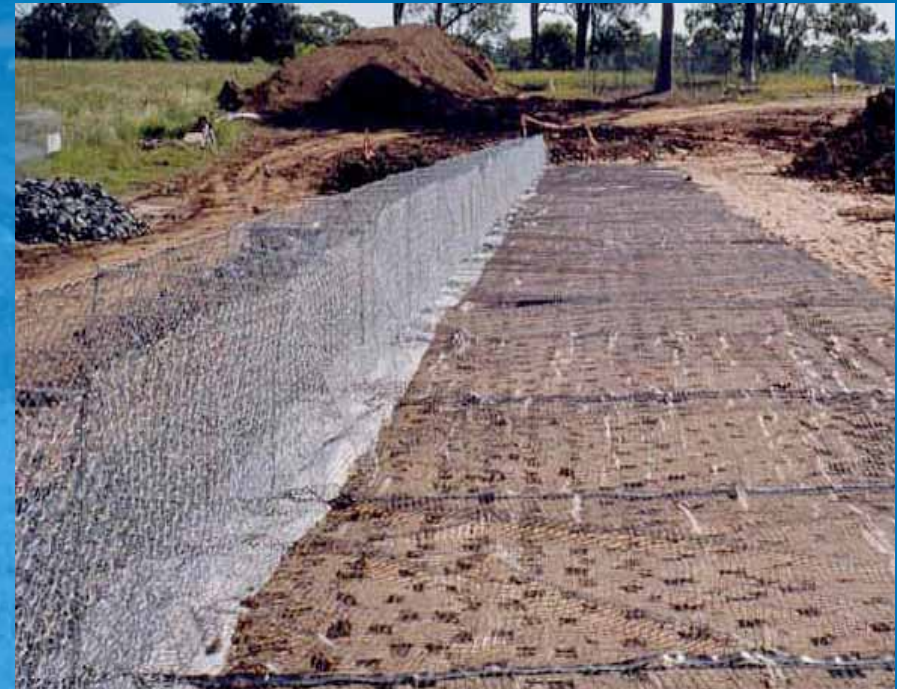
Gabion Basket Facing
