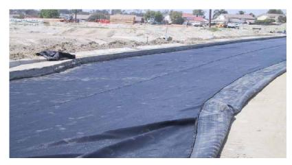
Among the geosynthetics uses described was a geotextile laid over a clay subgrade. This allows moisture to drain through but keeps the clay from migrating up into the roadway base and affecting pavement performance.
