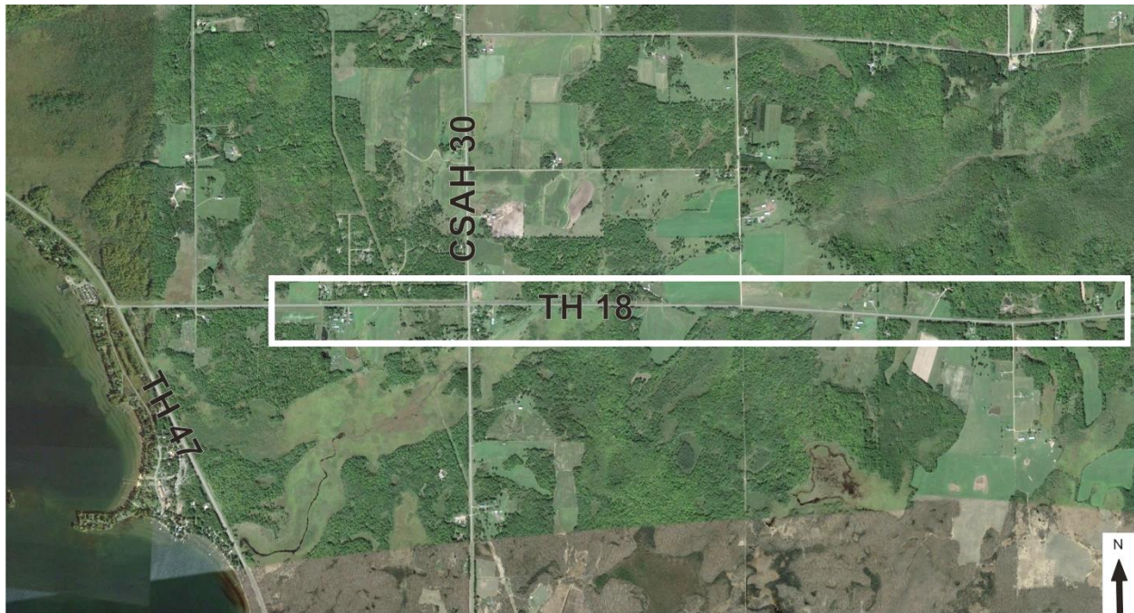
Figure 5.1 Test Area for Rumble Strips
