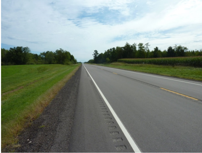
Figure 5.2 TH 18 Typical Corridor View
