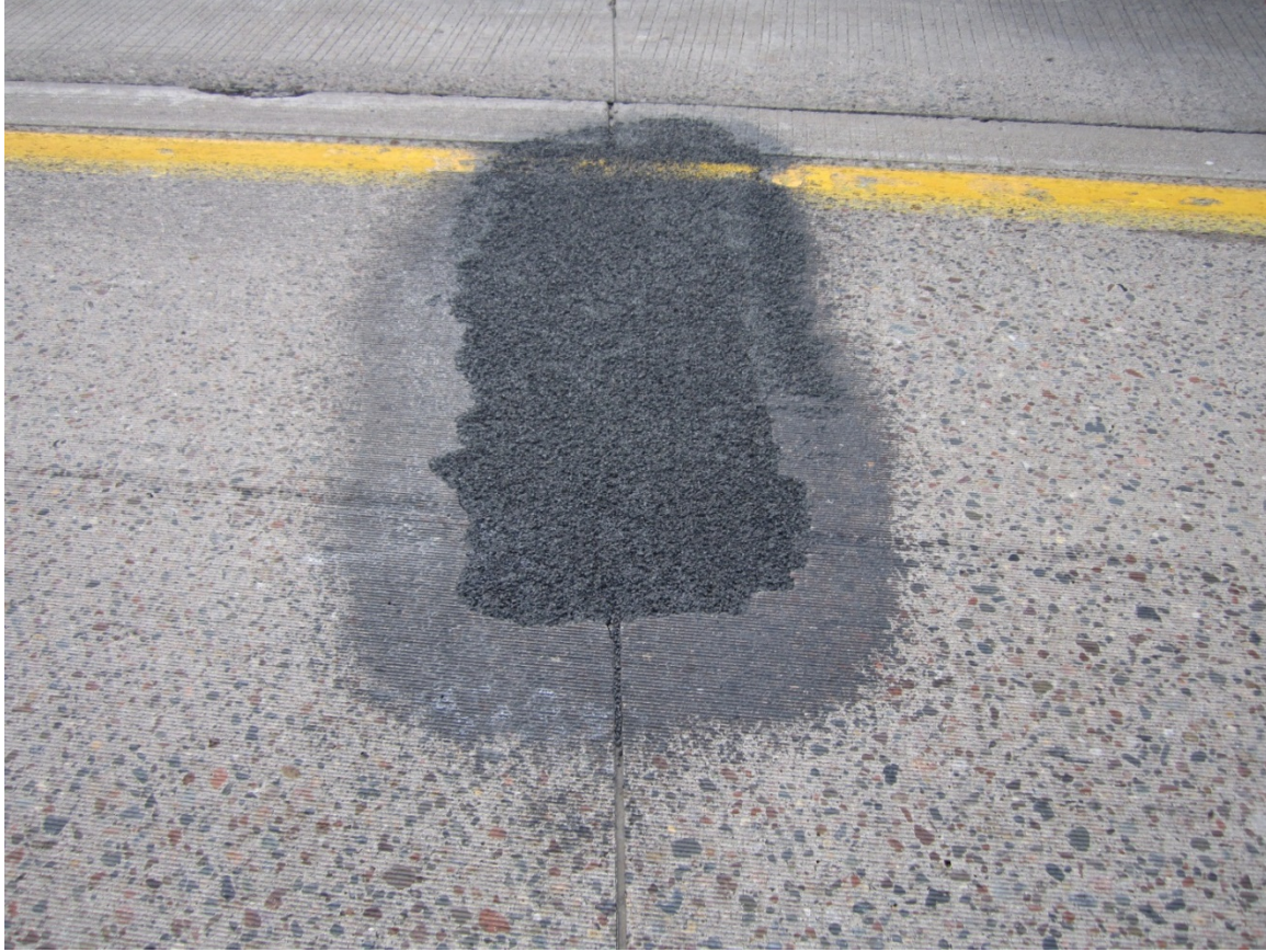
Figure 1.5. Typical MnROAD partial-depth repair with asphalt-based material.
