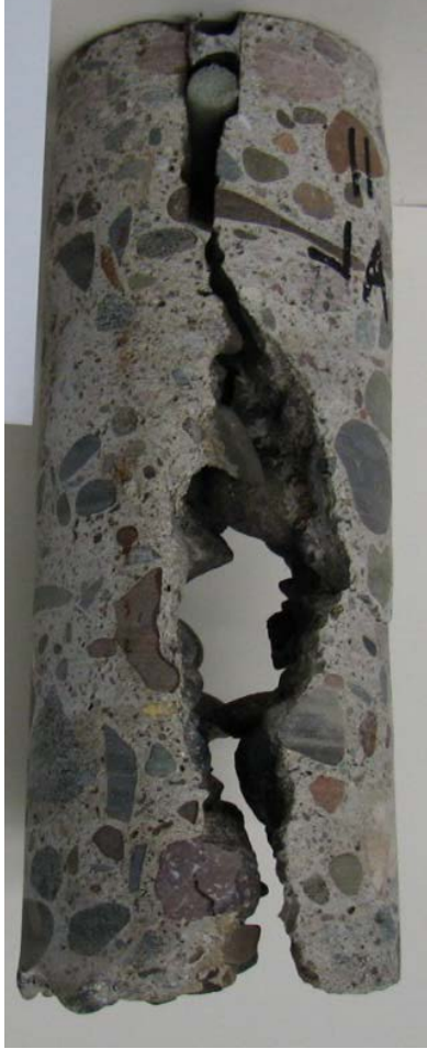
Figure 1.3. Distress at mid-depth and bottom of transverse joint placed on slow draining base layer [3].
