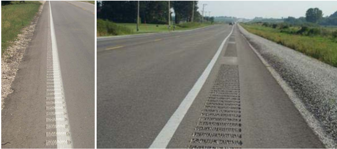
Figure 2. Shoulder Rumble Strips
