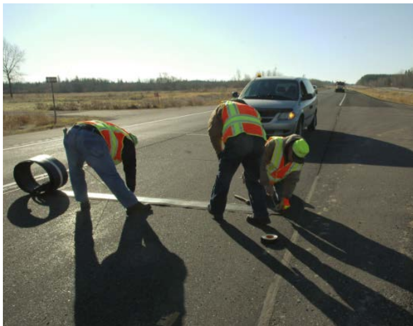
Figure 4: Crew Installing a Weigh-Pad along Trunk Highway 53 in Cotton, Minnesota
