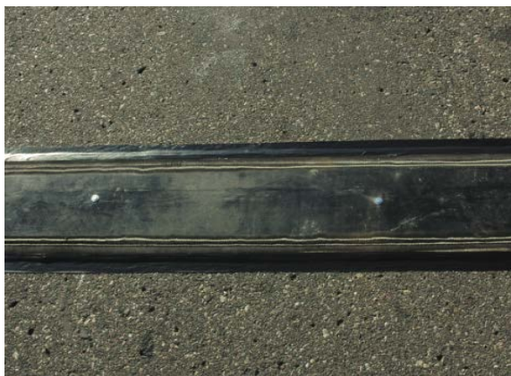
Figure 5: Segment of a Properly Installed Weigh-Pad
