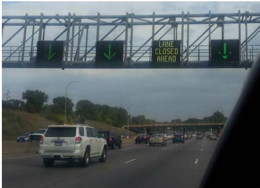
Figure 1-1. Gantry displaying ILCS messages.
