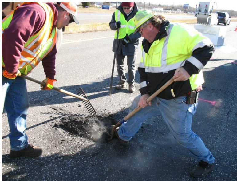
Figure 3.7. Working microwave-heated pavement with shovel.
