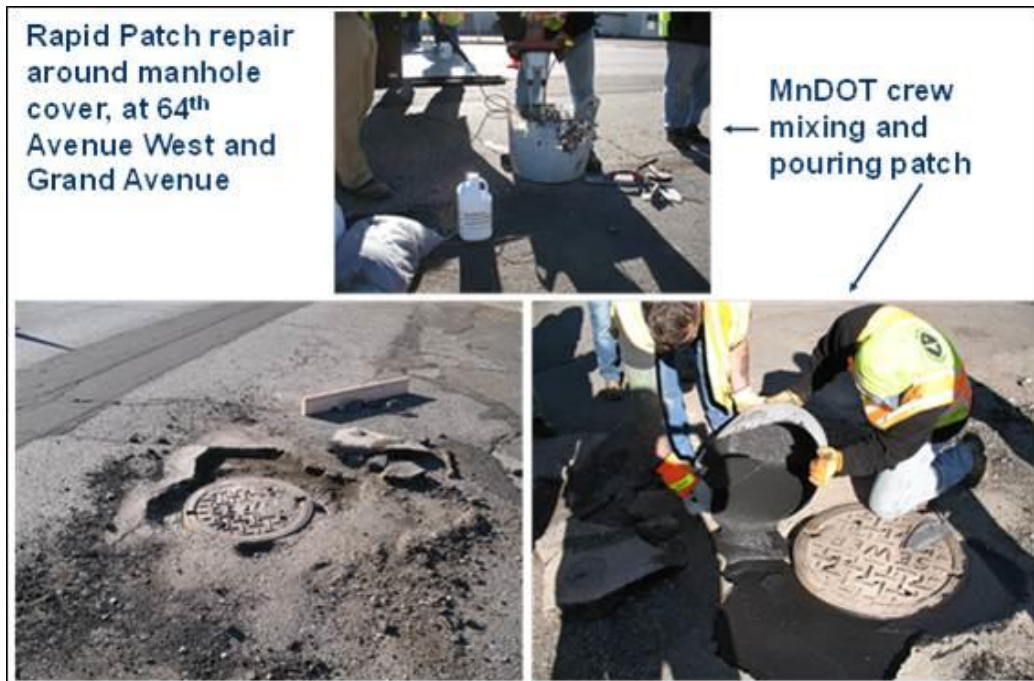
Figure 3.40. Rapid Patch manhole repair: 64th Avenue West and Grand Avenue.
