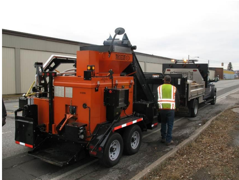
Figure 3.8. Stepp Asphalt Recycler, Grand Avenue (Hwy. 23), Duluth: November 13, 2012.
