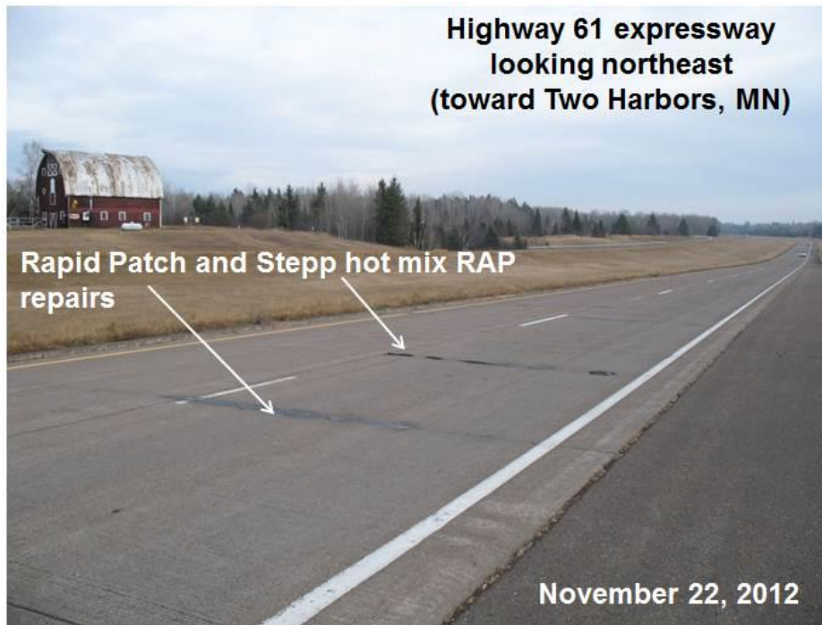
Figure 3.65. View of Highway 61 expressway Rapid Patch and Stepp hot mix RAP repairs: November 22, 2012.
