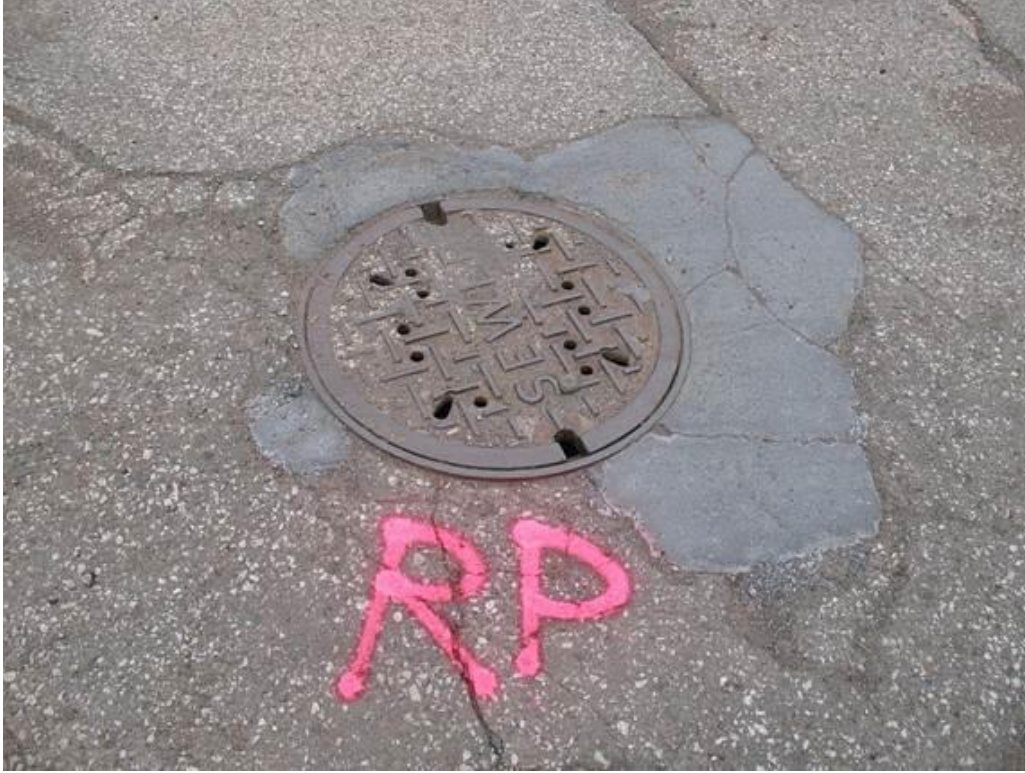
Figure 3.43. Rapid Patch manhole repair: Condition on July 30, 2013.
