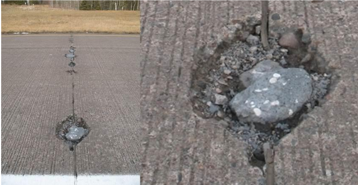
Figure 3.69. Failing condition of a Highway 61 Rapid Patch repair 2 years after installation: December 26, 2014.
