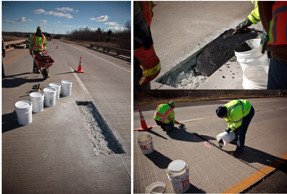
Figure 3.70. Installation of Highway 169 Keewatin bridge deck Rapid Patch repair: November 4, 2010.
