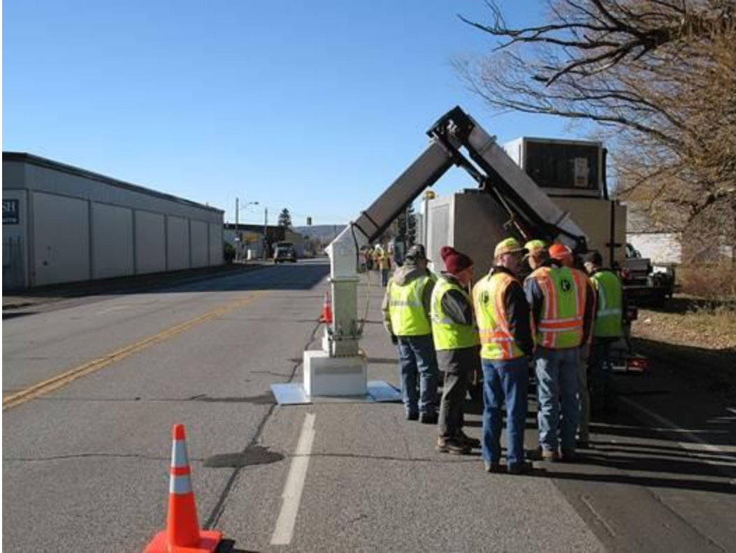
Figure 3.47. Preparing Grand Avenue Rapid Patch repair with microwave unit: October 31, 2012.
