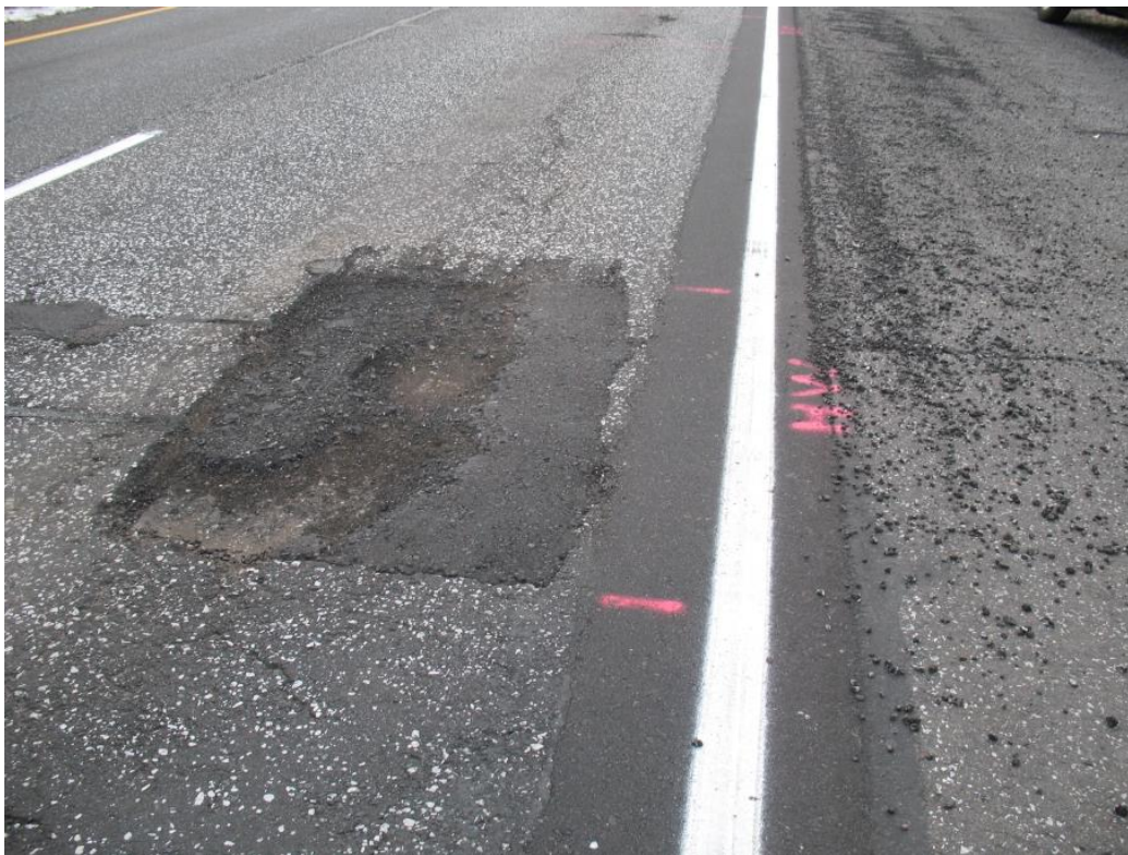
Figure 3.17. HeatWurx repair #2, Highway 53 (Monaco Air sign) location: failing condition on November 13, 2012.
