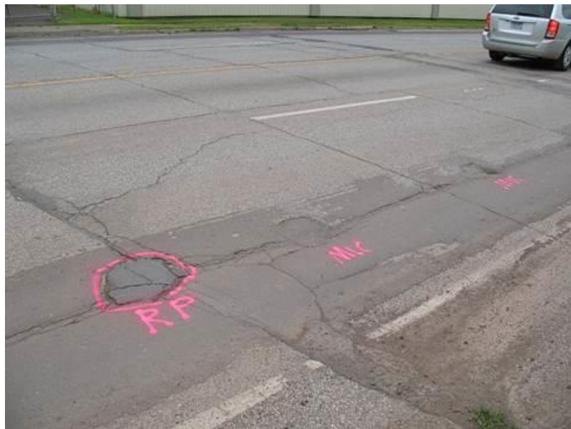
Figure 3.53. Rapid Patch repair condition on July 30, 2013. Replaced microwave repairs to the right.
