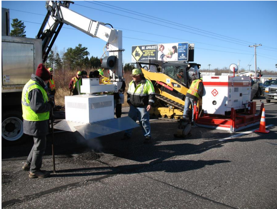
Figure 3.5. Field trial comparison of microwave (left) and HeatWurx (right): October 30, 2012.
