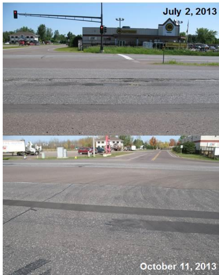
Figure 3.27. Mill-and-fill of Hwy 53/Cirrus Drive repair location.
