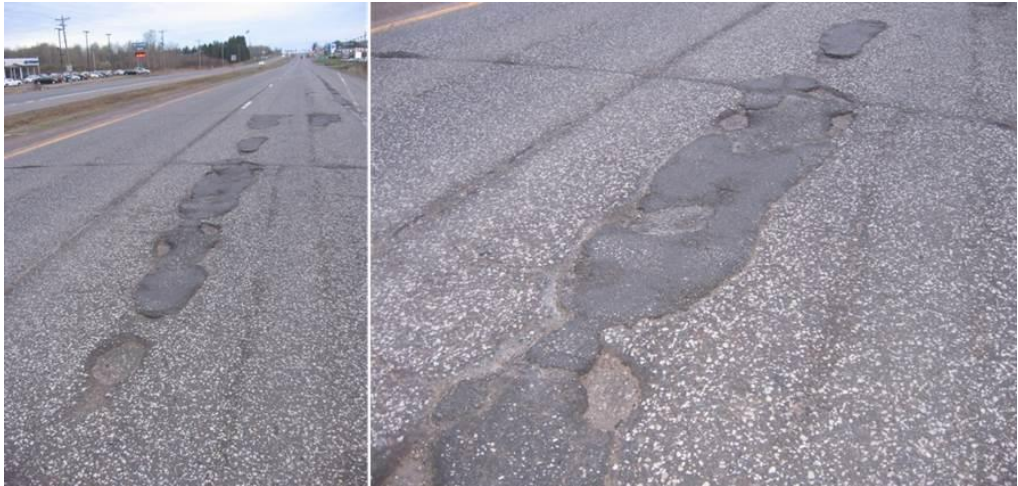
Figure 3.12. Stepp hot repair condition on May 17, 2013.
