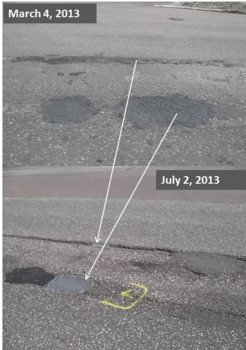
Figure 3.25. Condition of Hwy 53/Cirrus Drive Rapid Patch repair on March 4 and July 2, 2013.
