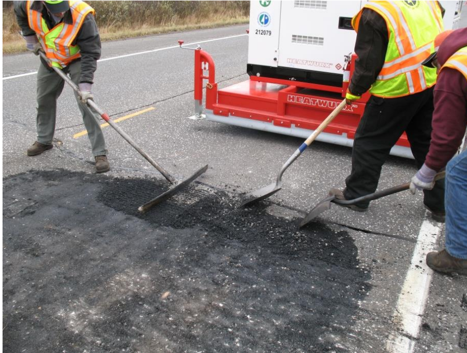
Figure 3.3. Raking heated and softened pavement following use of HeatWurx.
