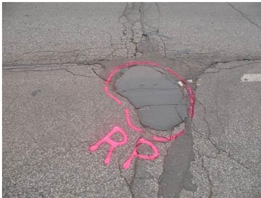
Figure 3.49. Rapid Patch repair condition, Grand Avenue driving lane: July 30, 2013.
