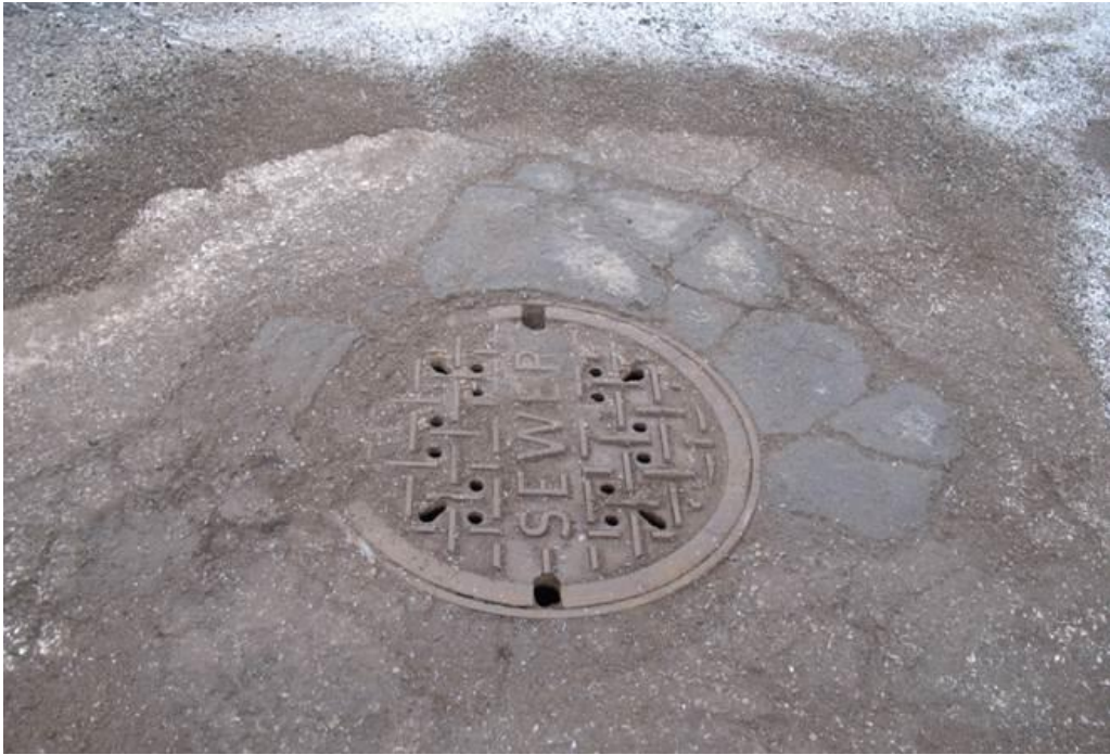
Figure 3.44. Rapid Patch manhole repair: Condition on December 26, 2014.
