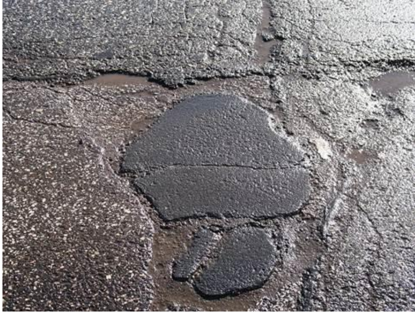
Figure 3.50. Rapid Patch repair condition, Grand Avenue driving lane: February 14, 2014.
