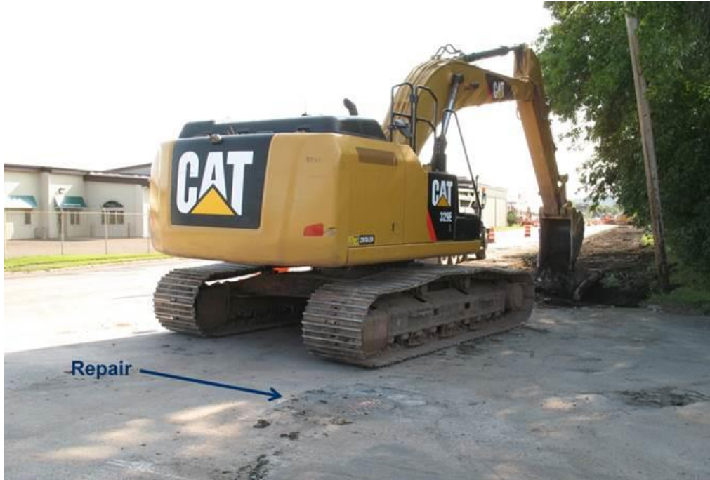
Figure 3.46. Rapid Patch manhole repair prior to removal: August 26, 2015.
