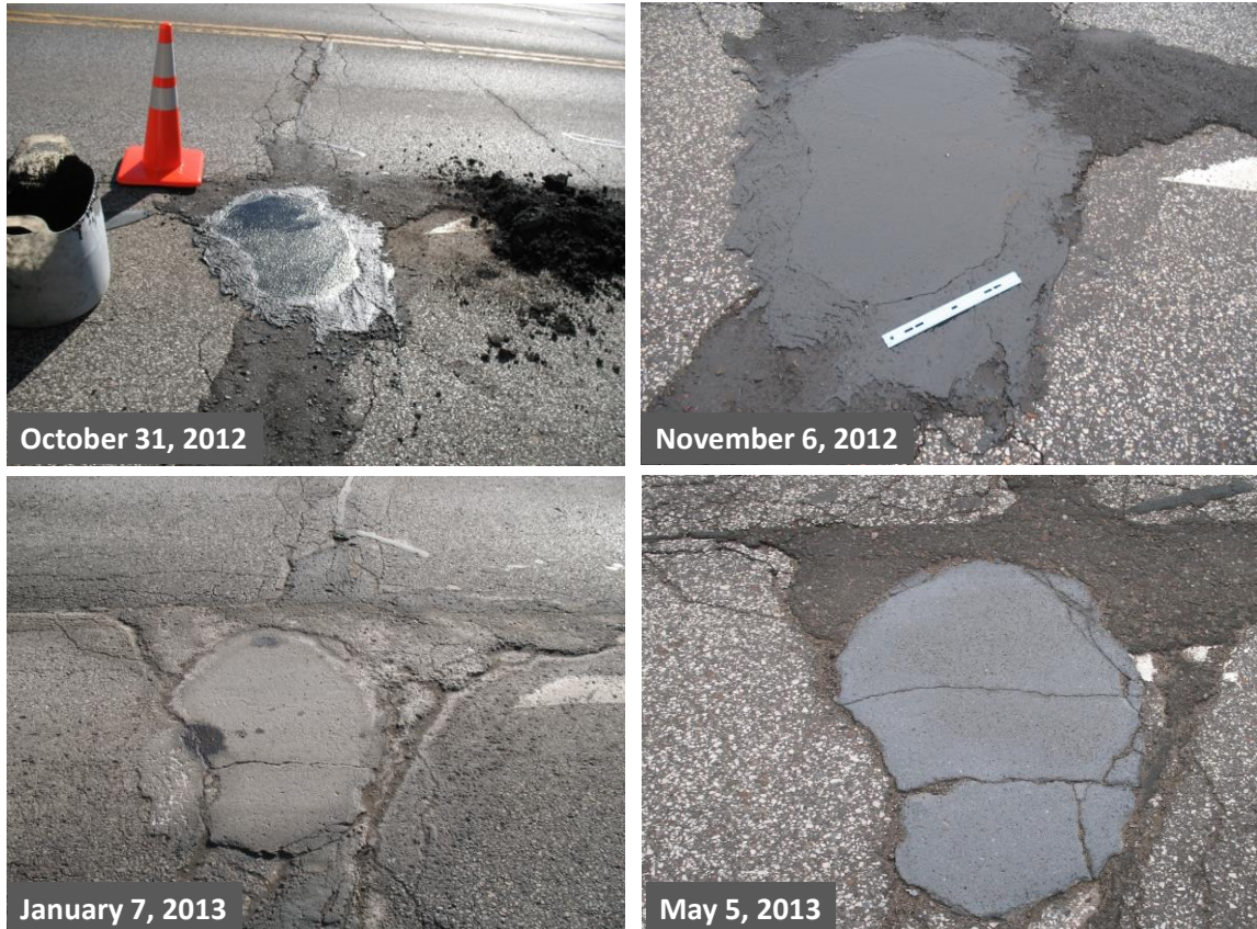
Figure 3.48. Rapid Patch repair condition over time: Grand Avenue driving lane.
