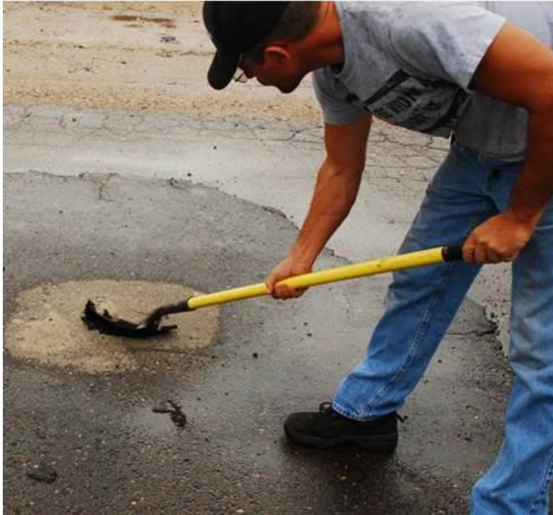
Figure 2.9. Microwave-heated pavement, easily removed with shovel (surface at 200° F).
