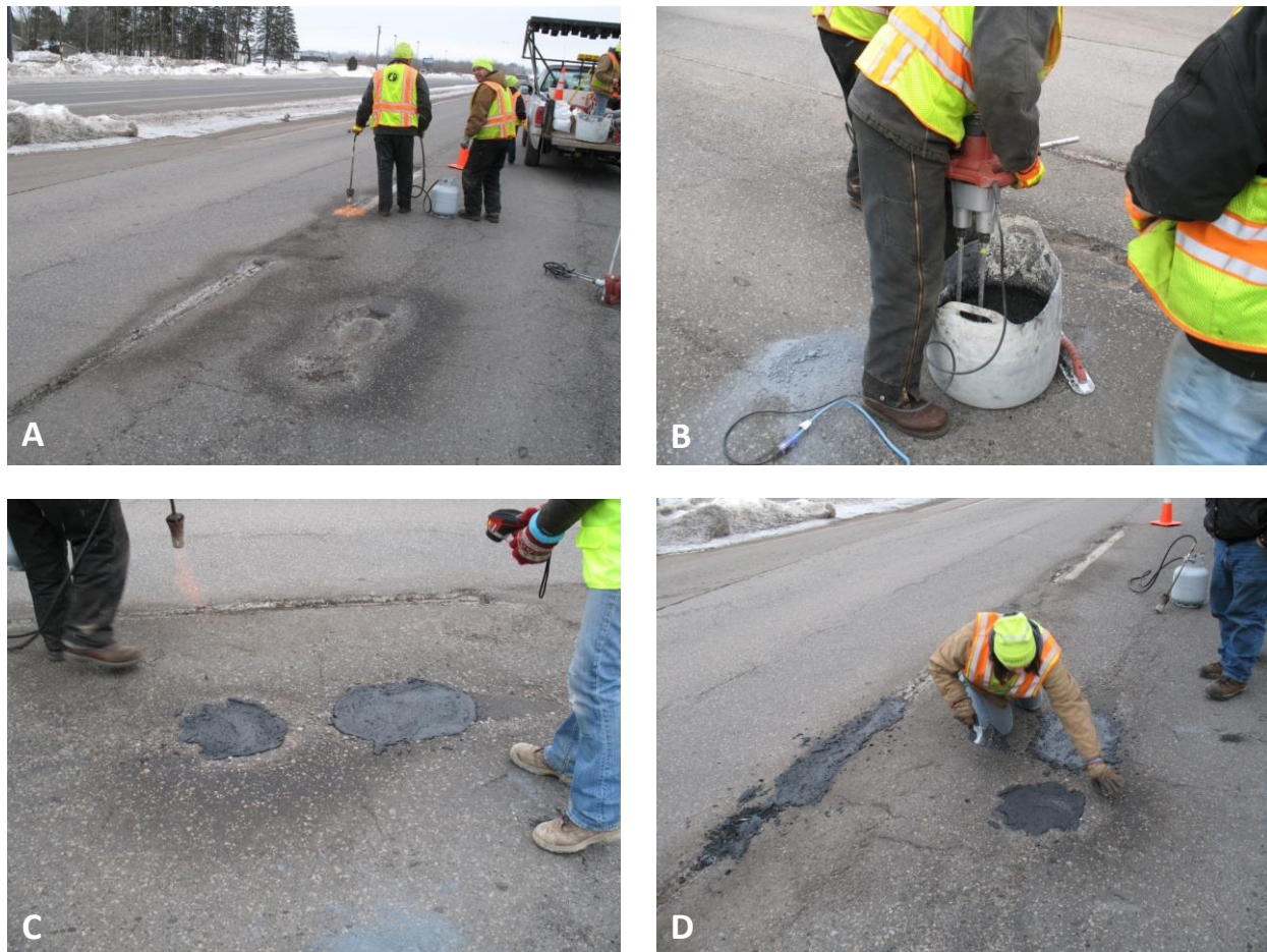
Figure 3.23. Rapid Patch preparation and repairs at Cirrus Drive/Highway 53 intersection location, March 1, 2013.
