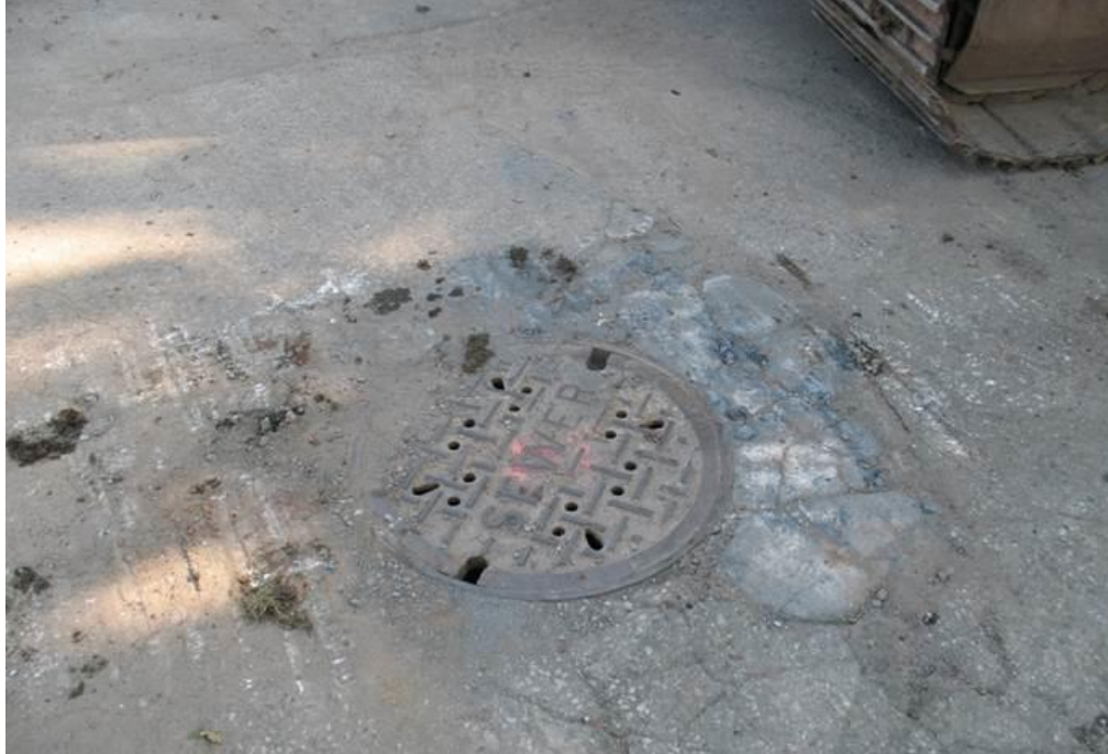
Figure 3.45. Rapid Patch manhole repair: Condition on August 26, 2015.
