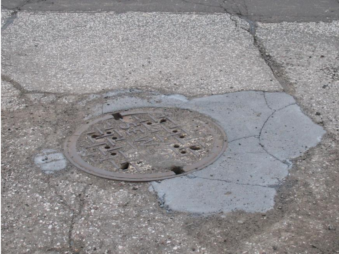
Figure 3.42. Rapid Patch manhole repair: Condition on May 5, 2013.
