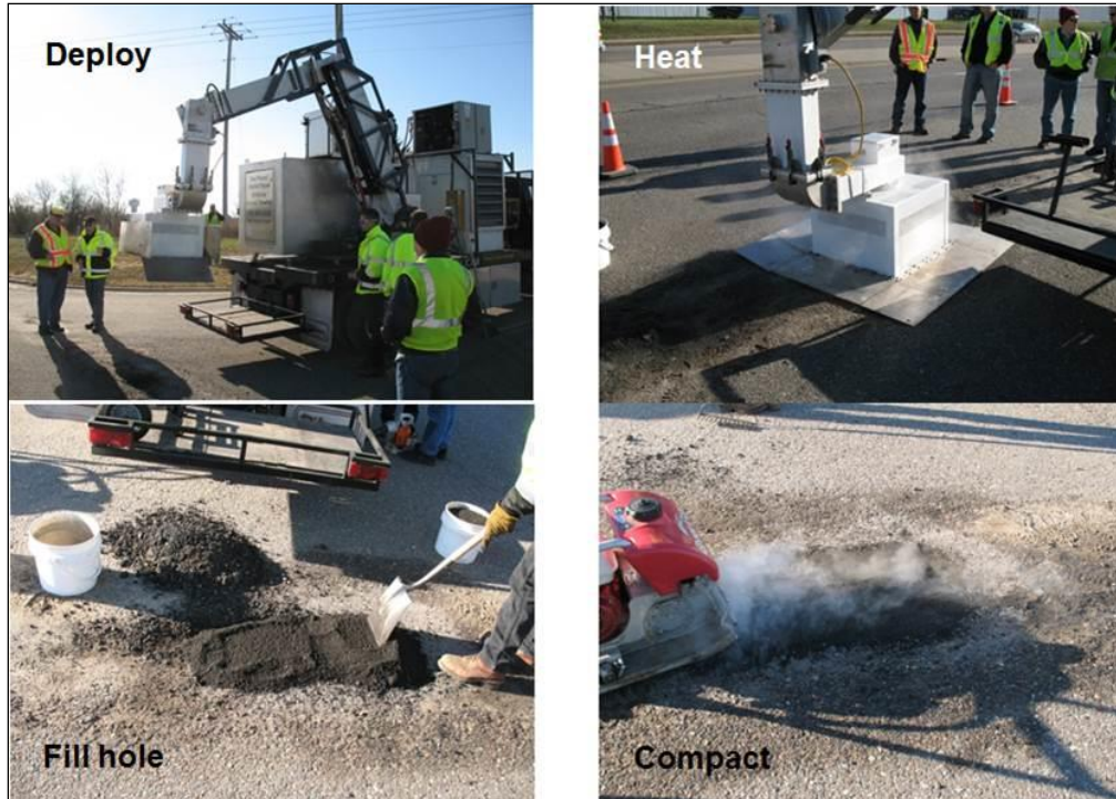
Figure 3.80. Microwave equipment and repair demonstration: November 14, 2013, Monticello, MN.
