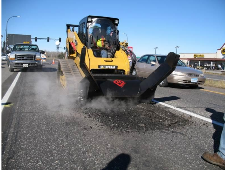
Figure 3.6. HeatWurx post-heating "tilling" of pavement.
