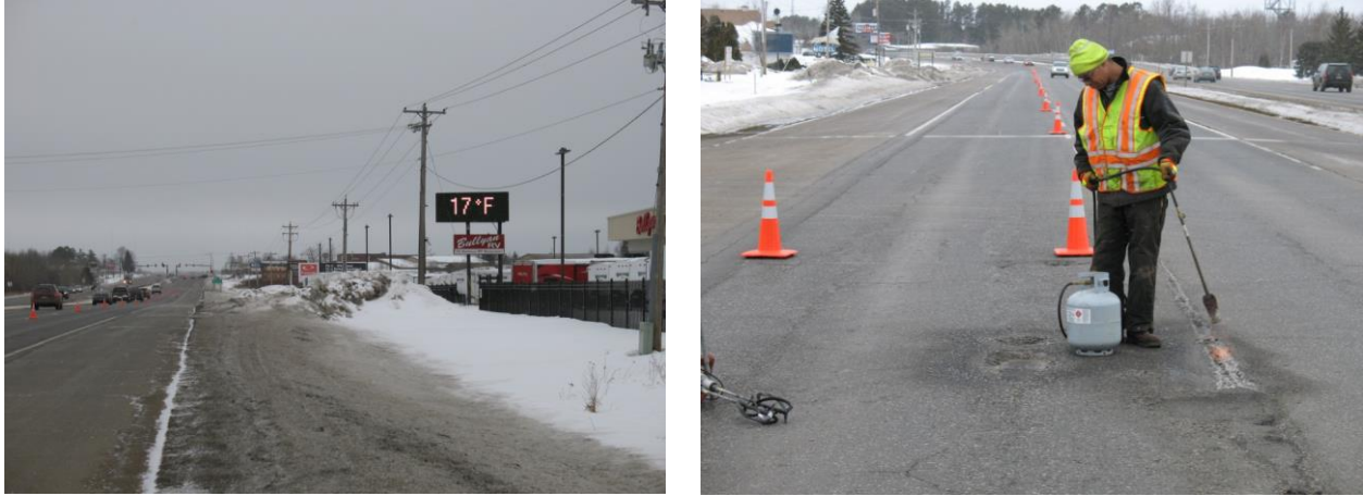
Figure 3.21. Temperature conditions (17° F; -8° C) and pavement preparation for March 1, 2013, field trial/demonstration.
