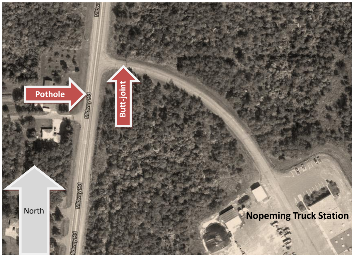
Figure 2.15. November 1, 2012, microwave repair locations (Becks Road/Midway Road Nopeming Truck Station).
