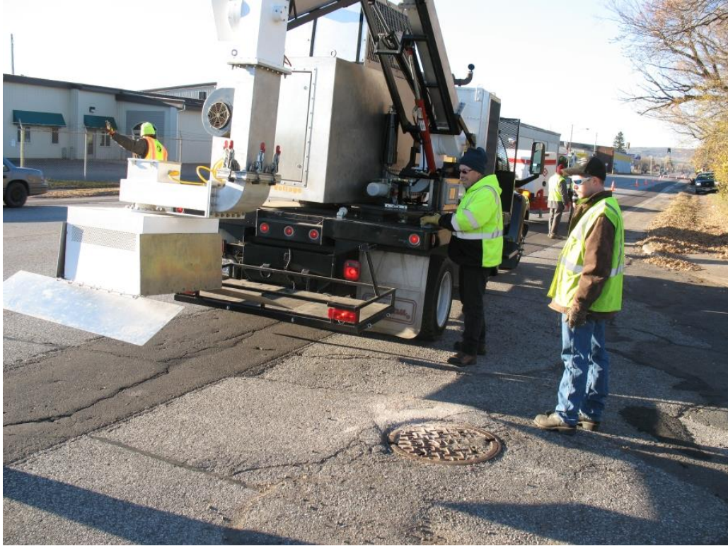
Figure 3.39. Preparing microwave for manhole repair test: 64th Avenue West and Grand Avenue.
