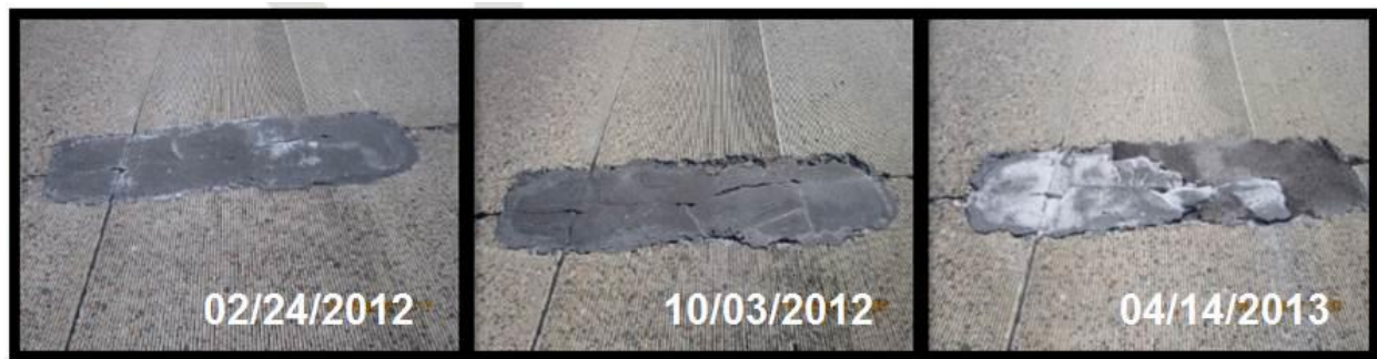
Figure 3.76. Photo sequence of Rapid Patch repairs, MnROAD I-94 mainline Cell 9, Joint 162 location: 2/24/2012 to 4/14/2013 (Johnson, 2014).
