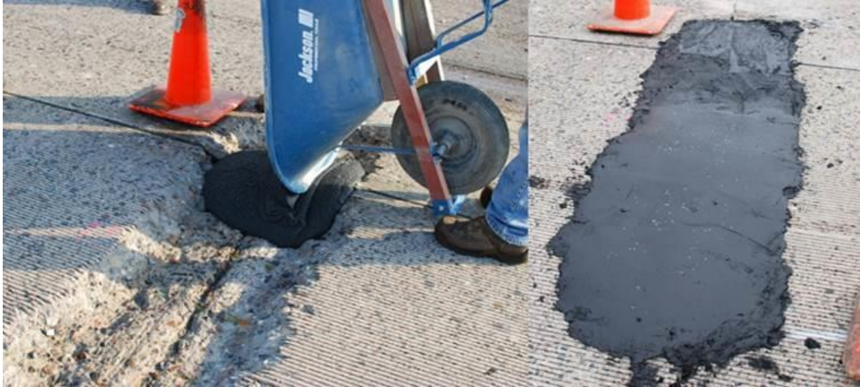
Figure 3.74. Rapid Patch installation on MnROAD I-94 mainline: Joint location 162, September 1, 2011.
