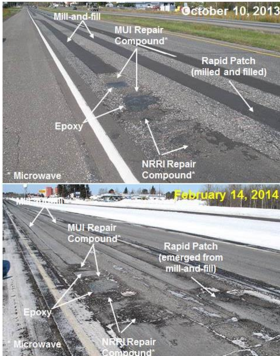
Figure 3.33. Condition of Highway 53 (Monaco Air sign) location repairs: October 10, 2013 and February 14, 2014.
