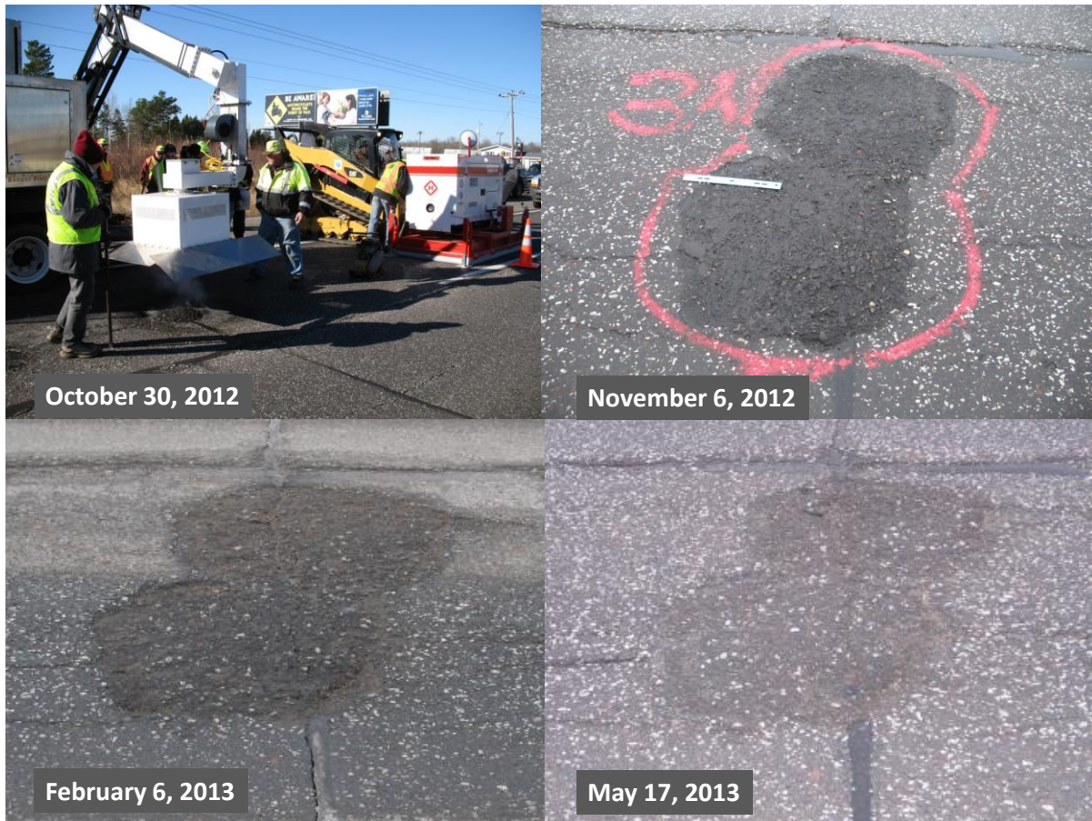
Figure 3.18. Highway 53 microwave pothole (Hole 3) repair; note the 12 inch ruler for scale in the November 6 photo.
