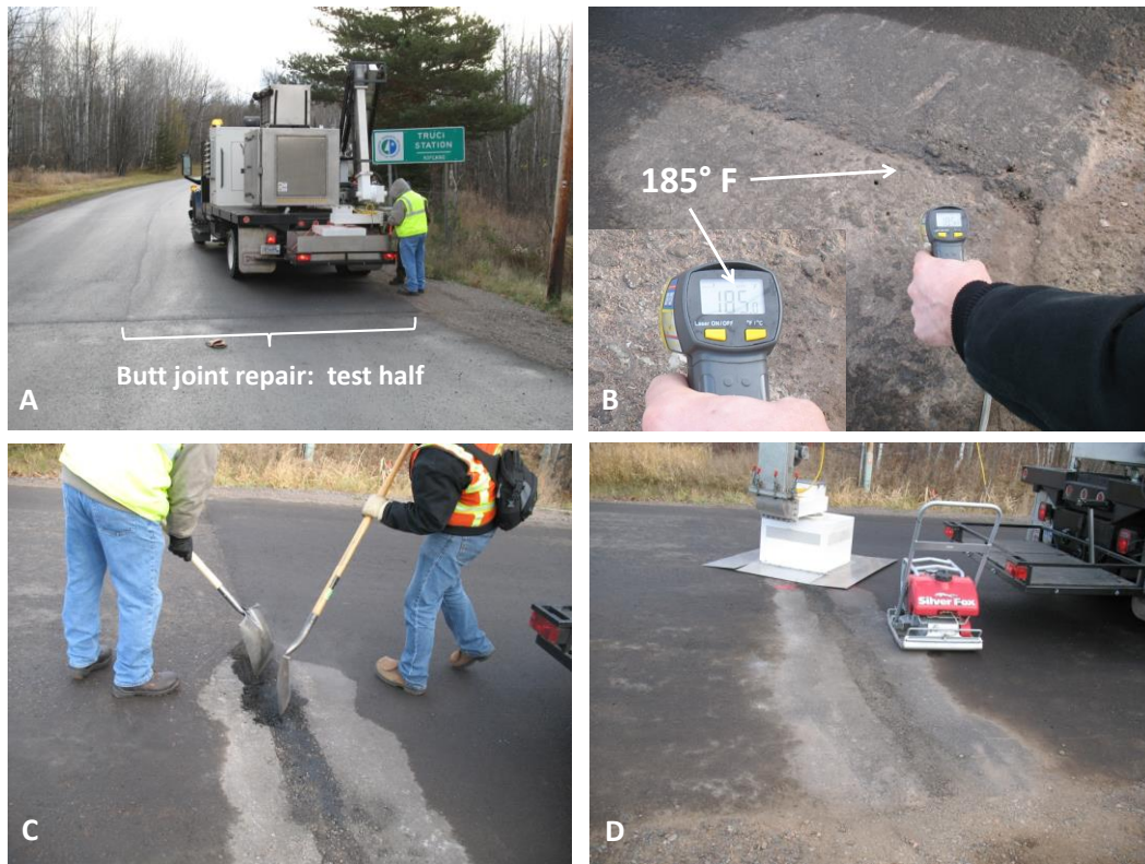
Figure 3.56. Microwave butt joint repair test, Nopeming Truck Station entrance, November 1, 2012.
