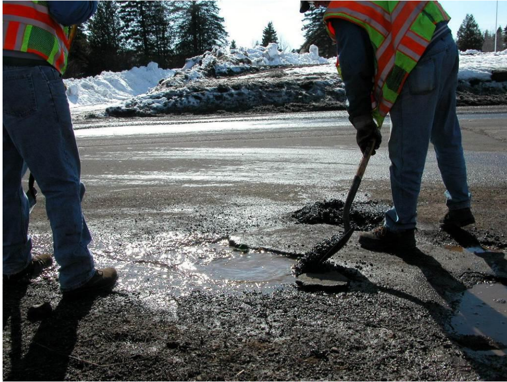
Figure 2.1. “Throw and go” method of pothole repair.
