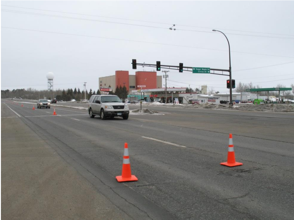
Figure 3.22. Location of first March 1, 2013, Rapid Patch repair; Highway 53, Duluth (NRRI building in background).
