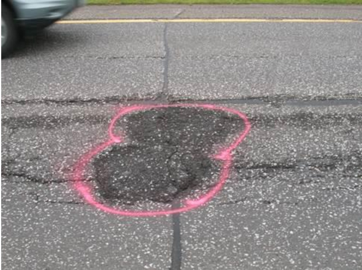
Figure 3.19. Highway 53 microwave pothole (Hole 3) repair condition on July 30, 2013.
