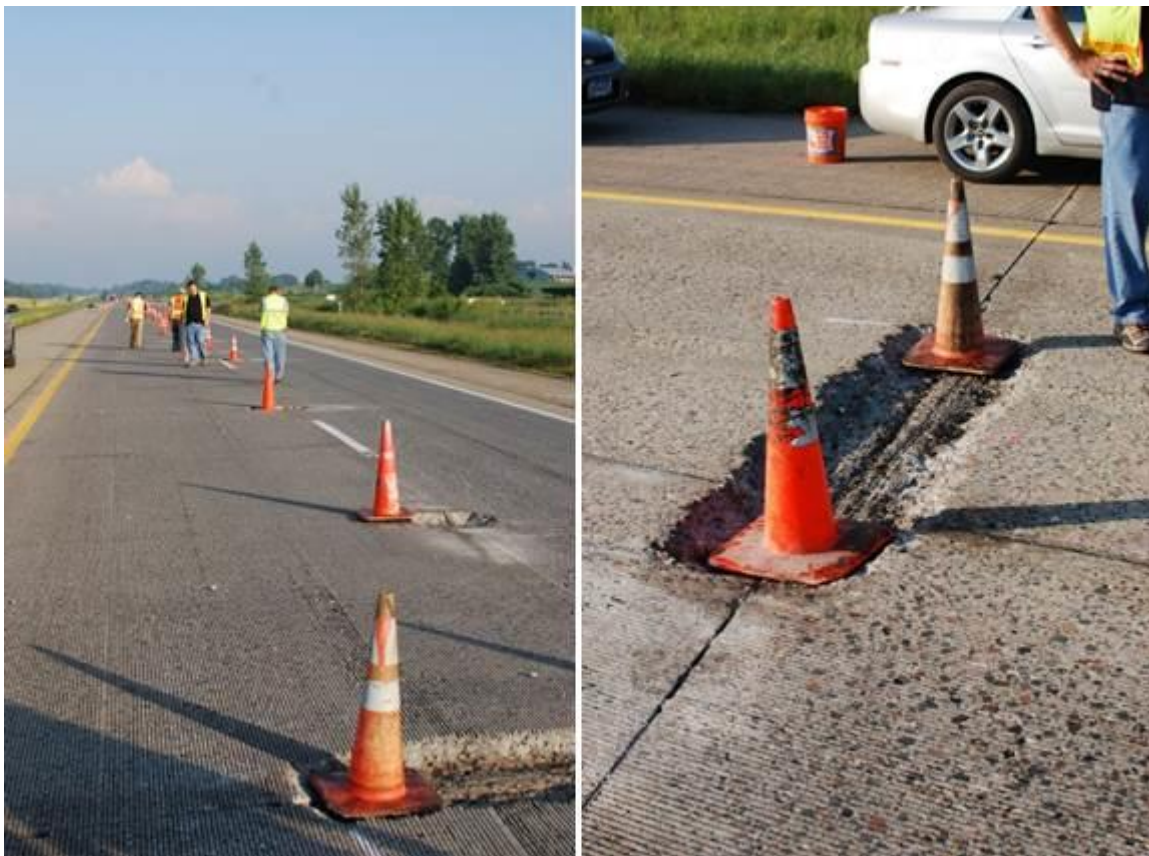
Figure 3.73. Rapid Patch repair location on MnROAD I-94 mainline: Joint location 162, September 1, 2010.
