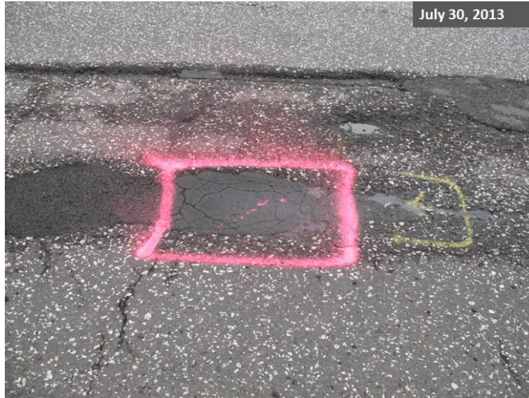
Figure 3.26. Condition of Hwy 53/Cirrus Drive Rapid Patch repair on July 30, 2013.
