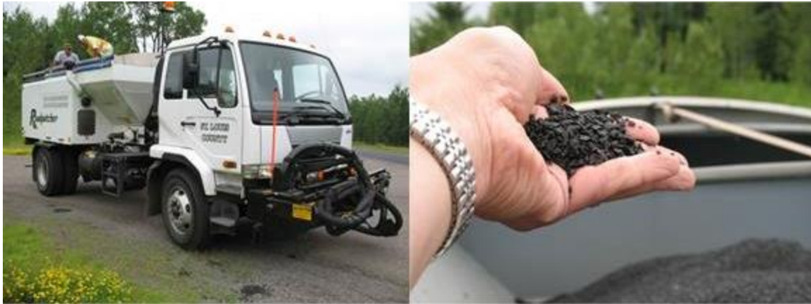
Figure 2.2. Spray patch vehicle (left) and coated aggregate used for patching (right).
