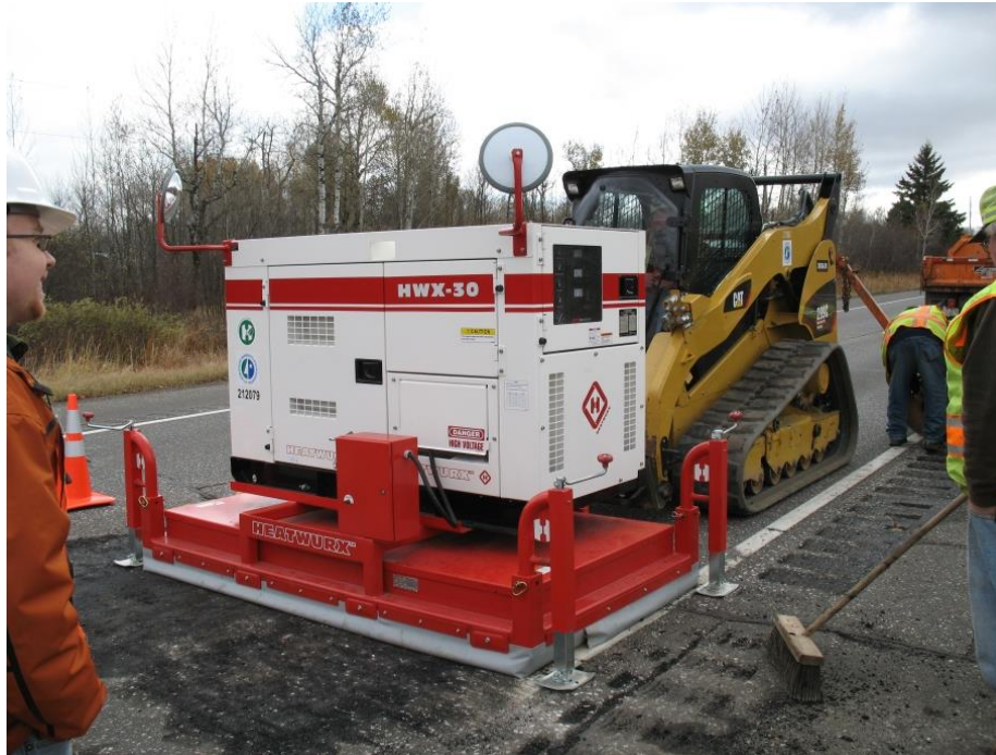
Figure 3.2. HeatWurx unit and skid-steer.
