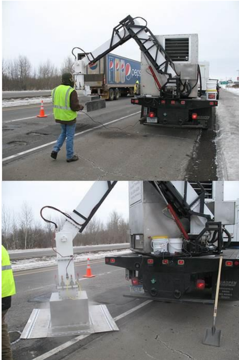
Figure 3.29. Positioning microwave unit (upper photo) and microwave heating (lower photo), Highway 53 Monaco Air sign location: March 1, 2013.
