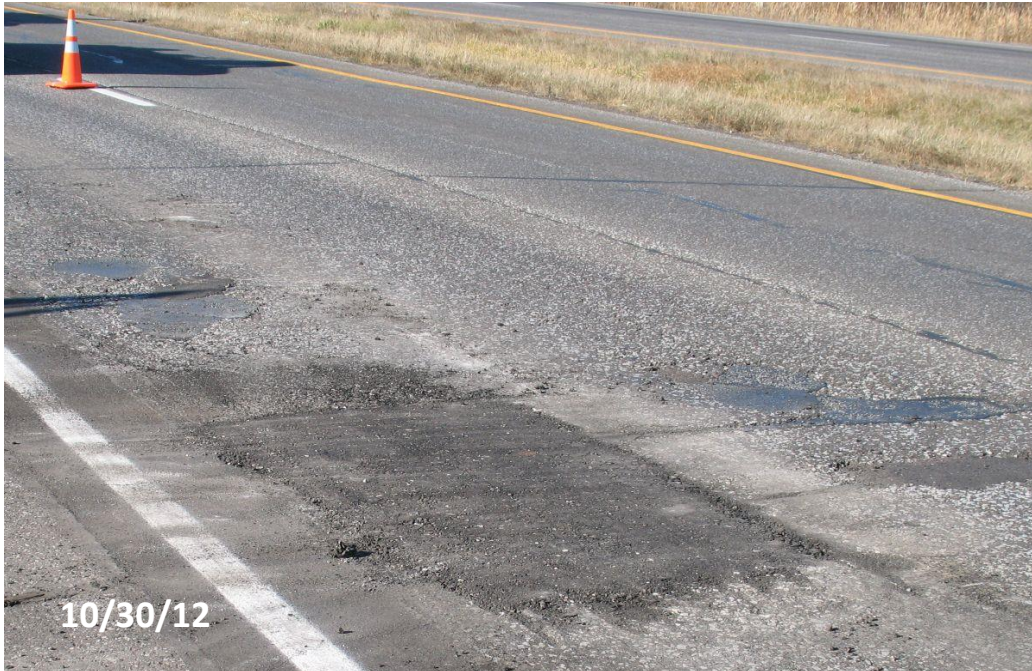
Figure 3.16. HeatWurx repair #2, Highway 53 (Monaco Air sign) location, October 30, 2012.
