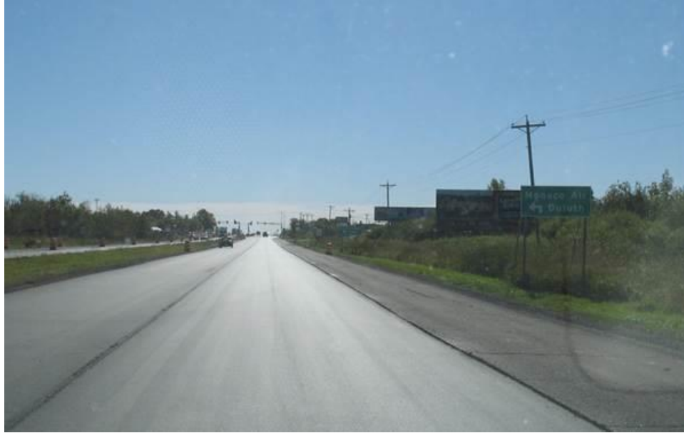
Figure 3.37. New mill-and-overlay of Highway 53 at Monaco Air sign field trial location: September 29, 2015.
