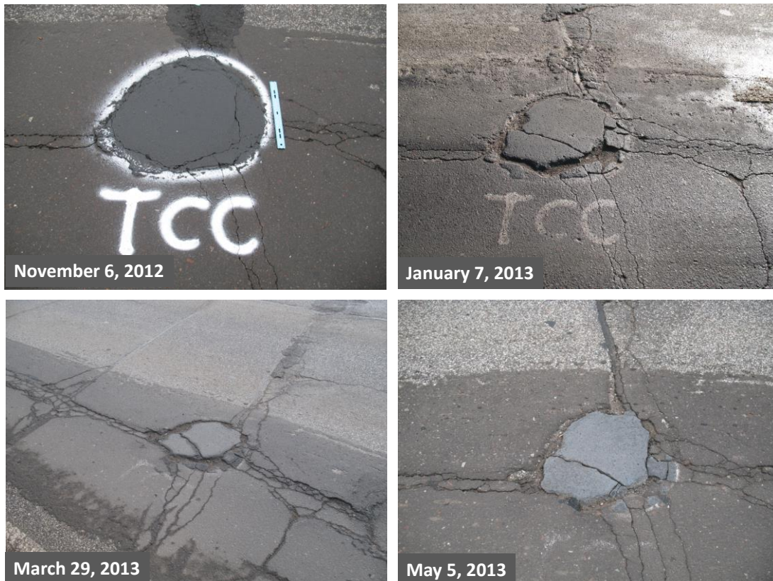
Figure 3.52. Rapid Patch repair condition through May 5, 2013; Grand Avenue wheel path.
