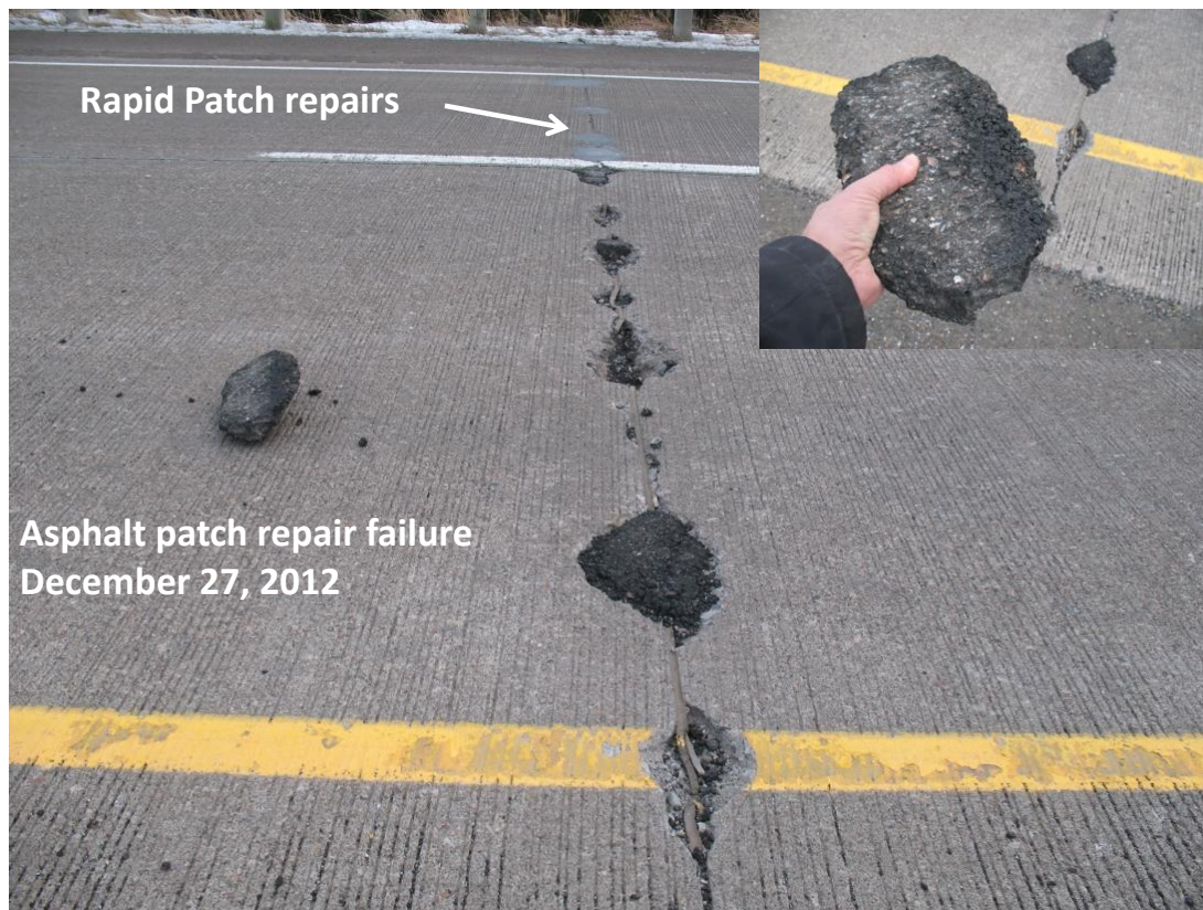
Figure 3.66. Highway 61 expressway asphalt patch repair failure: December 27, 2012.
