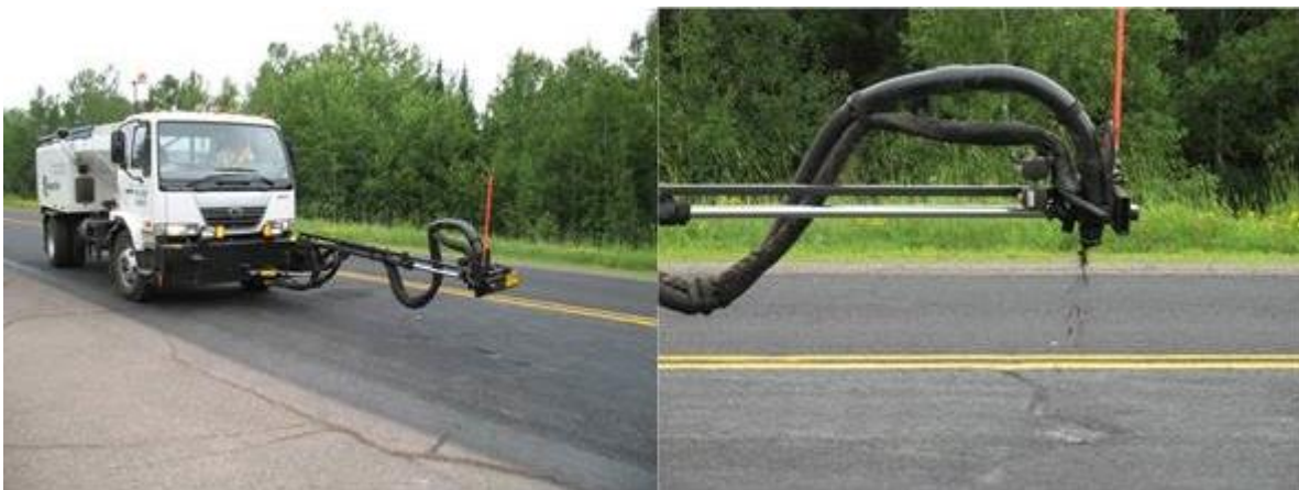
Figure 2.3. Spray patch vehicle deployed (left); close-up of spray nozzle and patching (right).
