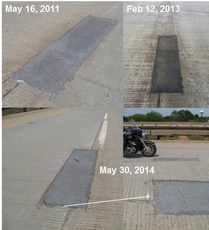
Figure 3.71. Photos showing condition of Highway 169 Keewatin bridge deck repair from May 16, 2011 through May 30, 2014.
