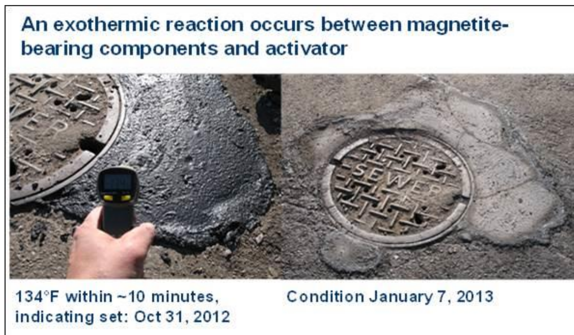
Figure 3.41. Rapid Patch manhole repair: initial set, and condition on January 7, 2013.
