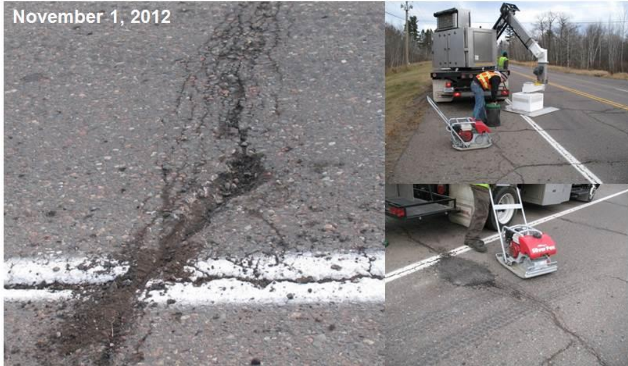
Figure 3.62. Becks Road/Midway Road pothole (left) and microwave repair (right): November 1, 2012.
