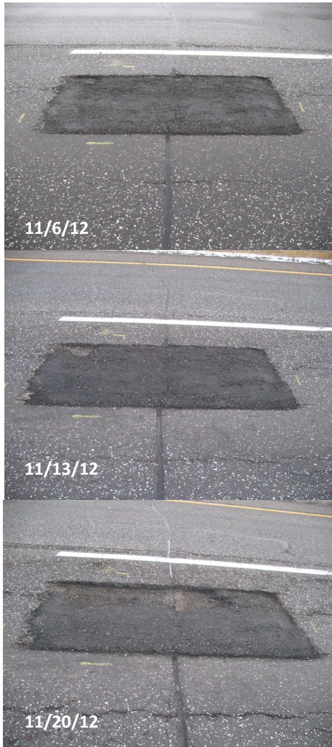
Figure 3.15. HeatWurx repair #1 (Bullyan location), showing progressive loss of material.
