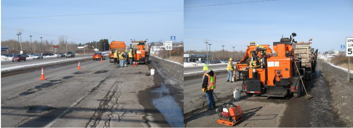
Figure 3.11. Stepp repairs Highway 53, Feb. 26, 2013. Note pre-heating of repair with torch (right photo).
