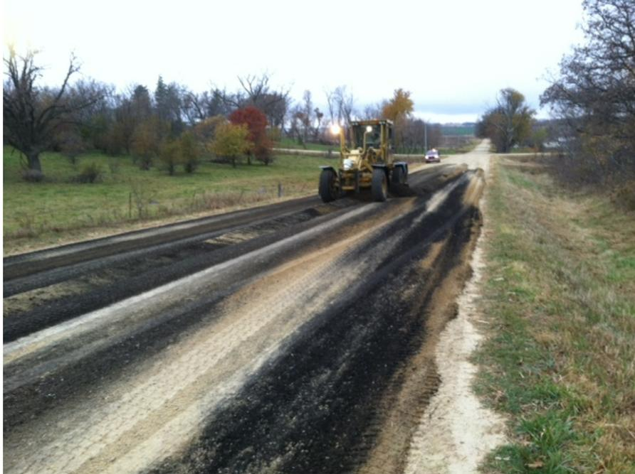
**Figure 6 Goodhue CR 6 placing shingles on CI 6 limestone**
