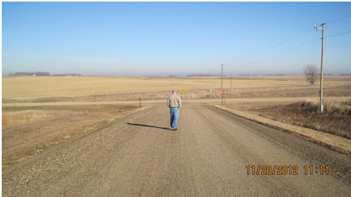
**Figure 4 Jackson Co. Looking toward CR 81 on 750th Str. 1 part shingle to 1 part gravel blend**
