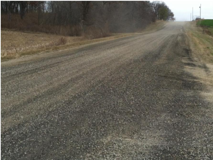
**Figure 7 Goodhue CR 52 Finished blend of TOSS and CI. 6**
