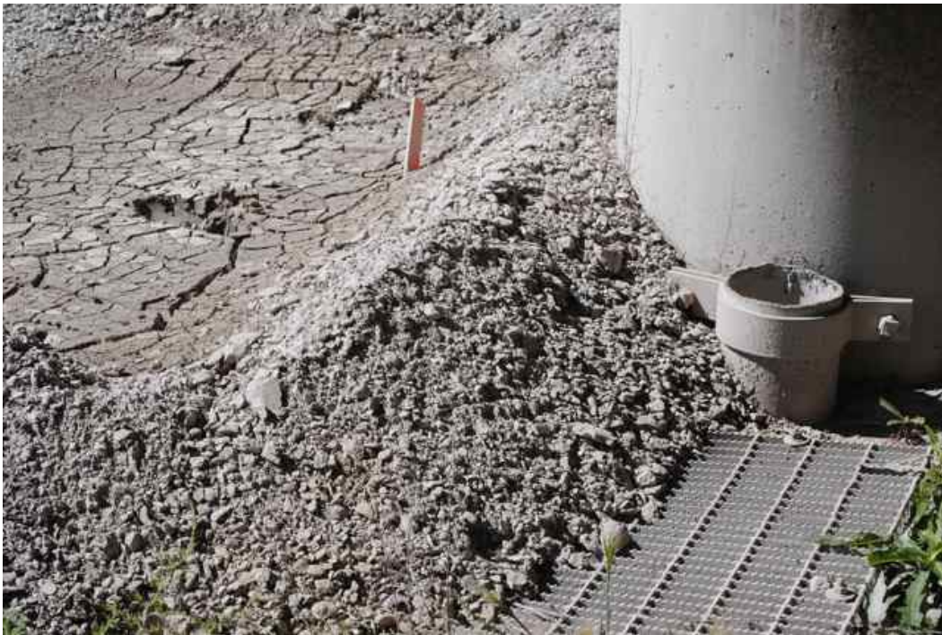
Figure 11: Concrete pavement grinding sediment dropped from elevated highway and formed into basin shape in location adjacent to scupper drain and catch basin.
