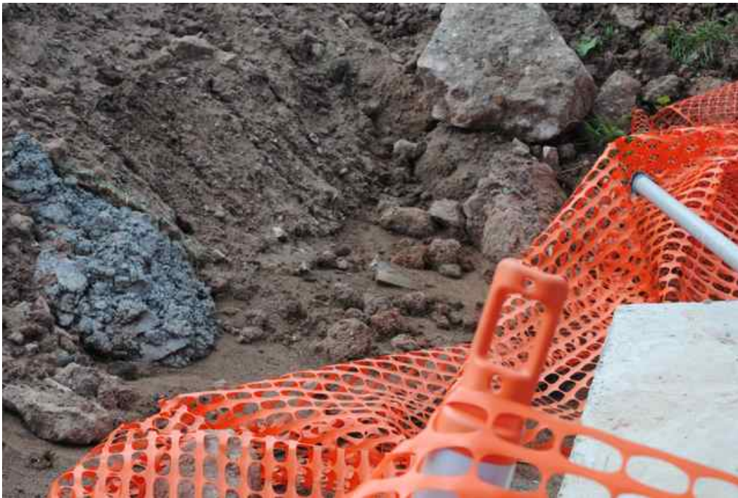
Figure 3: Concrete debris left on ground surface adjacent to high mast light pole foundation.
