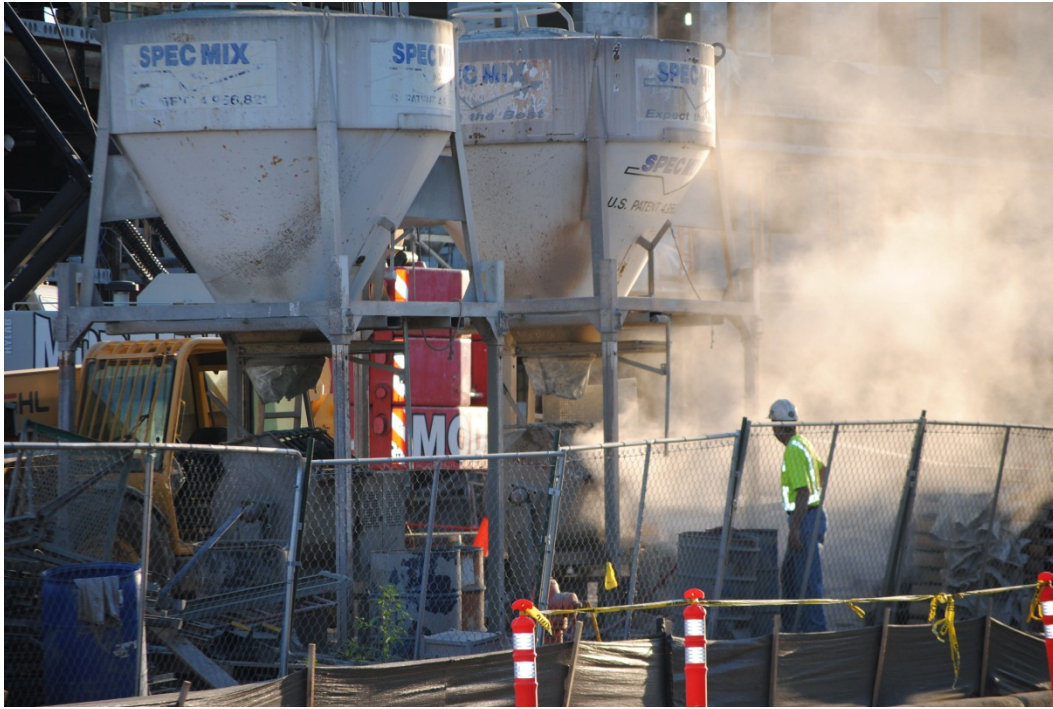
Figure 2: Dust cloud emerging during use of metering of cement for mortar mixing.
