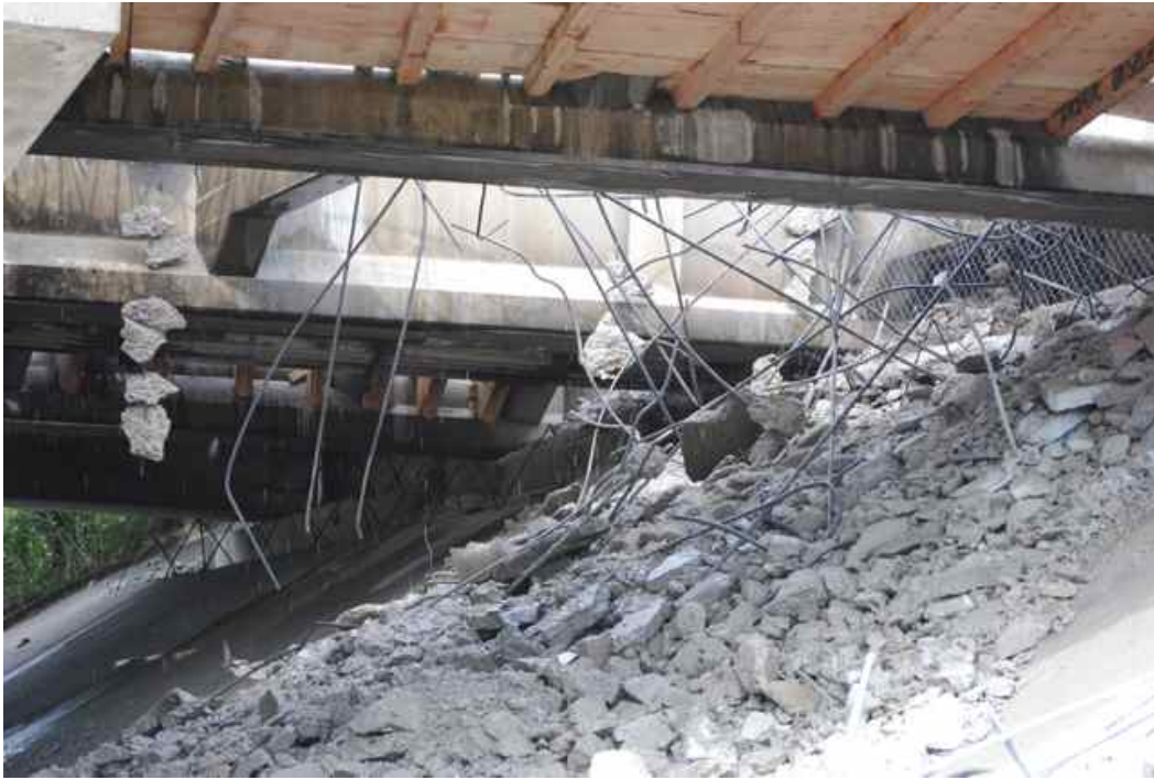
Figure 4: Debris dropped from deck breaking operations.
