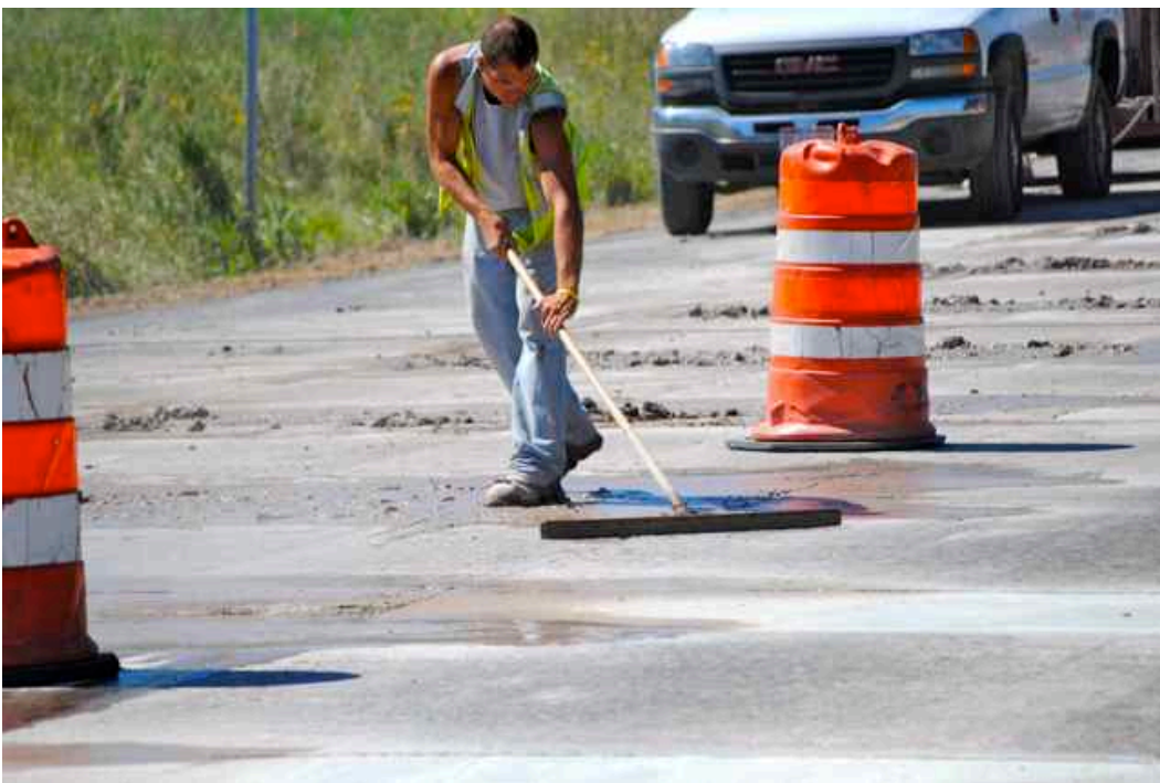
Figure 3: Saw cut debris management by screed prior to collection.
