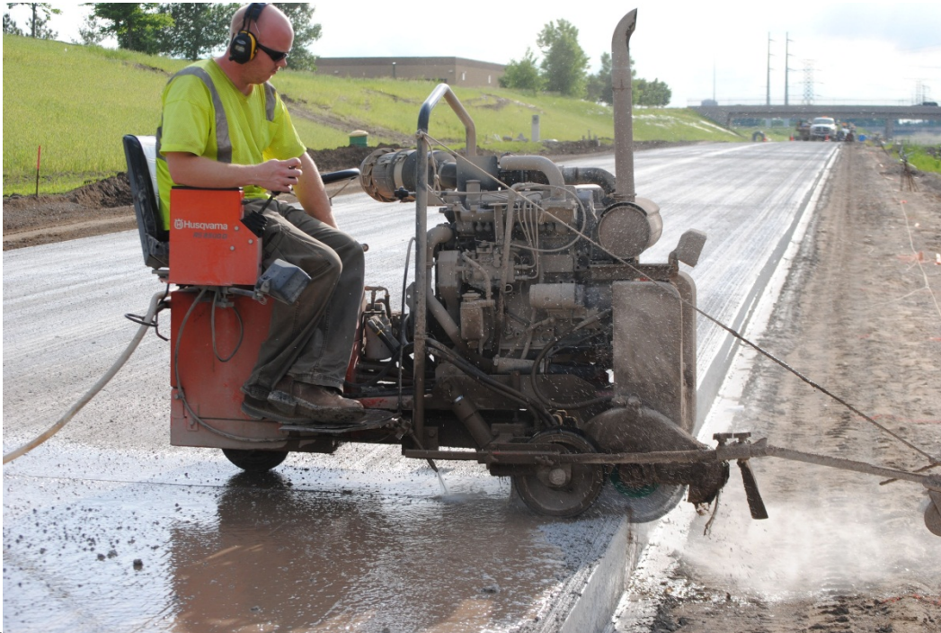
Figure 1: Wet sawing of green concrete.
