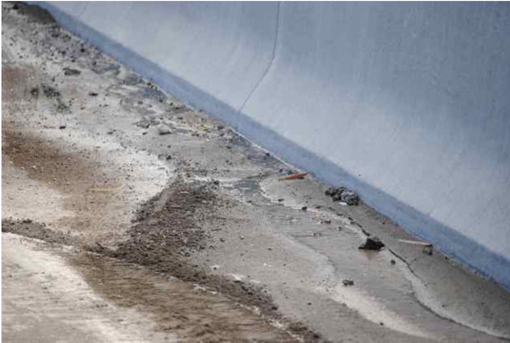
Figure 4: Sediment and incompletely filtered water released from bermed sediment filter sump in roadway gutter approximately 50 feet down slope.
