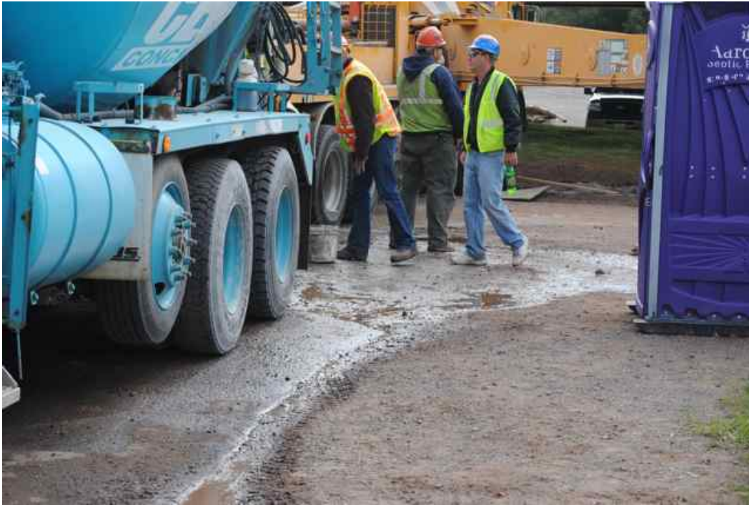
Figure 4: Water and sediment on grade adjacent to ready mix truck and concrete pump.
