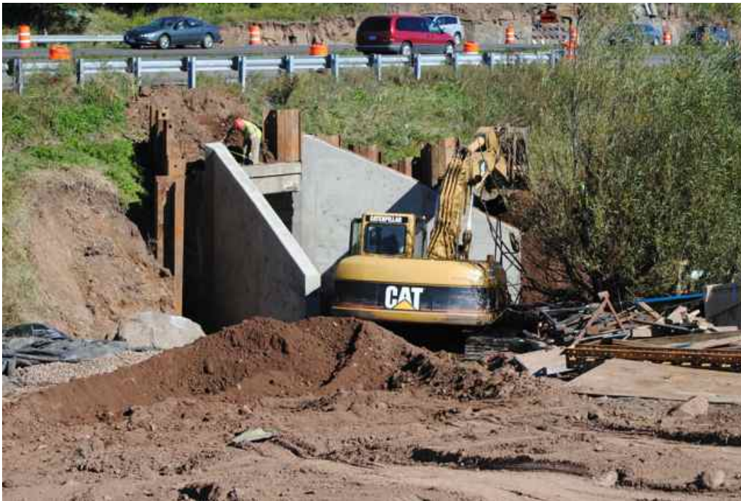
Figure 1: Concrete wing wall form removal after concrete curing and initial backfill casting.
