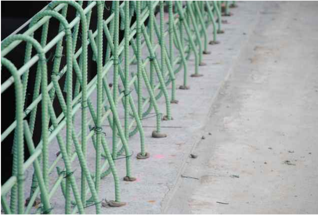
Figure 2: Parapet reinforcement epoxied into drill holes adjacent to recently ground pavement.
