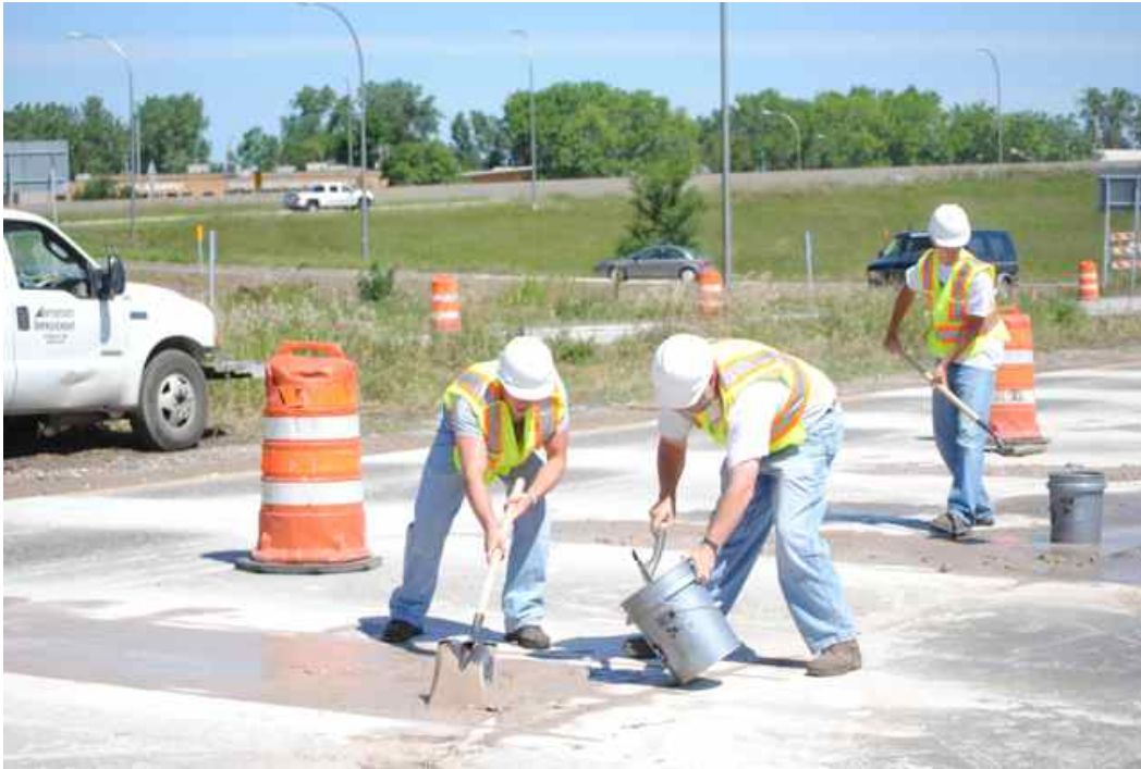
Figure 4: Saw cut debris sampling. Note open shoulder of roadway towards ramp gore.
