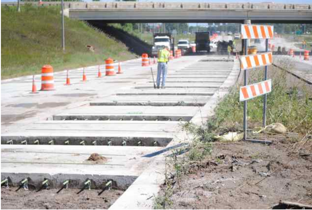
Figure 8: Repair sections prepared for rapid set concrete placement. Note disturbed median, set apart from roadway by existing curb.
