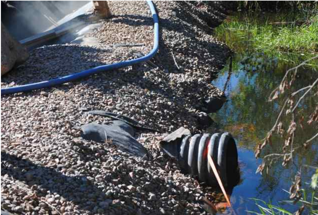
Figure 2: Lined stone berm cofferdam with corrugated HDPE bypass pipe inlet, upstream of culvert.
