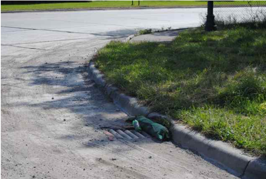
Figure 8: Concrete pavement grinding sediment bypassing catch basin following gutter line onto local street (bottom of ramp shown in Figures 4 and 6).
