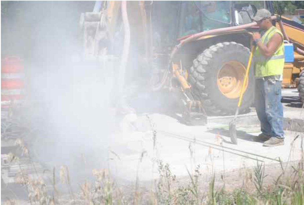
Figure 6: Drilling holes for inter-slab dowels using backhoe mounted air percussion drill, with fugitive dust and concrete sediment.
