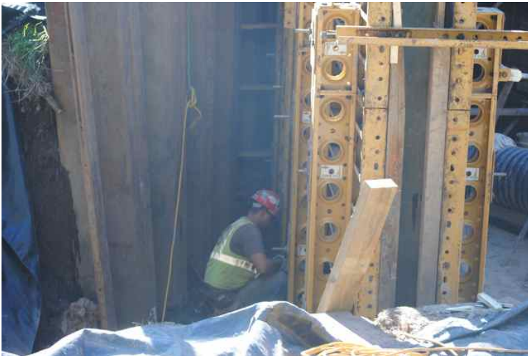
Figure 7: Wing wall formwork with end cap removed showing recently placed concrete.
