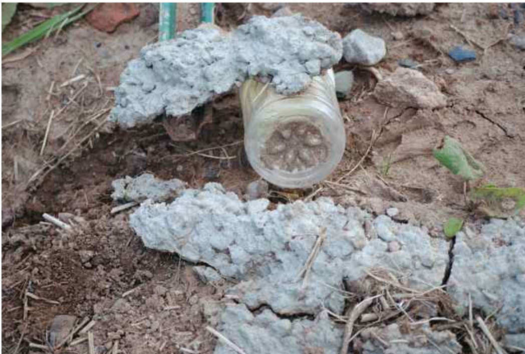
Figure 5: Concrete debris left on ground surface adjacent to high mast light pole foundation.
