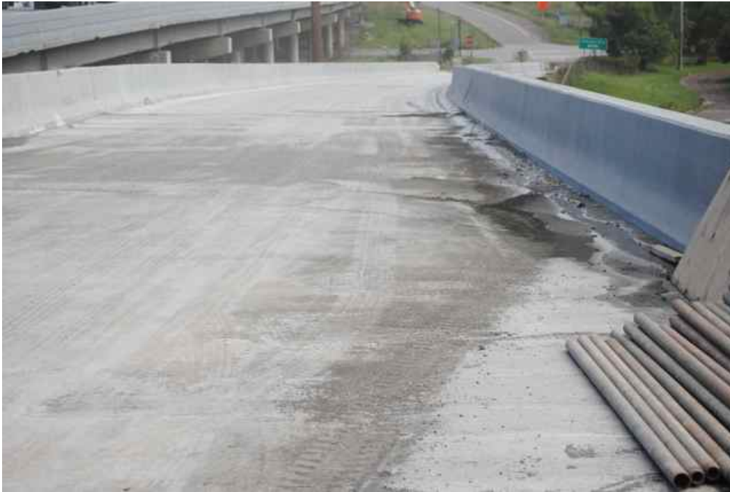
Figure 4: Concrete pavement grinding sediments remaining after incomplete sweeping effort (note: water in gutter is due to concrete washout activities).
