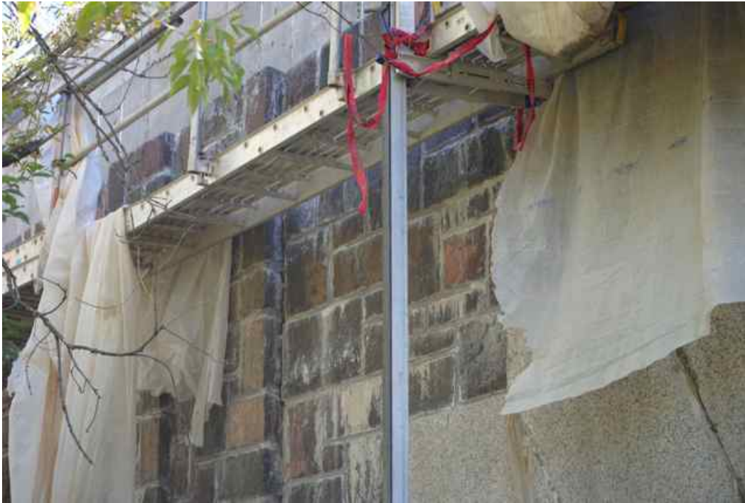
Figure 2: Chemical and debris catch system with discontinuities, view from below.
