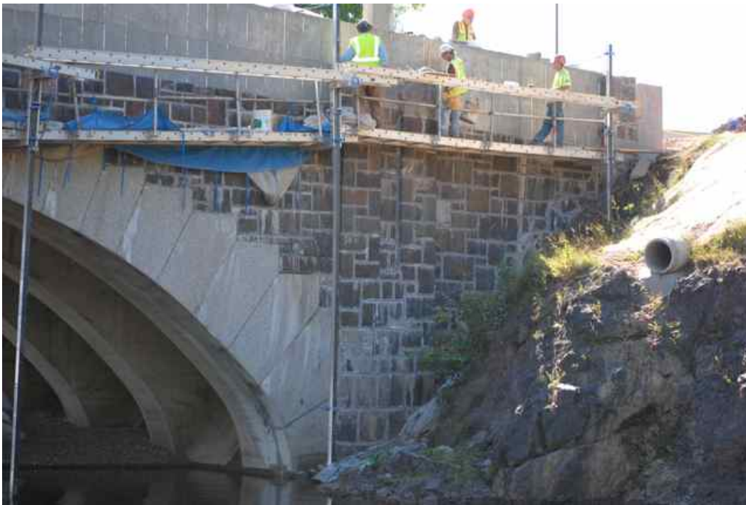
Figure 1: Masonry facing and parapet repairs being made from scaffolding, with chemical and debris catch system made of plastic sheeting on both the ground next to the abutment wing wall and on the scaffolding.
