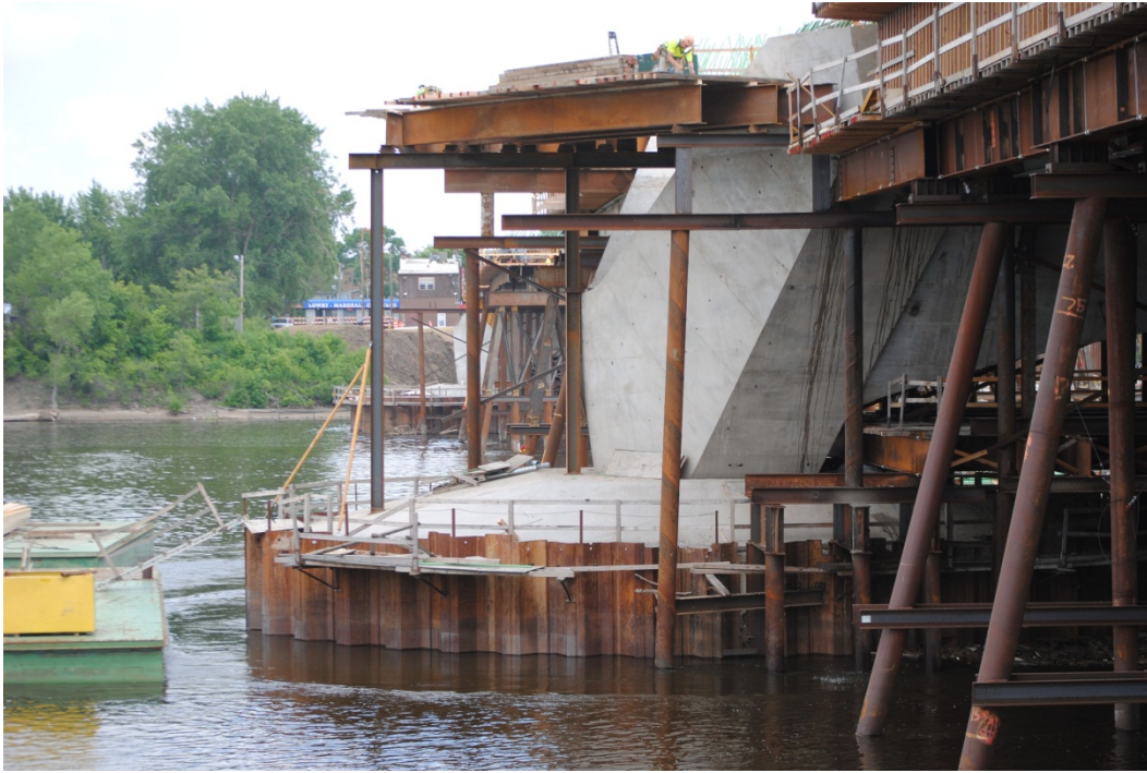
Figure 4: Sheet pilings in the river were used to create cofferdam that separates the river flows from the concrete pour. Note pile supported form work that also provides debris containment related to the bridge pier cap, beams and deck construction.
