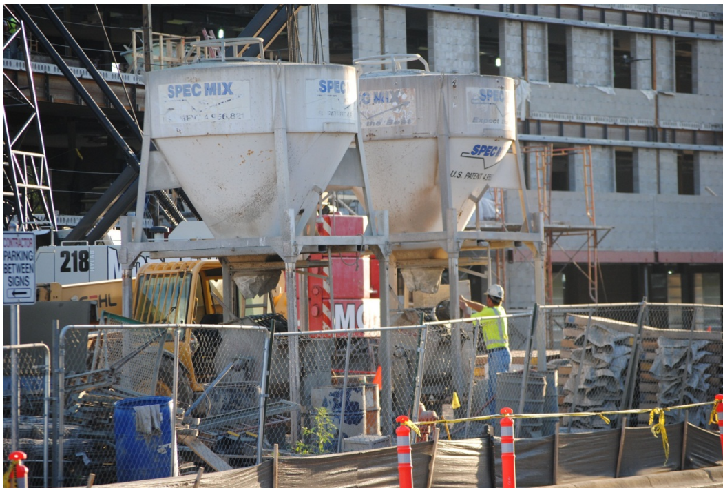
Figure 1: Super sack silo system and batch mortar mixers.
