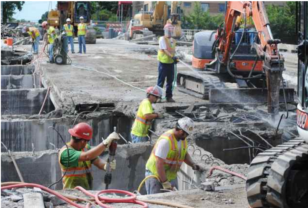
Figure 1: Removal of concrete deck by hand operated air hammers and equipment mounted hoe-ram, with water application for dust control.
