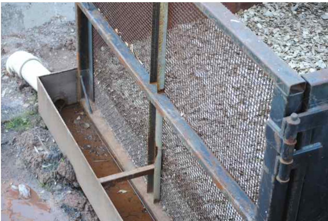
Figure 5: Filter compartment 4 with wood chip filter media, end screen, effluent trough and outlet pipe. Note trace of organic sediments in trough but no build up around outlet.
