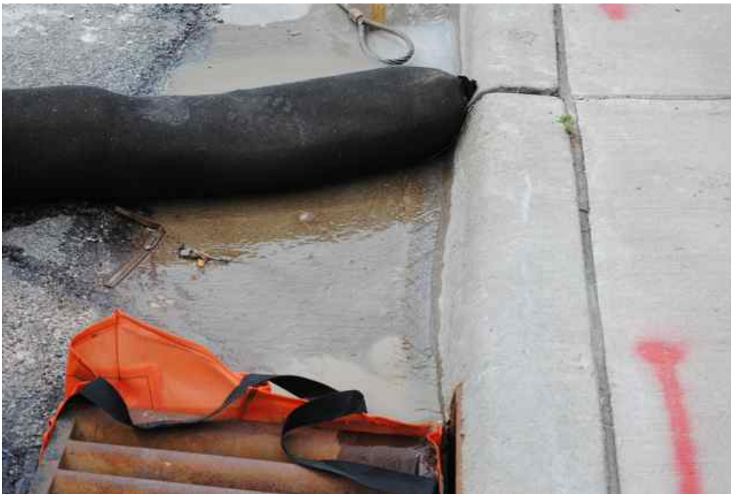
Figure 7: Filtration log and woven geotextile catch basin liner (Dandy Bag) placed in combination along gutter line of Lasalle Avenue. Note clarification of flow by filtration log with small amount of sediments trapped before the catch basin.
