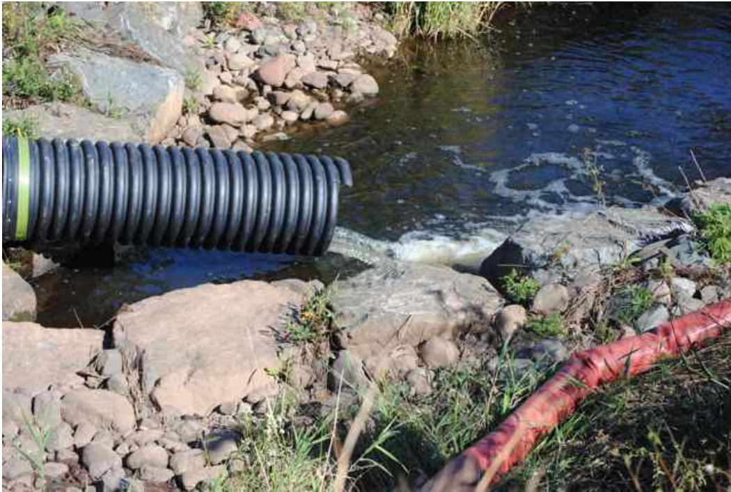
Figure 4: Bypass pipe discharge to streambed over downstream cofferdam.
