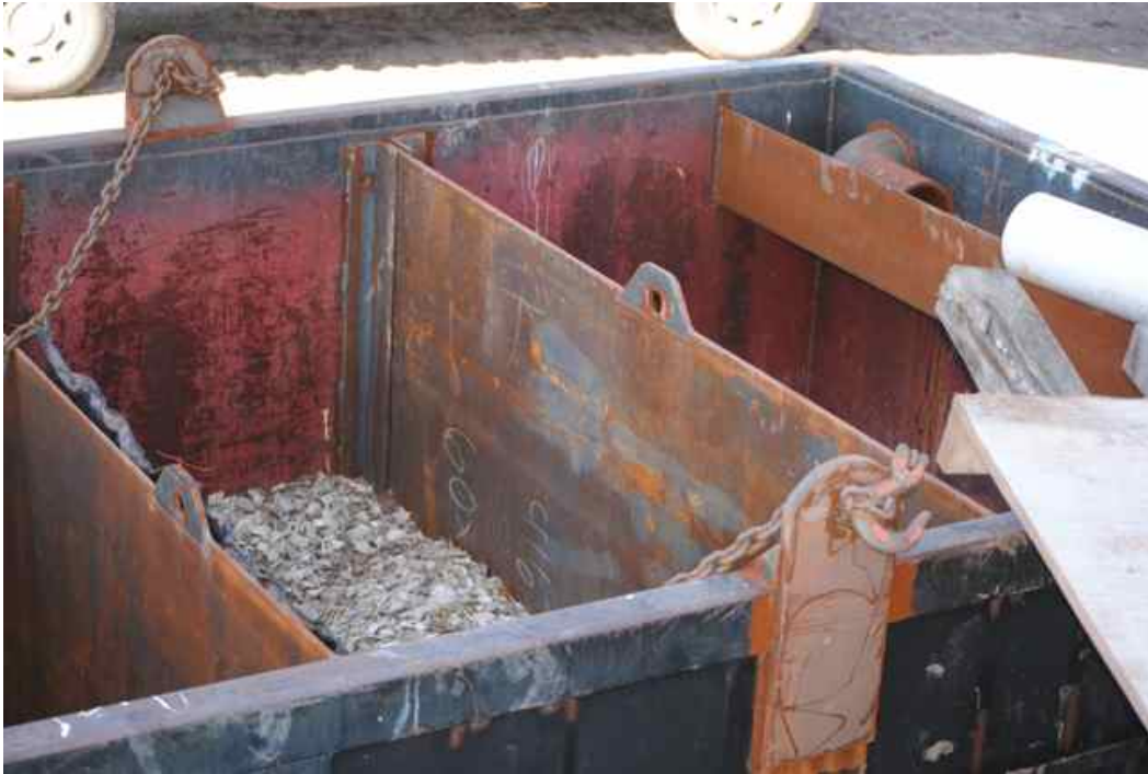
Figure 4: Filter box, compartments 1 and 2, showing wood chip filter media in compartment, inlet pipe and emergency overflow bypass weir, trough and outlet.
