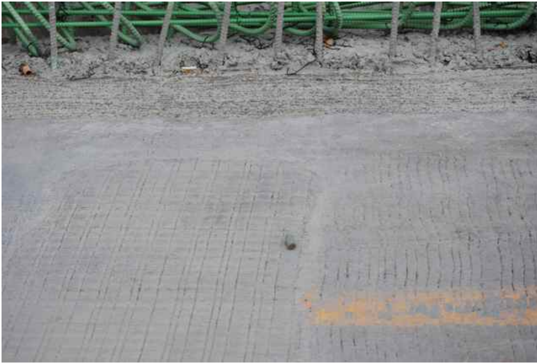
Figure 1: Elevated highway pavement profiled by grinding (grooving) adjacent to bridge parapet (yet to be poured), showing residual fines after sweeping.
