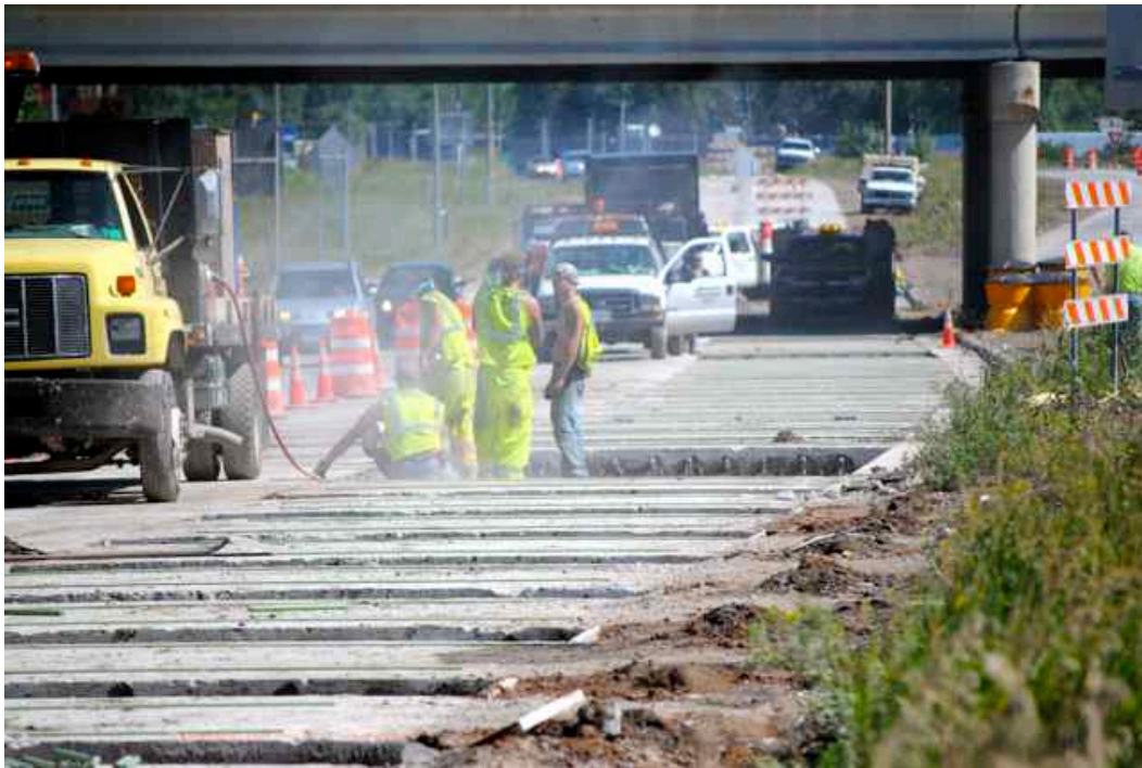
Figure 5: Epoxy and dowel installation in drill holes.
