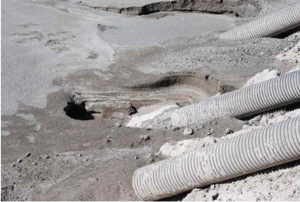
Figure 2: Concrete pavement grinding sediment disposal lagoon influent pipe discharge, adjacent to truck dump station.
