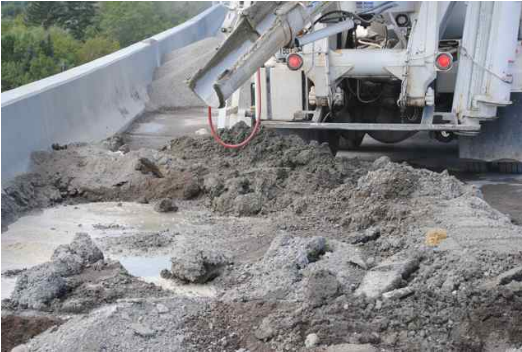
Figure 2: Liquid pool within bermed sediment filter sump, at or near capacity.
