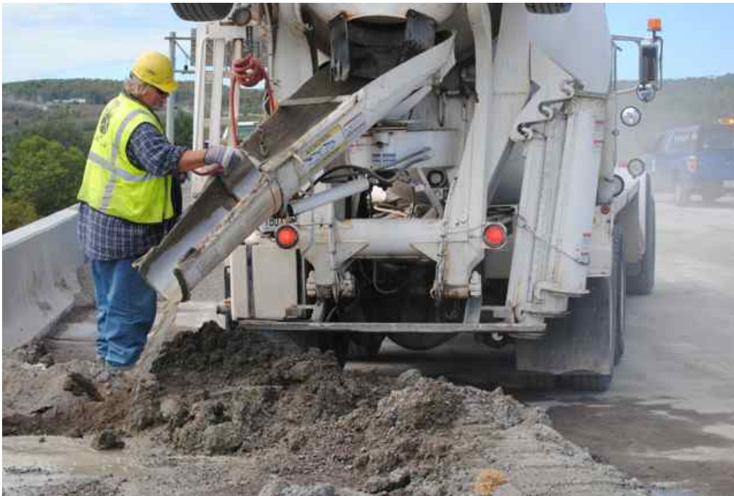
Figure 1: Washout of ready mix truck on elevated highway into bermed sediment filter sump.
