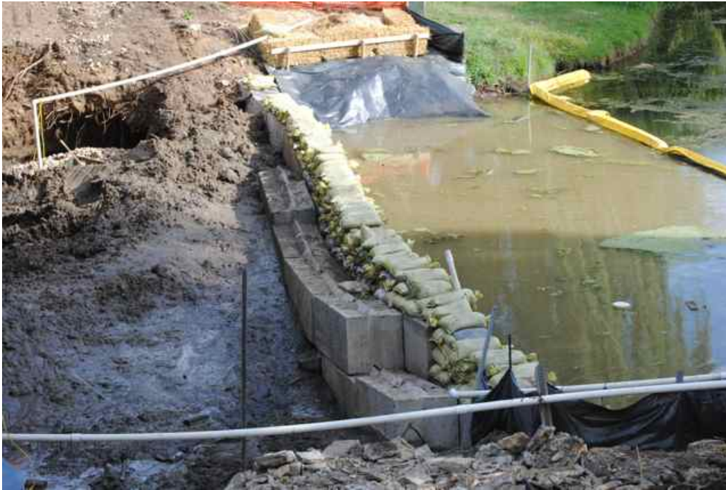
Figure 2: Silt curtain, concrete block and liner cofferdam, dewatering pump pit and dewatering discharge filter.
