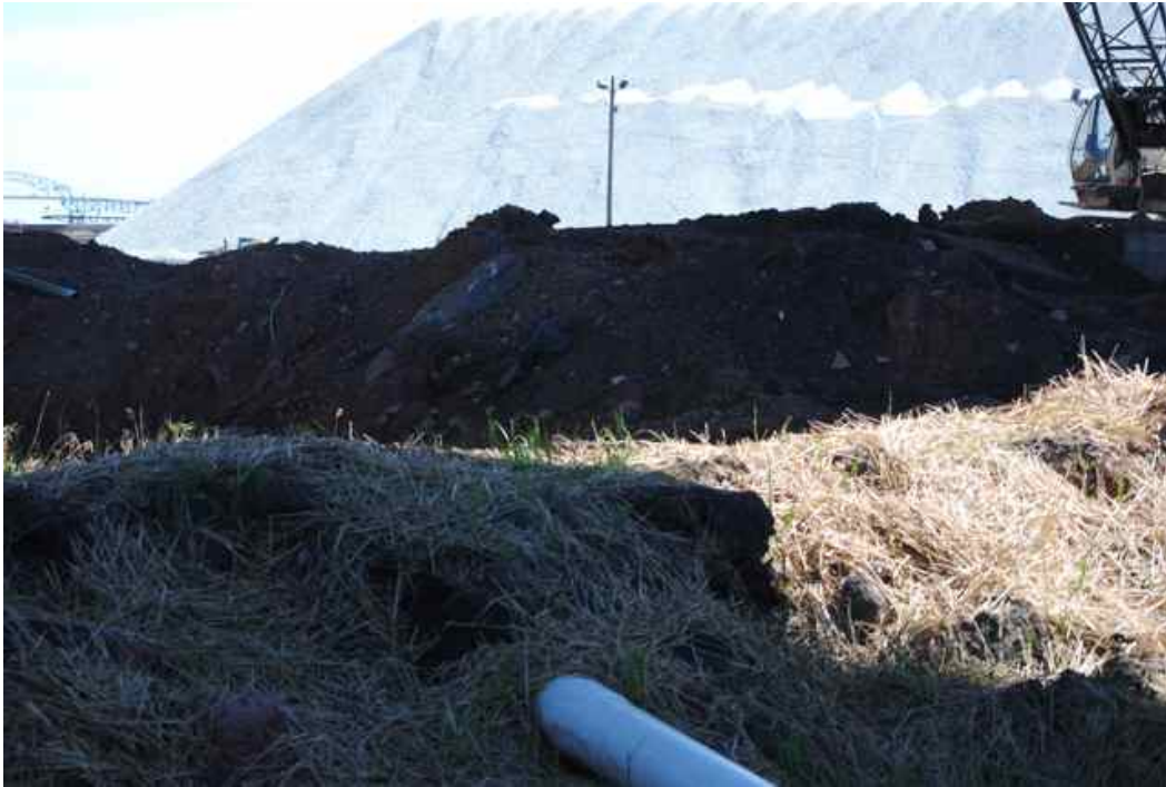
Figure 2: Sediment pond dike, mulched, with outlet pipe.
