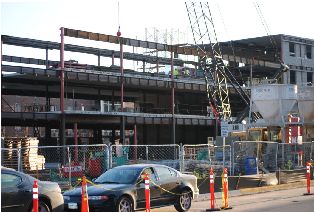
Figure 3: Super sack mortar station location in relationship to street. Note dust accumulating on vehicles.
