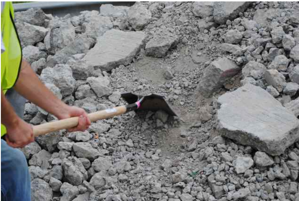
Figure 3: Debris pile, ready for load out. Note mixture of fines with coarse particles and slab chunks.
