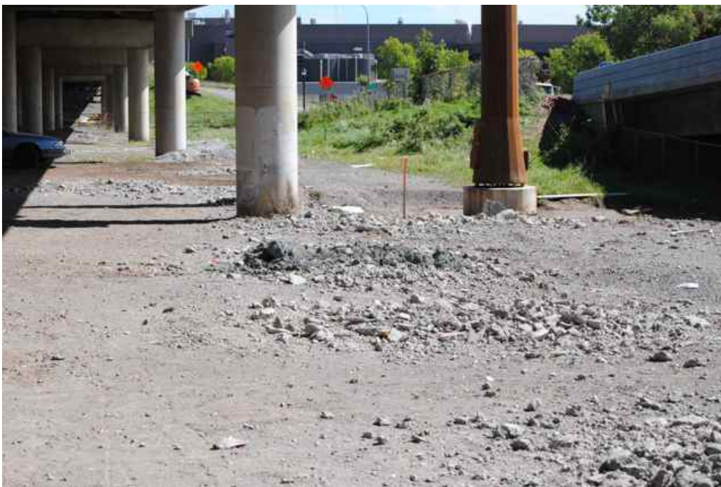
Figure 9: Concrete debris and fugitive pavement grinding sediment below elevated highway (below location of Figure 4), dropped to ground surface with no stormwater controls (perhaps awaiting follow up excavation).
