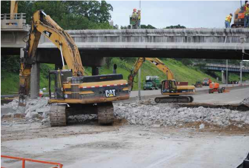
Figure 2: Excavator-mounted jaws performing concrete crushing to allow for reinforcing bar removal prior to load out. Note sand protective layer below concrete rubble.
