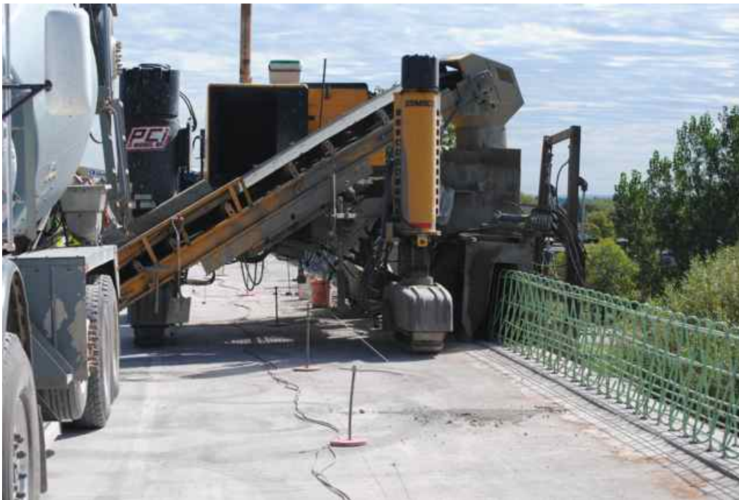
Figure 1: Parapet wall pour with traveling form machine and delivery of concrete by ready mix truck.
