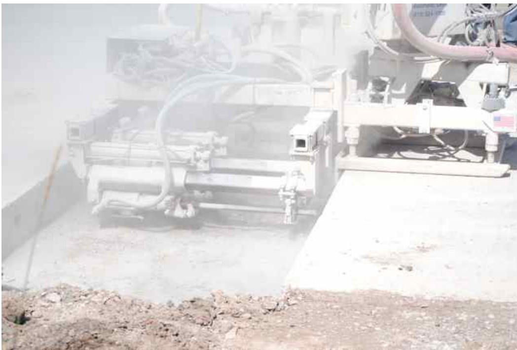
Figure 7: Air percussion drill in operation.
