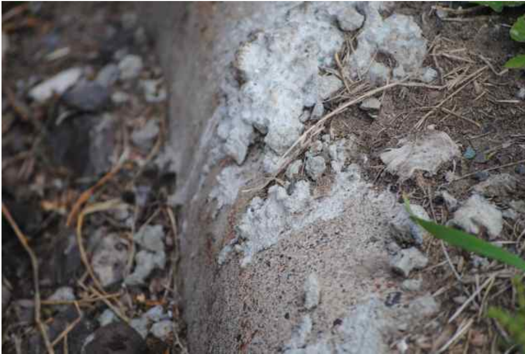
Figure 4: Concrete debris left on curb adjacent to high mast light pole foundation.
