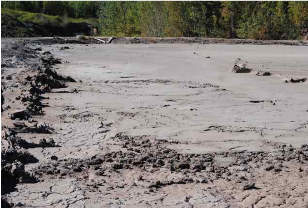
Figure 4: Second concrete pavement grinding sediment disposal lagoon.
