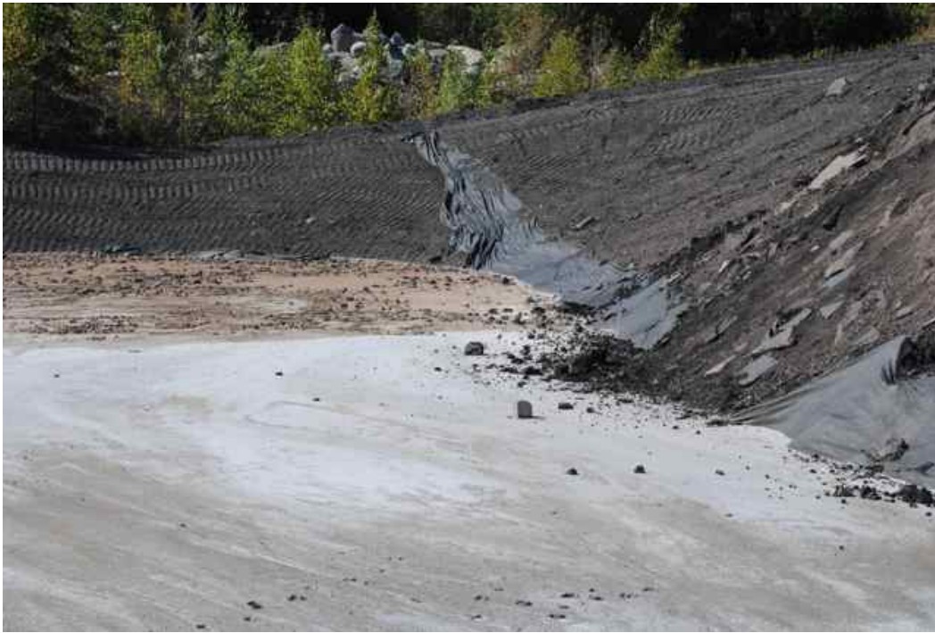
Figure 1: Concrete pavement grinding sediment disposal lagoon with current estimated depth of 10 to 15 feet.
