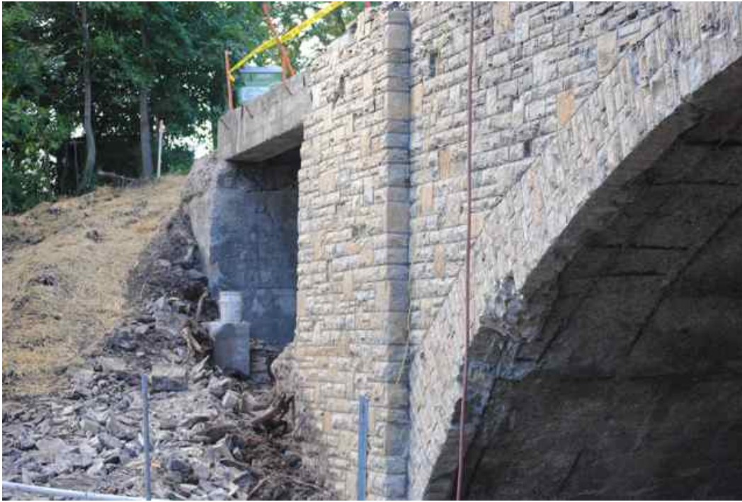
Figure 4: Wing wall and arch fascia masonry prior to repair grouting and repointing with localized removal for abutment repairs.
