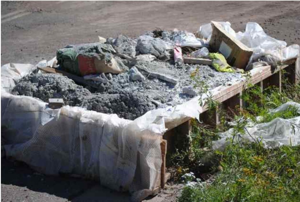
Figure 4: Accumulation and on-site storage of concrete and mortar debris plus solid waste.
