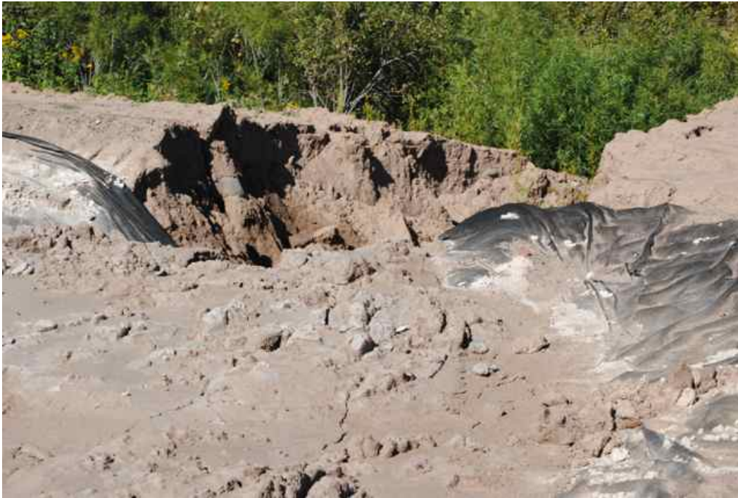
Figure 6: Containment dike failure, second concrete pavement grinding sediment disposal lagoon.
