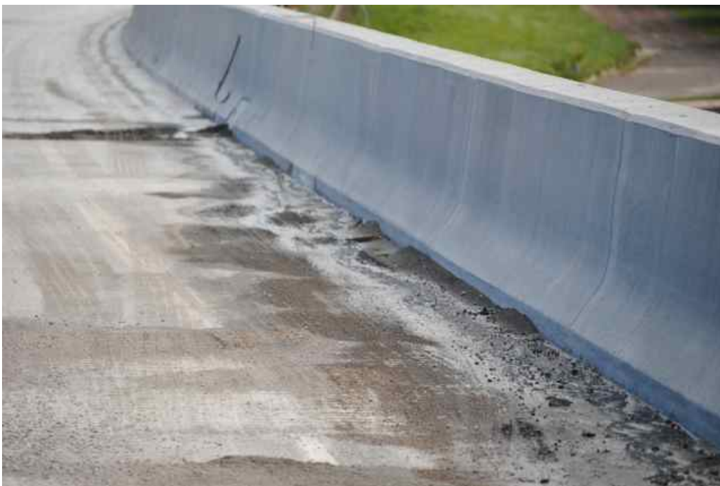
Figure 3: Sediment and incompletely filtered water released from bermed sediment filter sump in roadway gutter approximately 25 feet down slope.
