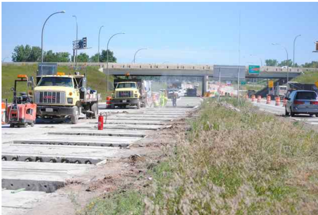
Figure 1: Concrete pavement repairs consisting of saw cutting, removal of damaged concrete, preparation of base, dowel connection to adjacent pavement slabs and replacement of pavement with quick set concrete.
