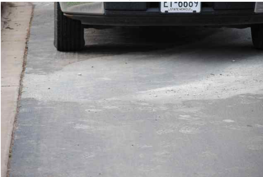
Figure 5: Cement sediment draining to pavement approximately 50 feet from concrete pump.
