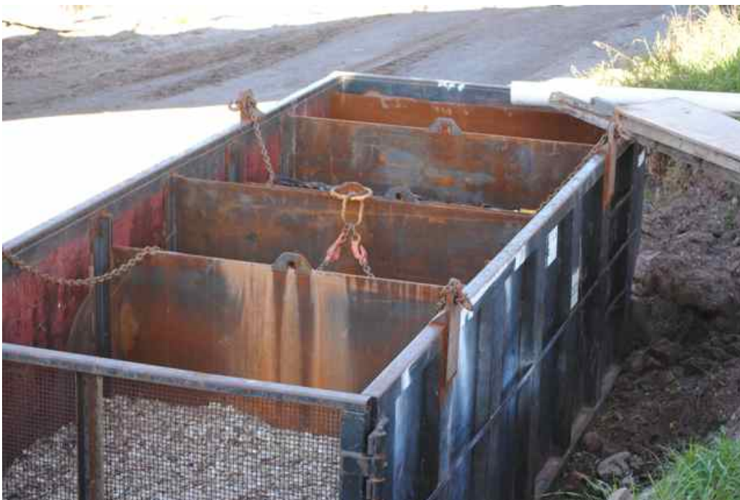
Figure 3: Sediment pond outlet pipe and four zone filter comprised of wood chips and vertical steel sheet baffles, set for underflow, in a roll off box.
