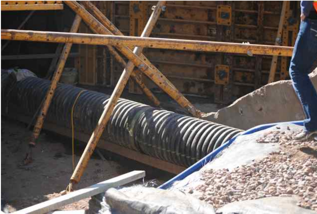
Figure 6: Upstream wing wall formwork and bracing, placed around bypass pipe and cofferdam.
