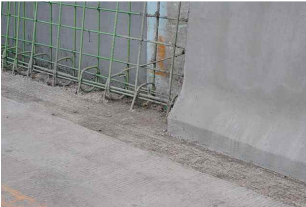
Figure 3: Concrete pavement after profile grinding, adjacent to bridge parapet being reconstructed.
