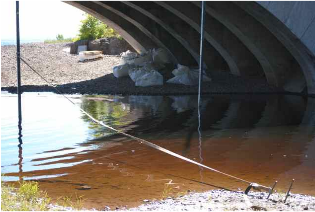
Figure 6: Chemical and debris catch system disposal bags in storage beneath bridge.
