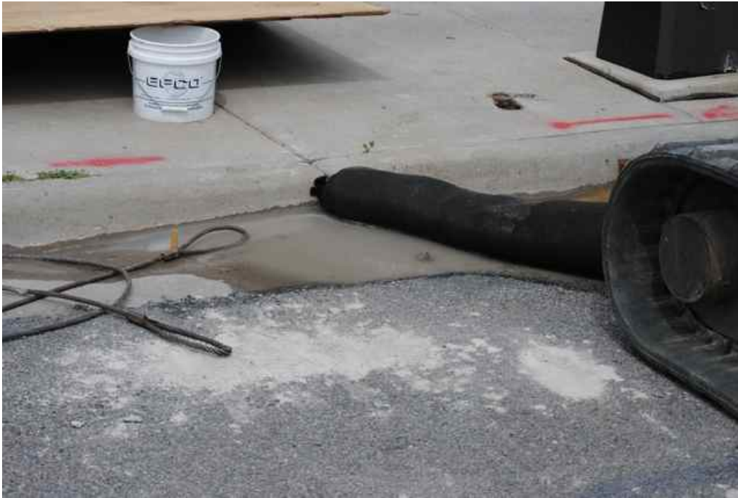
Figure 6: Filtration log placed along gutter line of Lasalle Avenue, approximately 30 feet down slope from deck being removed. Note concrete sediments both wet and dry.
