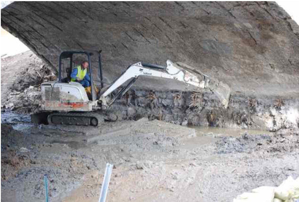
Figure 3: Foundation excavation.
