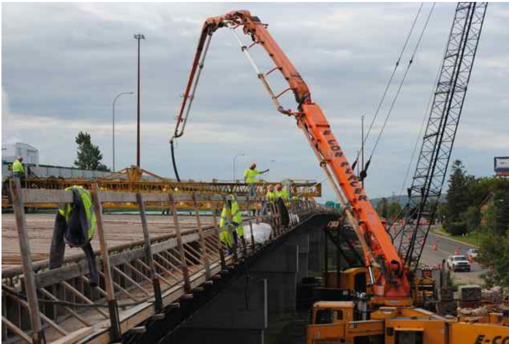
Figure 1: Concrete pumping and delivery to deck pour of elevated highway.
