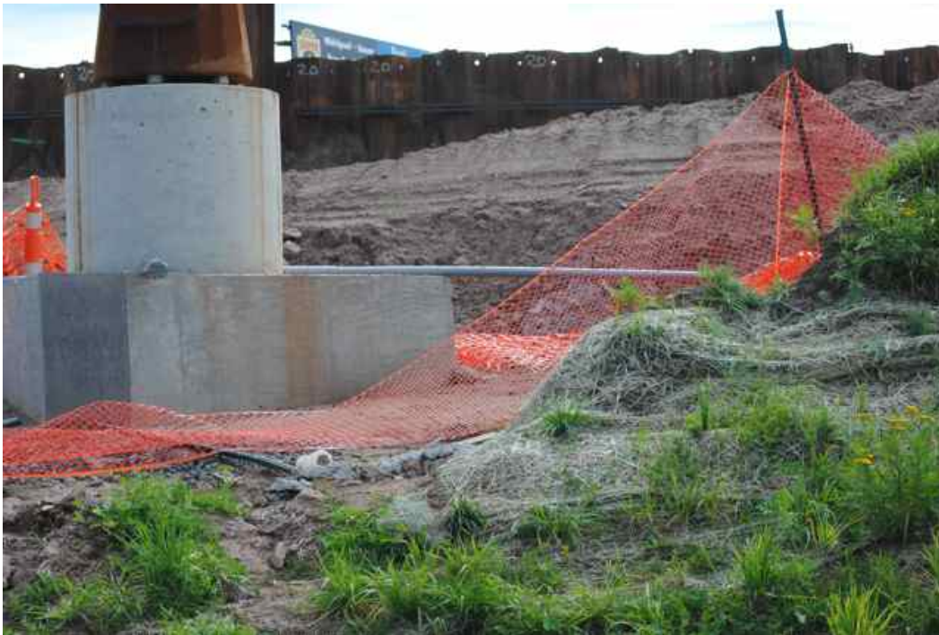
Figure 1: High mast light pole foundation adjacent to new embankment next to tied back sheet pile wall. Note disturbed ground with disrupted sediment control measures.
