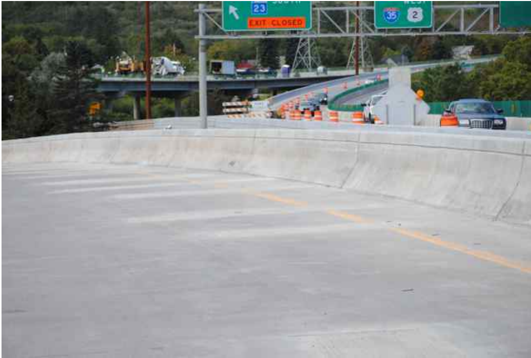
Figure 2: Concrete pavement after profile grinding, with residual fines on surface.
