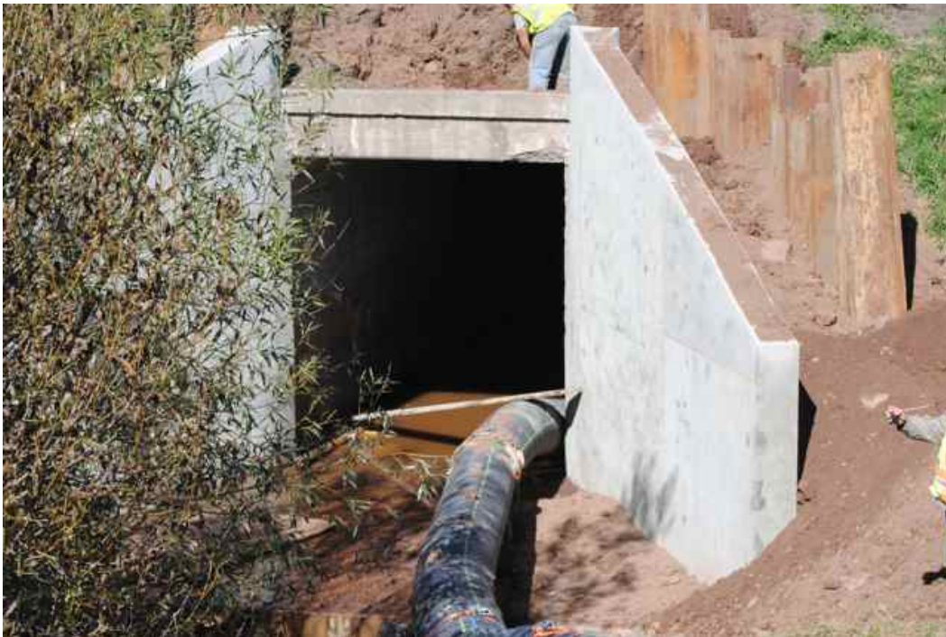
Figure 3: Bypass pipe exiting from culvert adjacent to new concrete wing walls.
