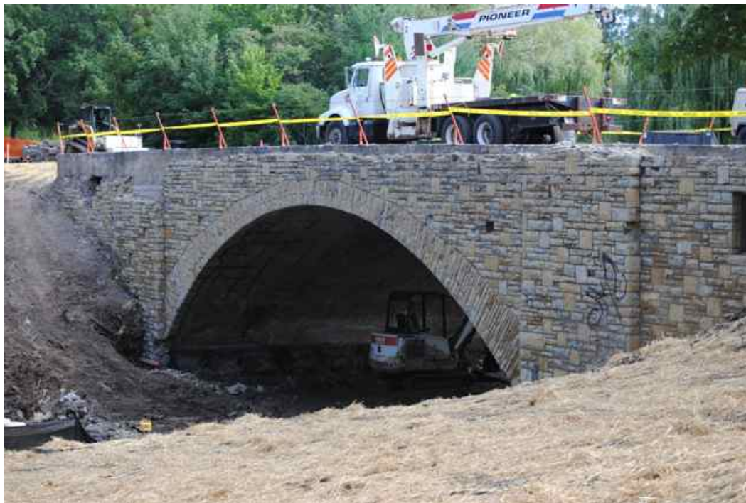
Figure 1: Concrete arch bridge with underlying stream bed cofferdammed off to allow for foundation excavation prior to reinforcing arch member placement.
