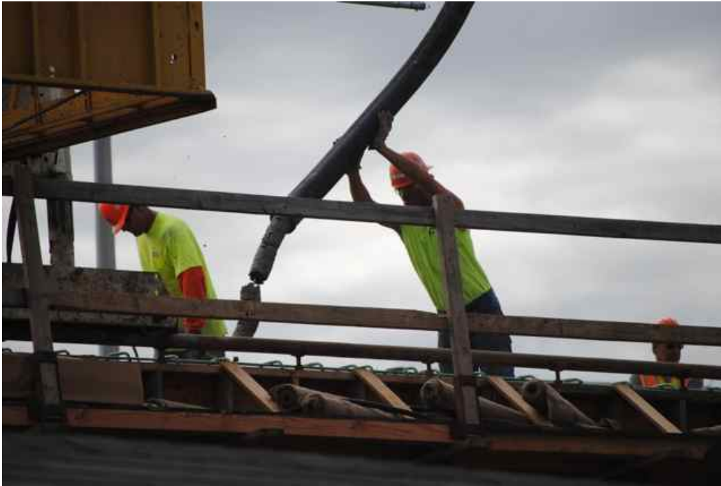
Figure 2: Concrete delivery for deck pour.
