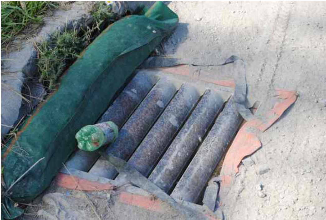
Figure 7: Catch basin protection (Dandy bag and rock filter log) overwhelmed by sediment at bottom of ramp in Figures 4 and 6.
