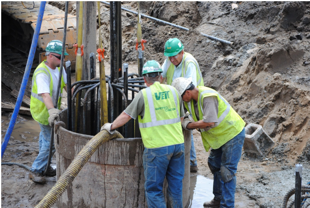
Figure 1: Drilled shaft for onshore bridge pier at a depth of 75' below ground surface. Polymer slurry used to stabilize the sides of the shaft excavation. Water and slurry mixture is being pumped out of the piling in preparation for tremie placement of concrete.
