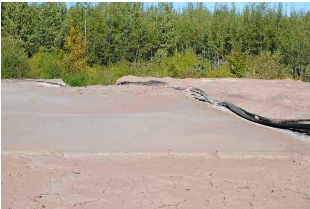
Figure 5: Containment dike failure, second concrete pavement grinding sediment disposal lagoon.
