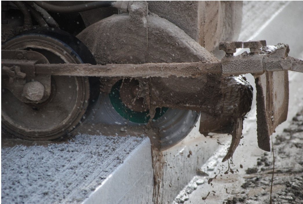
Figure 2: Saw cut edge showing slurring generation.
