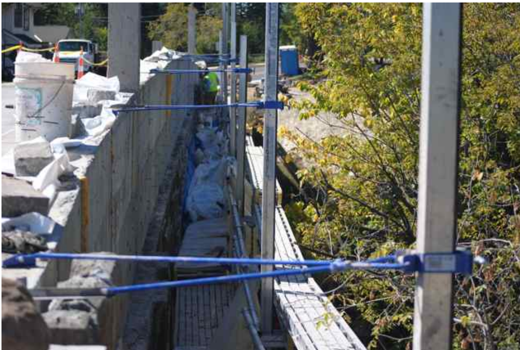
Figure 3: Chemical and debris catch system with discontinuities, view from below.
