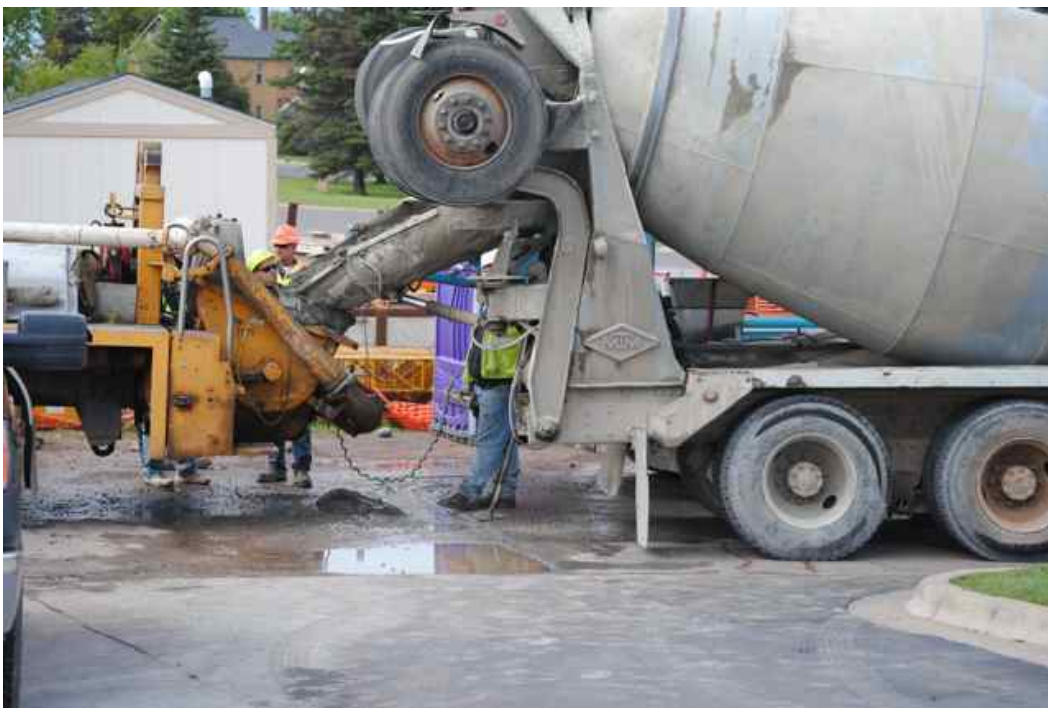
Figure 3: Concrete ready mix truck delivering to concrete pump hopper, with water and sediment on grade in vicinity of hopper.
