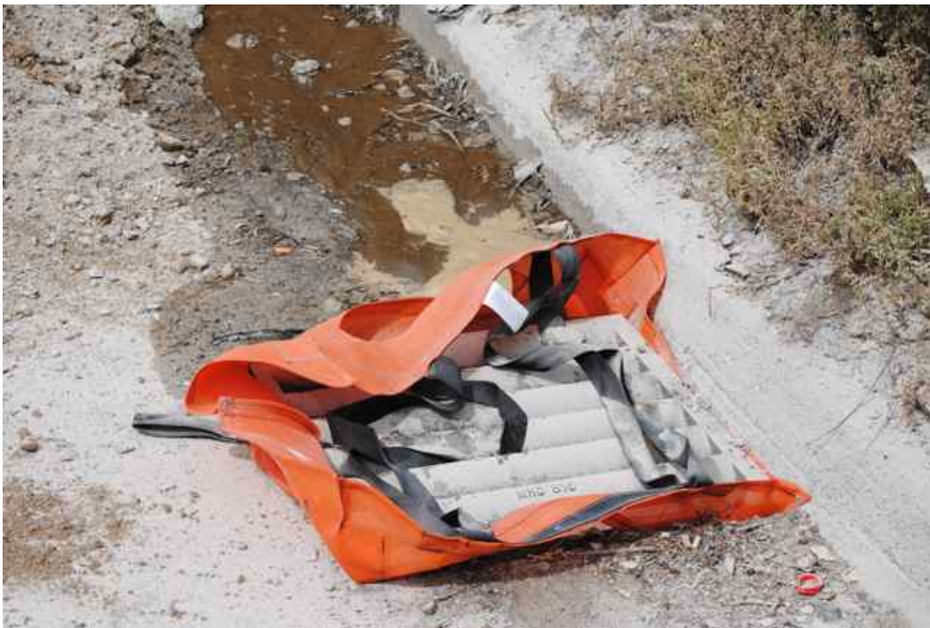
Figure 5: Woven geotextile catch basin liner (Dandy Bag) placed along I-94 gutter line, approximately 250 feet down slope from concrete debris pile. Note dust control water, sand and concrete sediments, plus urban sediments on both sides of the catch basin.
