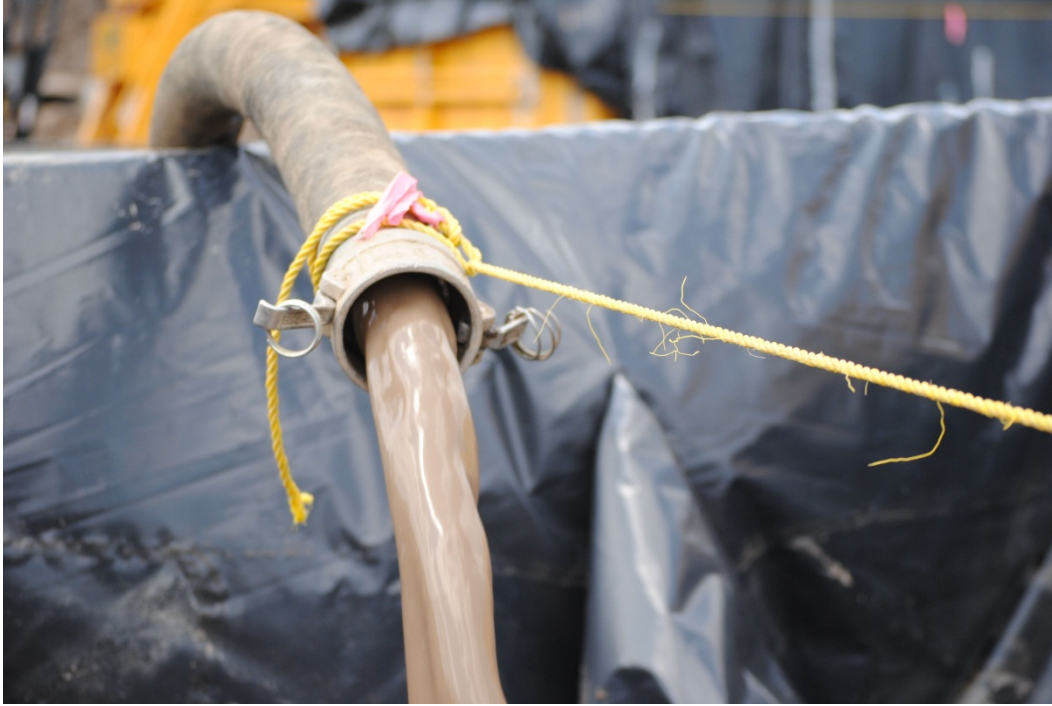
Figure 2: Polymer slurry mixture pumped from the shaft excavation (shown in Figure 1) entering treatment system located in a lined roll off box. Treatment consists of clarification of larger solids and biodegradation of the polymer.
