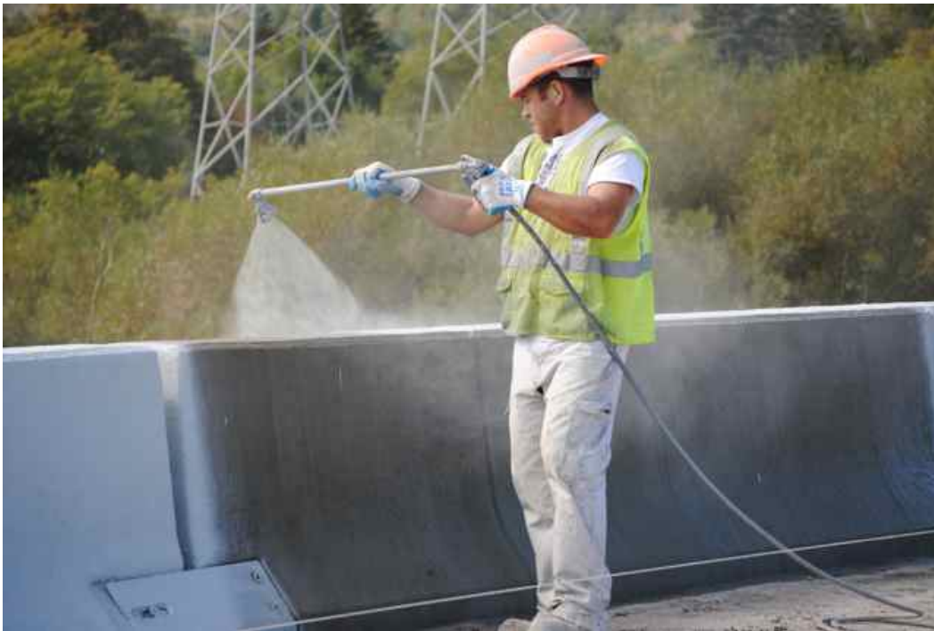
Figure 3: Curing compound application to newly poured parapet.
