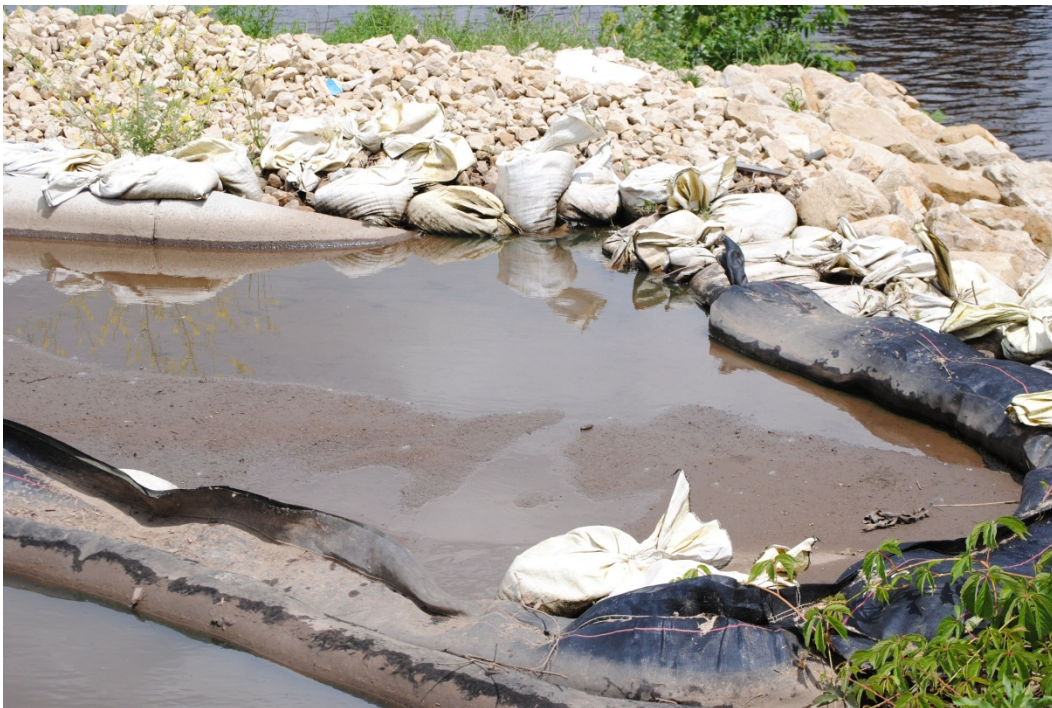
Figure 3: Upon completion of biodegradation process described in Figure 2, water is placed in sediment pond to flow through filter logs and rock bags then discharged.
