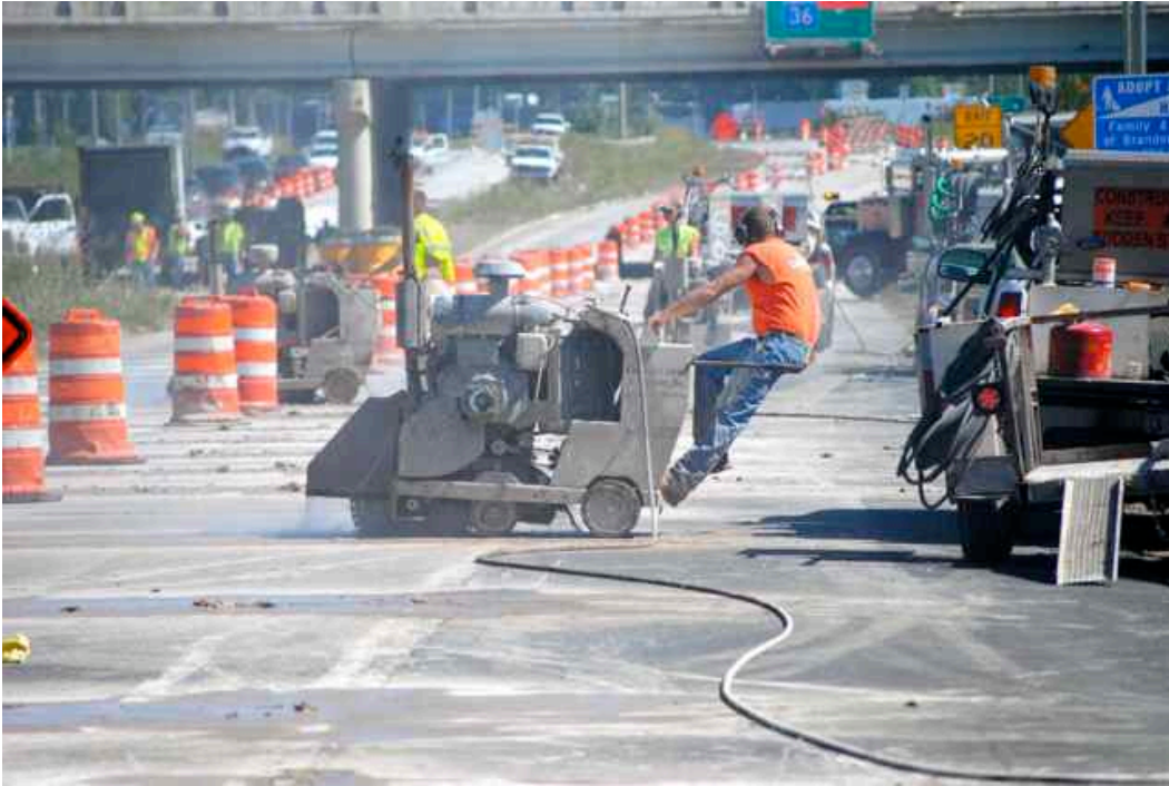
Figure 2: Saw cutting prior to removal of damaged concrete using a fleet of saws.
