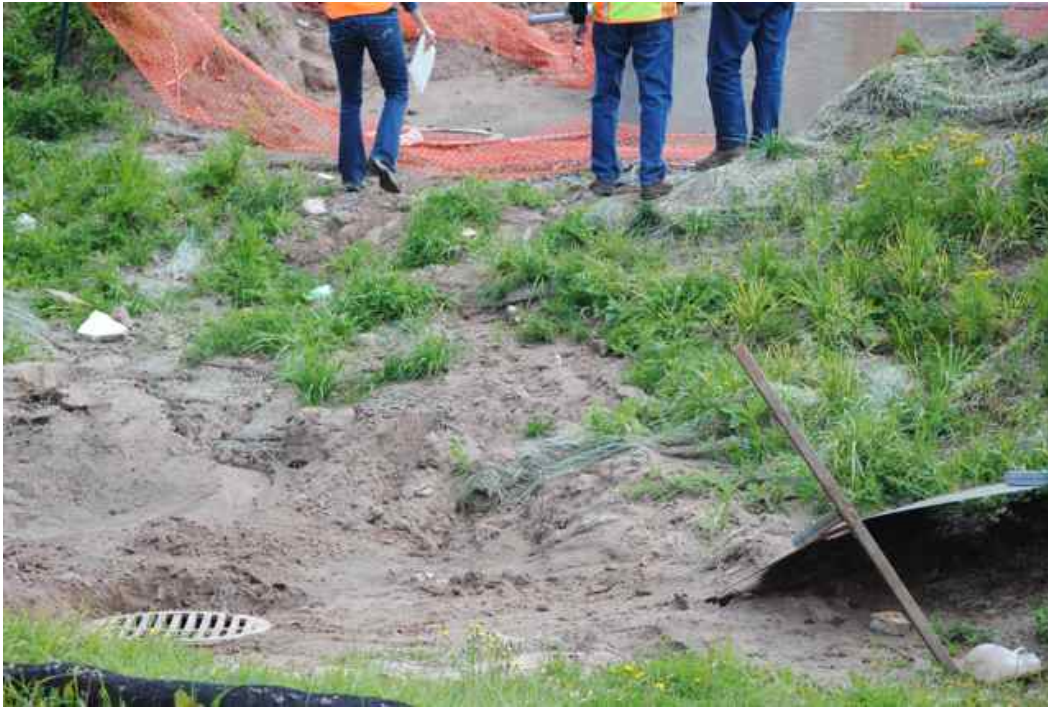
Figure 2: Ground surface immediately down slope of high mast light pole foundation showing disturbed ground and lack of inlet protection.
