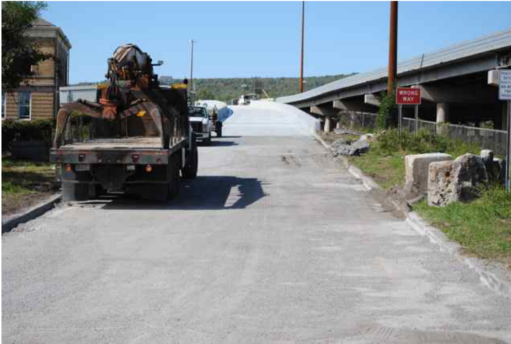
Figure 6: Concrete pavement grinding sediments remaining after incomplete sweeping effort (view up ramp towards location in Figure 4).
