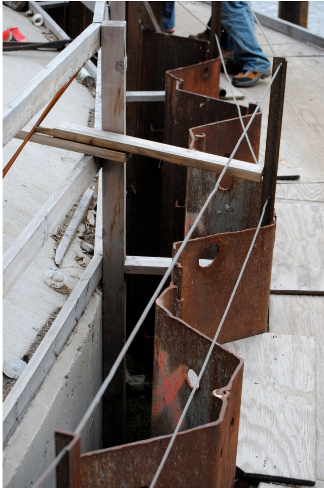
Figure 5: View from the top of the sheet piles on the cofferdam perimeter showing the recently poured concrete pier.
