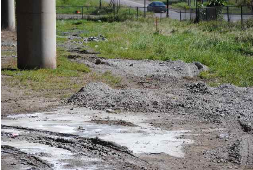
Figure 10: Fugitive concrete pavement grinding sediment dropped from elevated highway with no stormwater control (adjacent to ramp of Figure 6).
