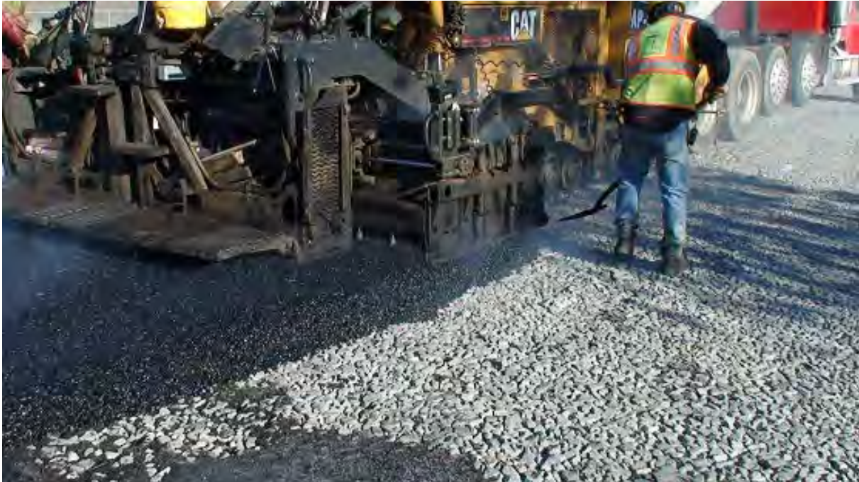
Figure 4.8. Porous asphalt paving
