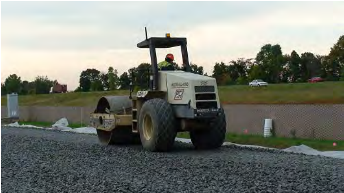
Figure 4.6. Light rolling to seat base material
