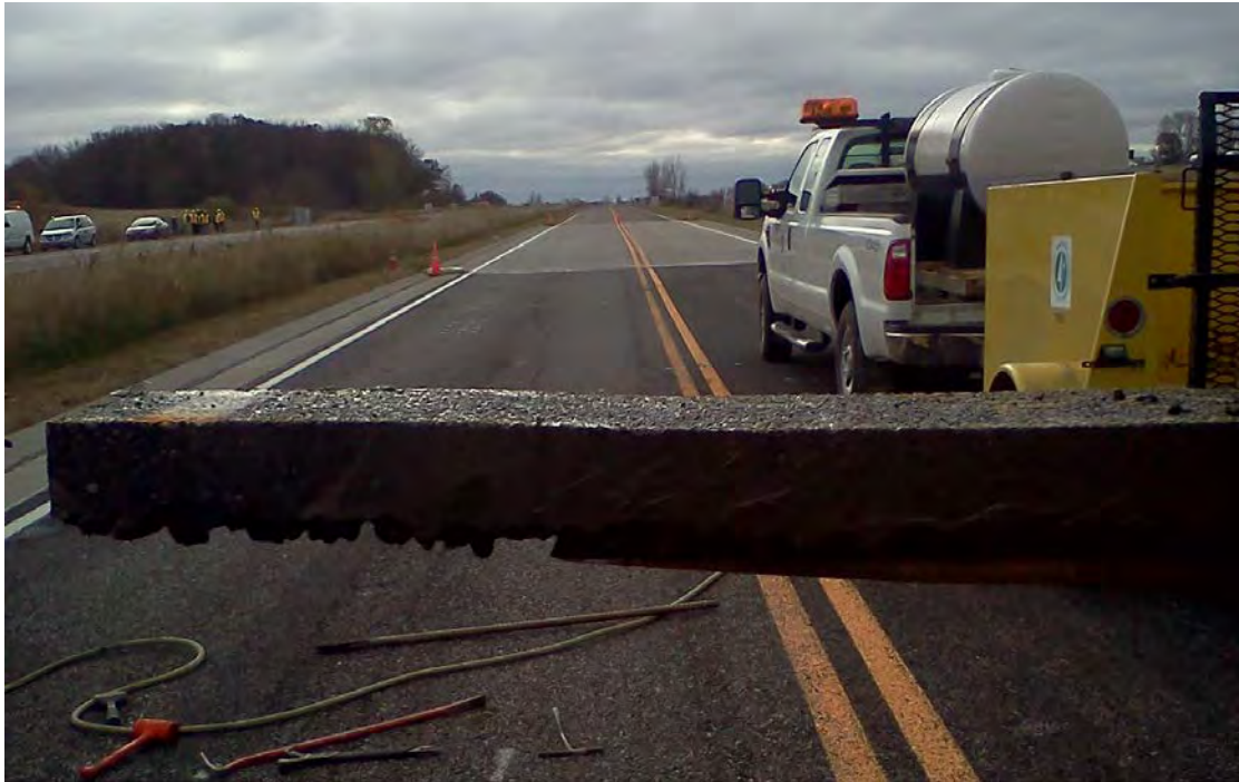
Figure 5.20. Forensic pavement section removed
