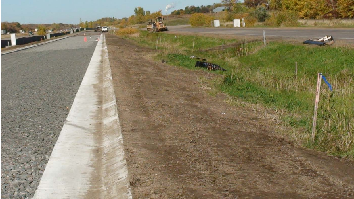
Figure 4.7. Curbing and shoulder installation
