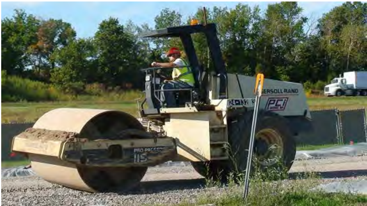
Figure 4.4. Placement of CA-15 base material
