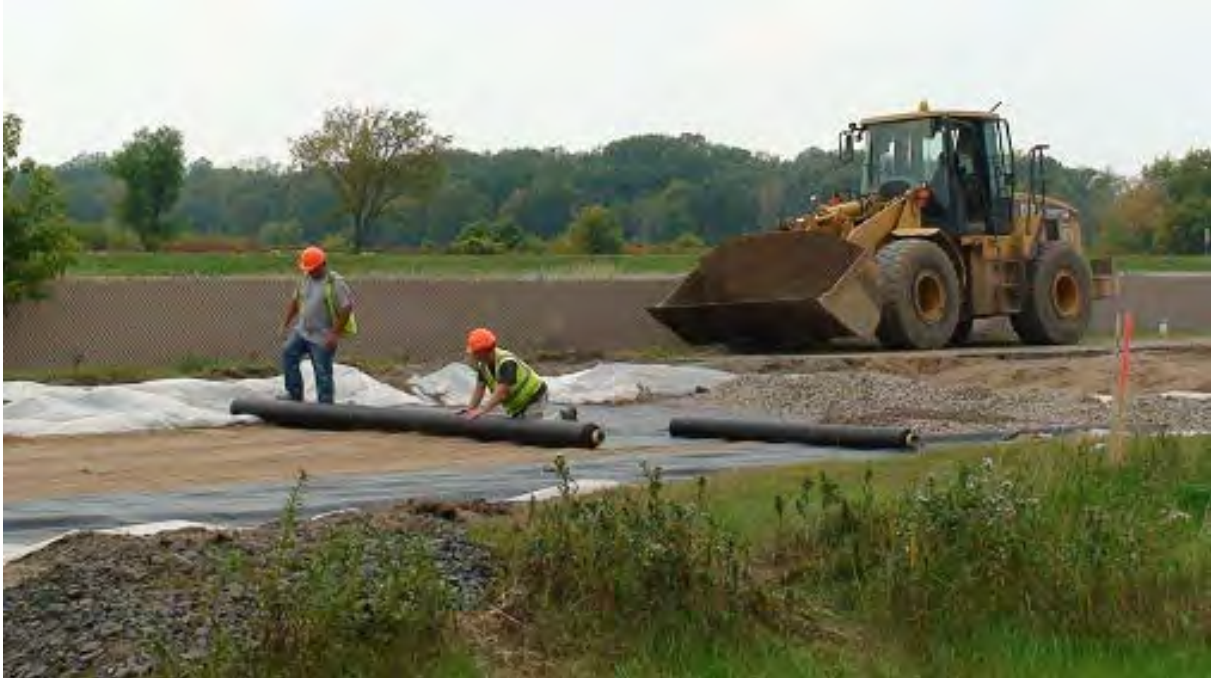
Figure 4.3. Installation of type V geotextile
