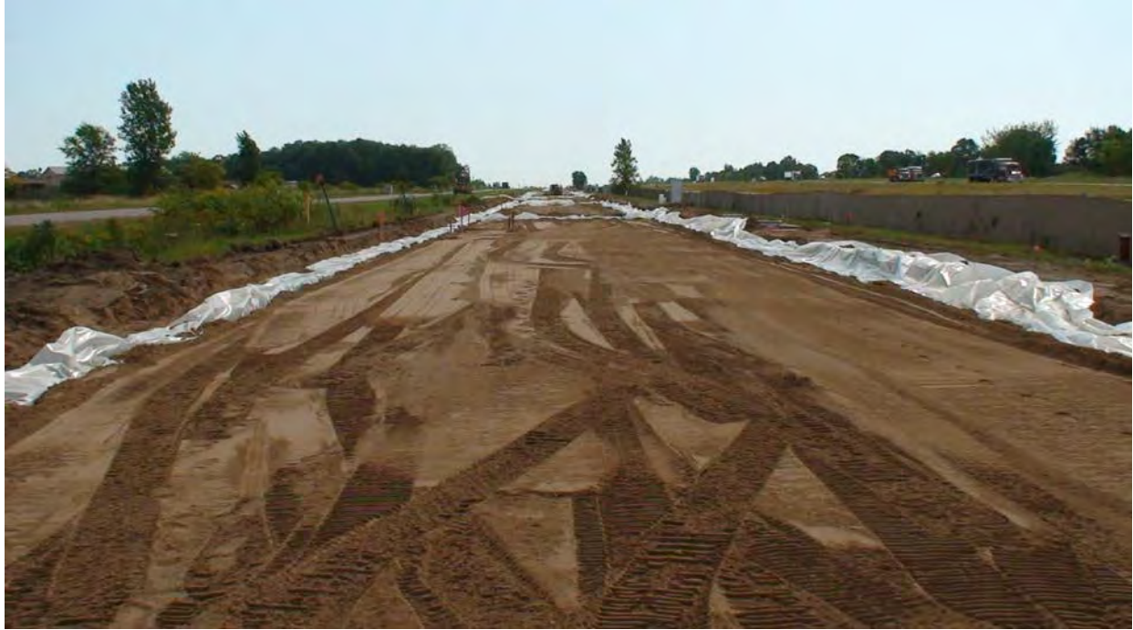
Figure 4.2. Cell 88 (clay subgrade) with plastic edge barriers installed
