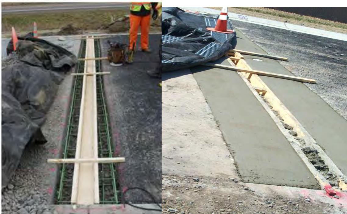
Figure 4.10. Cell-separating transverse drains
