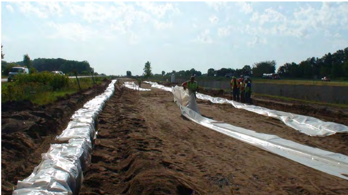
Figure 4.1. Cell 86 (sand subgrade) installing plastic edge barriers
