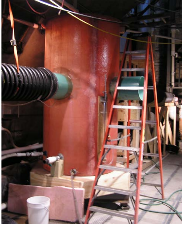
Figure 2.1. 4×4ft Sump and Test Stand
