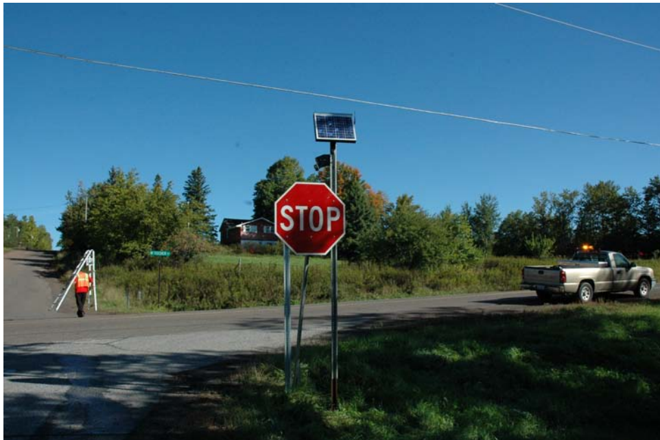
Figure 44: Installed radar detector.
