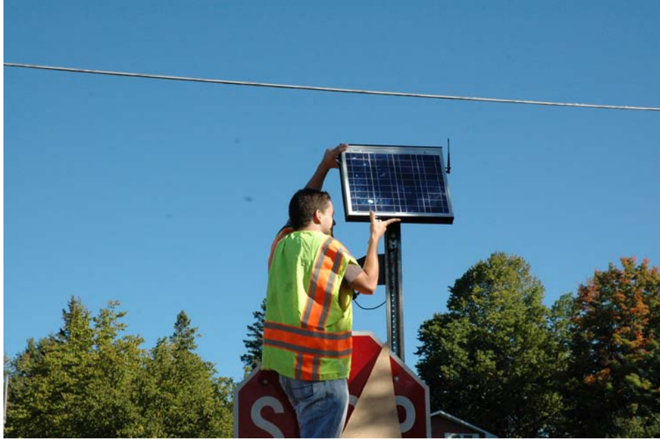
Figure 43: Adjusting the solar panel tilt angle.
