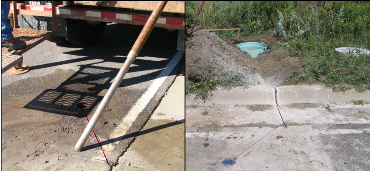
Figure 3 MDD Core and Manhole
