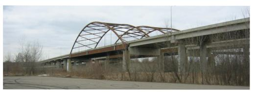
Built about 30 years ago, the Cedar Avenue bridge carries MN 77 over the Minnesota River to connect Minneapolis to the southern suburbs. It is a steel tied-arch bridge that is considered fracturecritical: The design lacks redundancy such that failure of a structural member could lead to collapse. As such, it was selected for this project to develop advanced structural monitoring systems.
