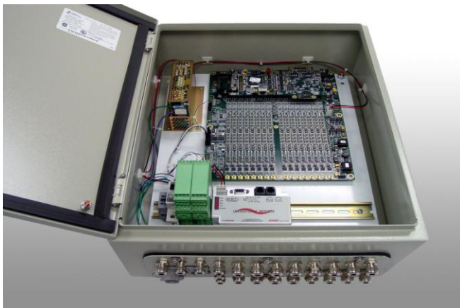
Figure 2. Inside the Sensor Highway Cabinet
