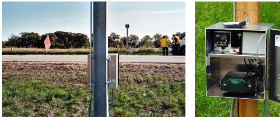
Figure 30. TIRTL Pole Mount Examples (Permanent Installation)
