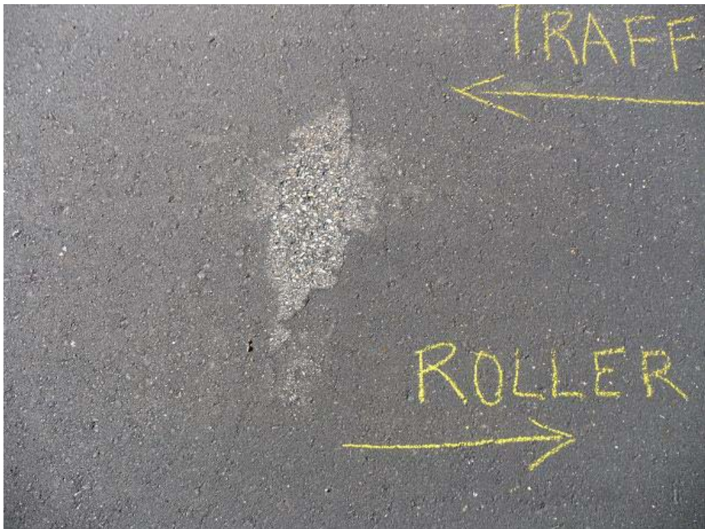
Figure 15. CSAH 15 – Section 1, Paved 1 August 2007.
