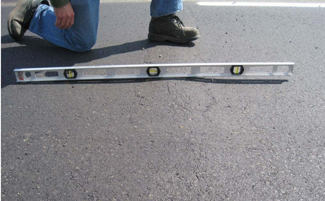
Figure 21. Severe Bump in Lower Lift on US 52.
