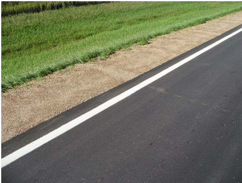
Figure 13. CSAH 15 – Section 1, Paved 1 August 2007.
