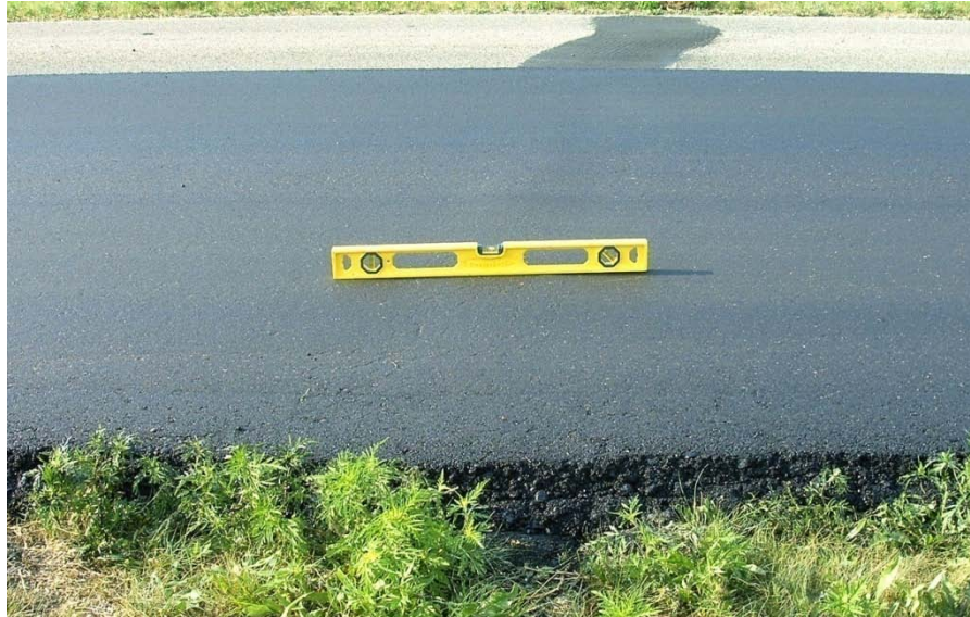
Figure 12. Bump Over Leveled Crack, Eastbound CSAH 15.
