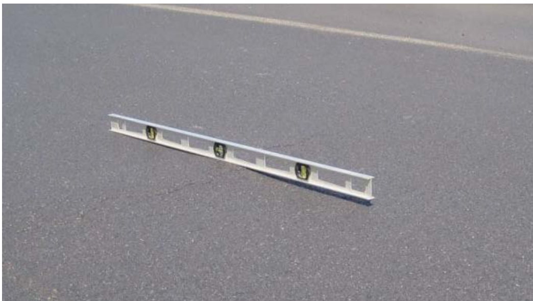
Figure 24. Bump in the Final Lift of HMA on TH 52.
