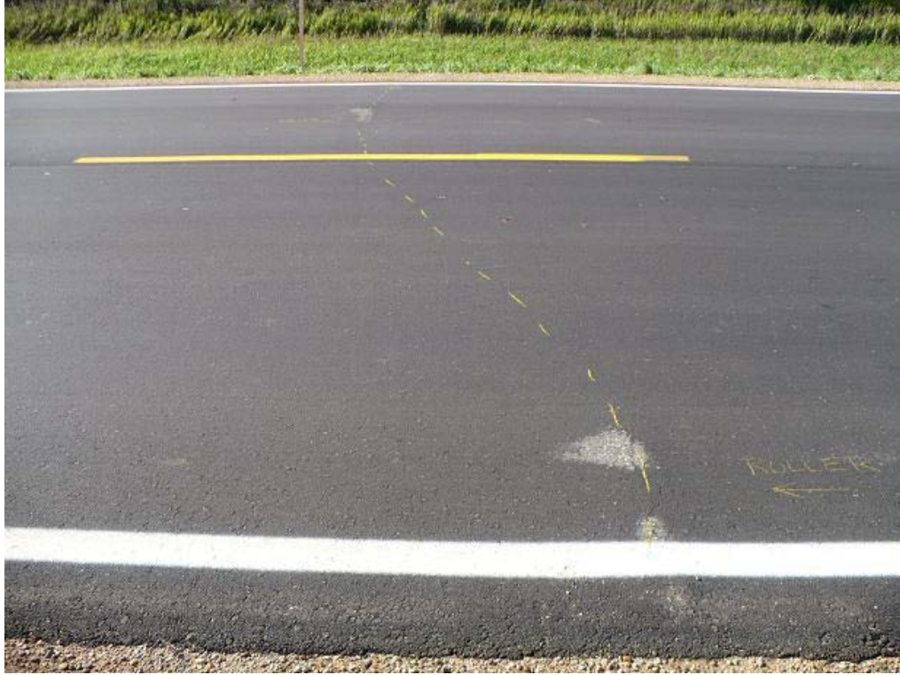
Figure 14. CSAH 15 – Section 1, Paved 1 August 2007.
