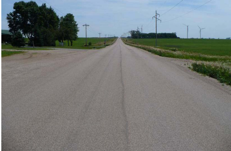
Figure 26. Chip Seal on Sealant Site.
