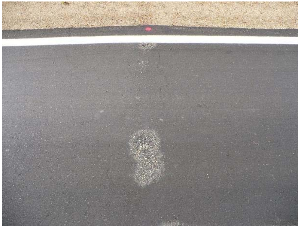
Figure 16. CSAH 15 – Section 1, Paved 1 August 2007.
