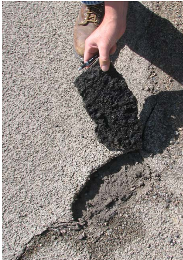
Figure 4.6. De-bonding over an asphalt repair patch.
