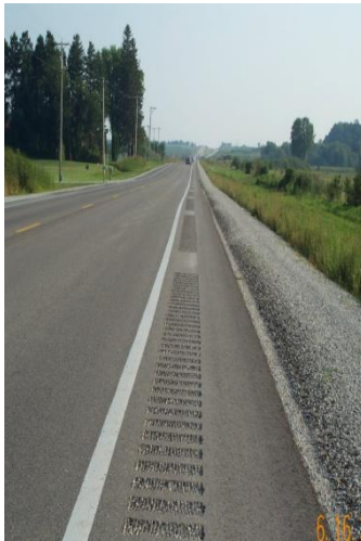
Figure 2.21 Example of Rumble Strip
