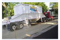
This truck laying down fly ash on RPM will be followed by a road reclaimer with tines for blending them together.
