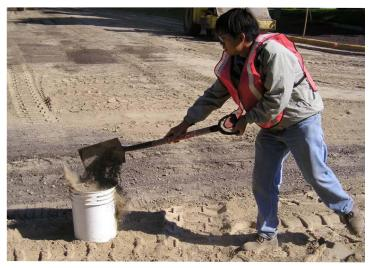
Researchers collected samples of fly ash to mix in the laboratory with samples of RPM and RSG; these stabilized samples were tested for stiffness and strength over five freeze-thaw cycles.
