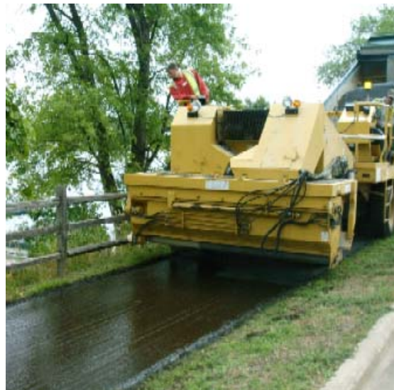
Figure 8: Rec. Trail Chip Seal in McCarrons Lake Roseville, MN
