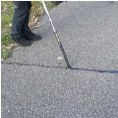
Figure 9: Flush Fill Crack Sealing
