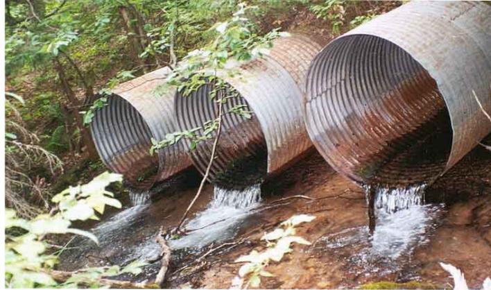
Erosion has created a dropoff distance between the water and culvert opening. Salmon swimming upstream would not be able to enter these culverts and continue their passage.
