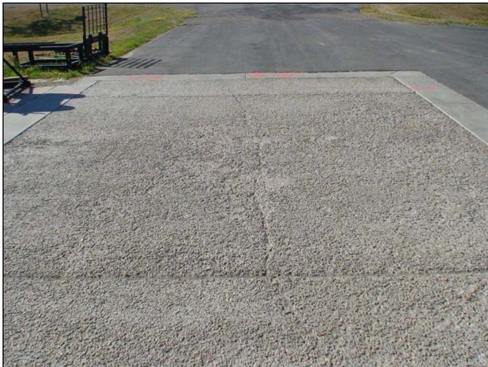
**FIGURE D-5: Header/construction joint, facing south, 8.11.08.**
