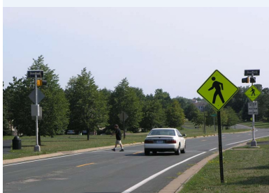
Researchers studied user-activated warning crosswalks such as this one in Woodbury, Minnesota.
