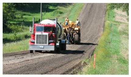
Bituminous stabilization involves laying new gravel and mixing asphalt binder to a depth that supports anticipated loads on a roadway.
