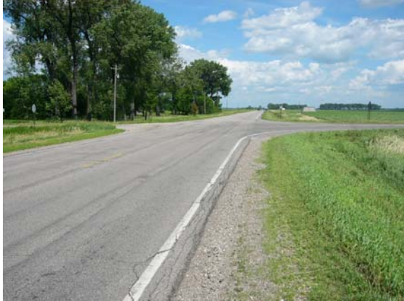
Four-legged intersection on 28th Ave. N with 40th St. N in Moorhead as viewed from the west approach
