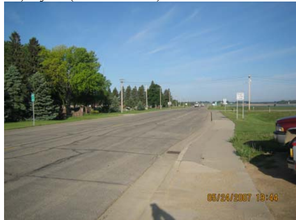
Three-legged intersection on US-14 with CR-8 in Tyler viewed from east approach
