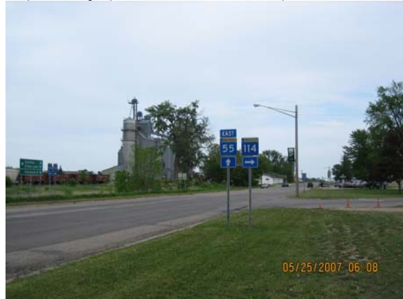
Three-legged intersection on MNTN-55 with CR-114 in Lowry viewed from west approach
