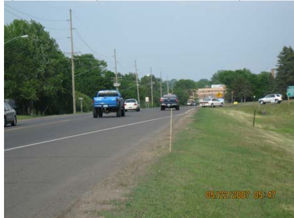
Four-legged intersection on MNTN-8 with Akerson St. in Lindstrom viewed from west approach
