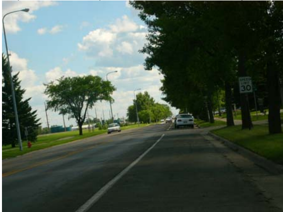
Four-legged intersection on 20th St. S with 16th Ave. S in Moorhead as viewed from the north approach
