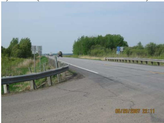
Four-legged intersection on MNTN-210 with CR-54/CR-56 near Aitkin with west approach in view (crash location – west approach)
