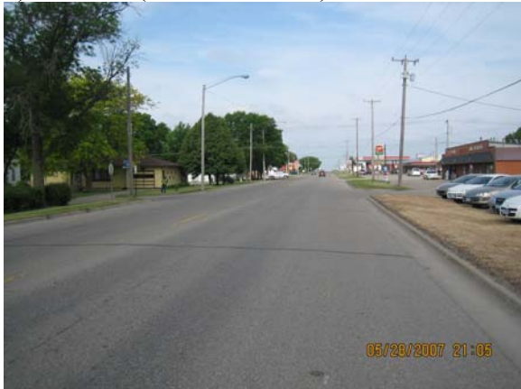
Four-legged intersection on US-212 with 4 th St. at Dawson, viewed from east approach (crash location – west approach)
