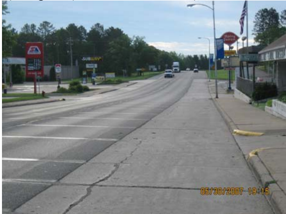
Four-legged intersection on US-10 with 12 th St. NE in Staples viewed from west approach, also shows intersecting 11 th St. NE and Subway-Dairy Queen driveways (crash location – west approach)
