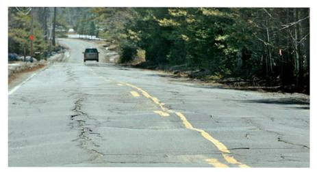
Damp subgrade and pavement may shift during expansion in freezing temperatures, causing frost heave that can severely damage surface conditions and ride quality.
