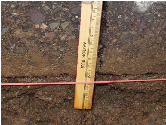
Figure 16 String line shows HMA tenting at bottom of D1 pit.
