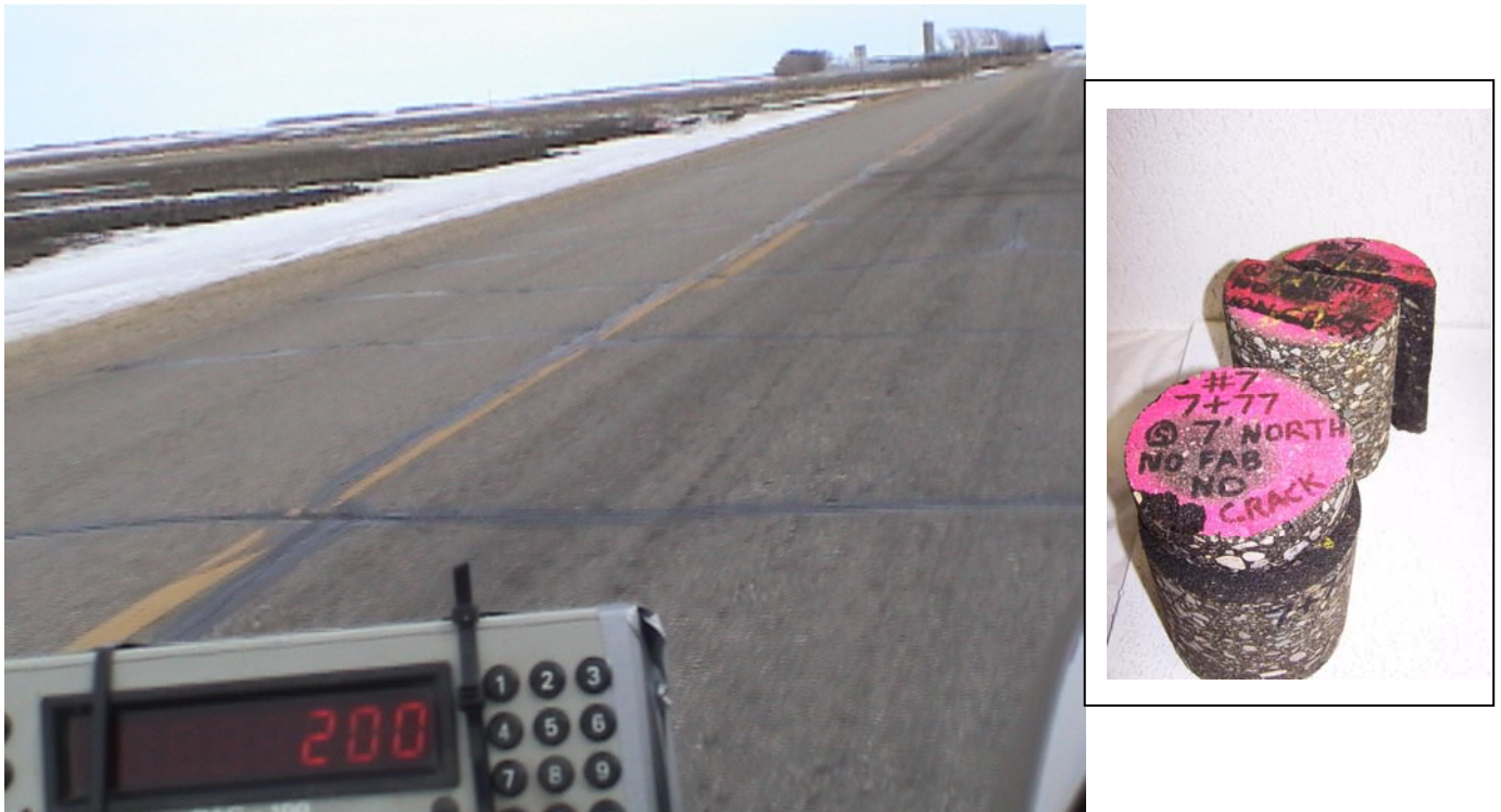
Figure 2.1 CSAH # 7: 11 ½” Base & 3” Existing Bit
