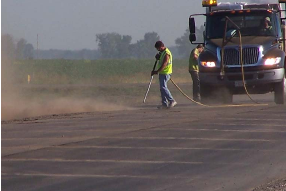
Figure 3.8 CSAH # 10 Saw & Seal
