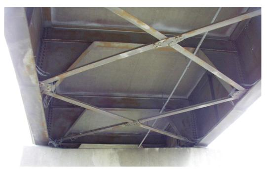
Figure 3-9: Diaphragm and Lateral Wind Bracing at Pier 8
