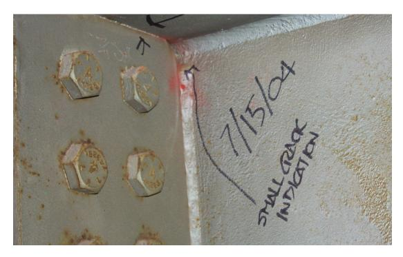
Figure 5-26: Small Crack in Weld at Diaphragm Connection South of Pier 8 on Girder C
