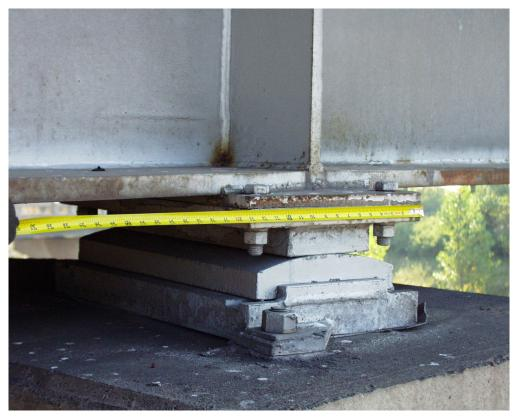
Figure 3-14: Expansion Bearing at Pier 9
