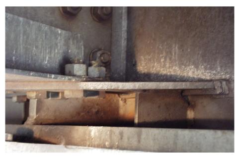
Figure 3-11: Gusset Plate Connection
