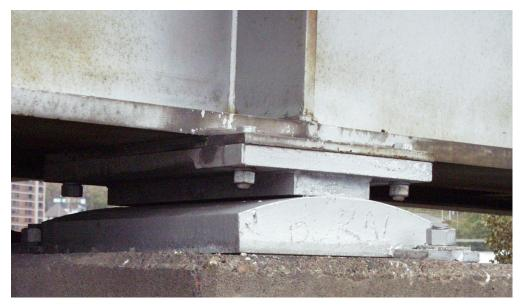
Figure 3-15: Fixed Bearing at Pier 8
