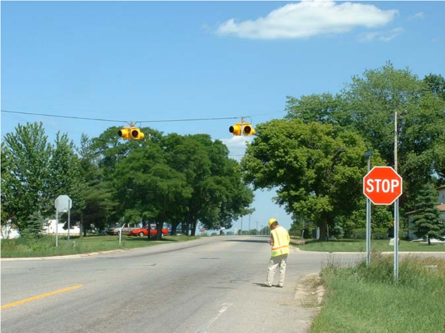
FIGURE 5-2 Red/Yellow Warning Flashers Located at Intersection
