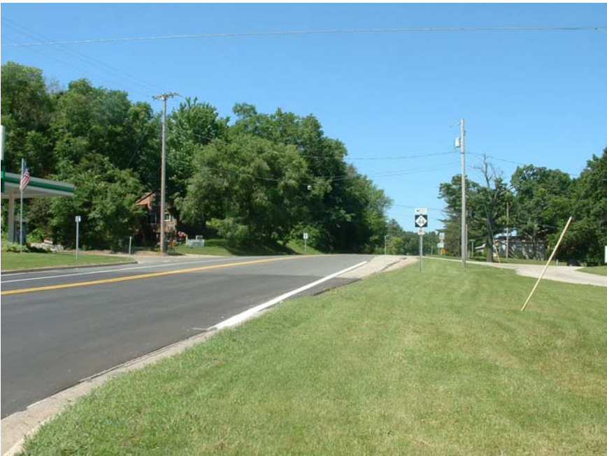
FIGURE 5-12 Restricted Sight Distance Due to Crest Vertical Curve Located West of Intersection
