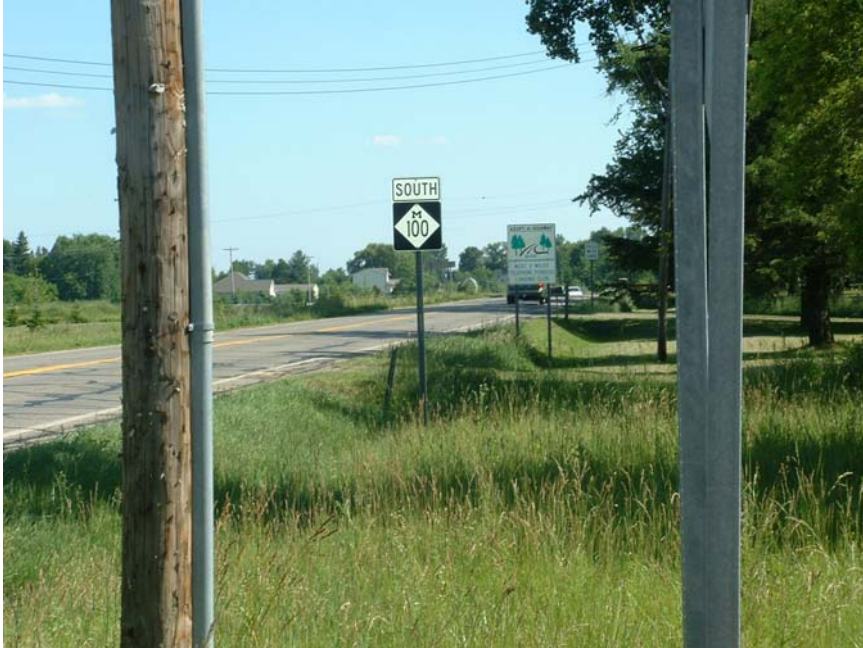
FIGURE 5-7 Cluttered Line of Sight While Stopped on the West Approach
