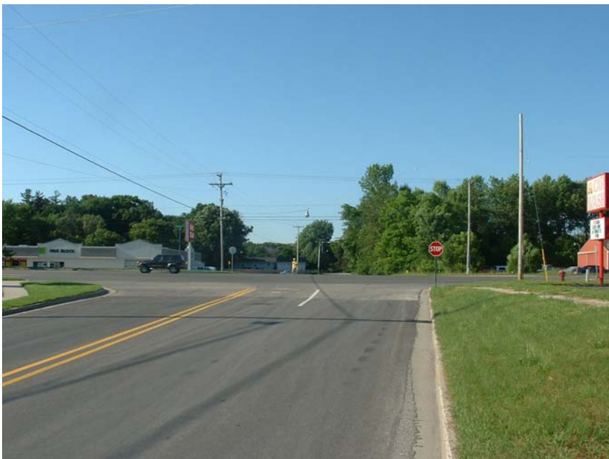
FIGURE 5-14 Vance Road North Approach
