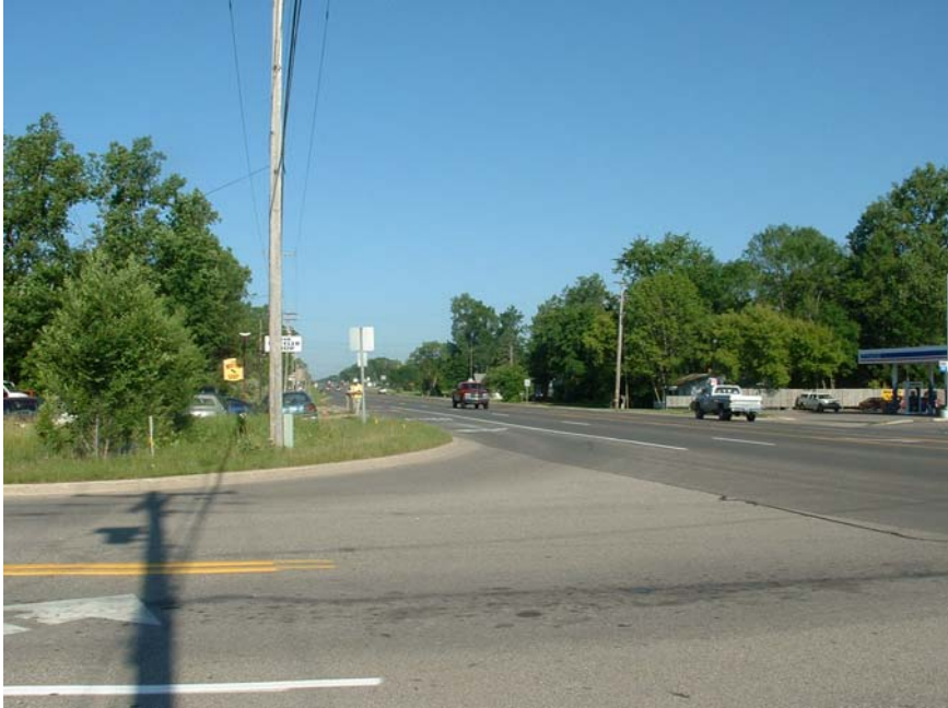
FIGURE 5-13 M-20 West Approach
