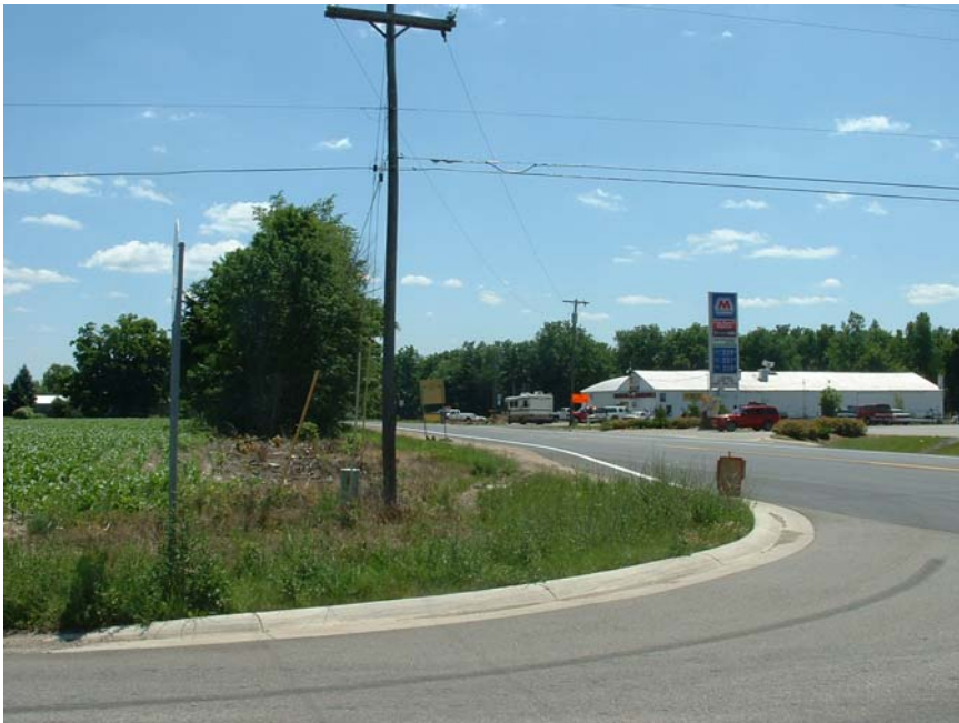
FIGURE 5-8 Restricted Sight Distance When Stopped at STOP Sign (Looking South from East Approach)
