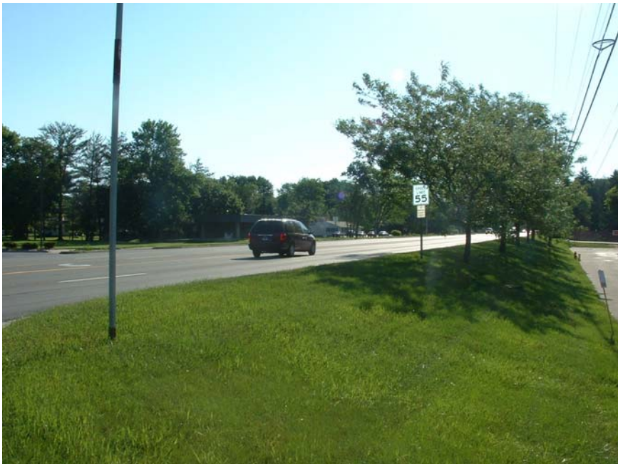
FIGURE 5-16 Intersection Sight Distance Restricted by Low Hanging Branches
