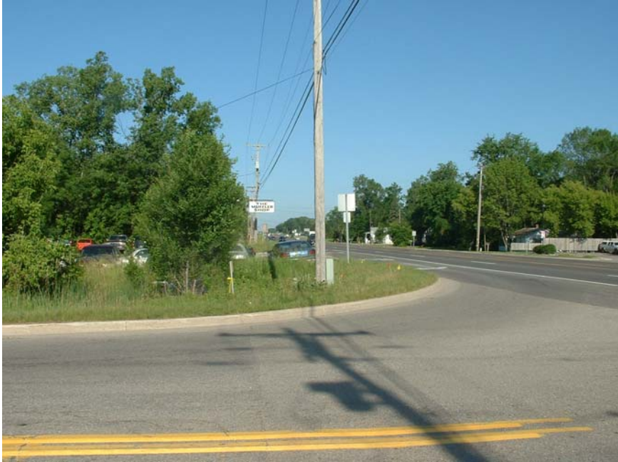
FIGURE 5-15 Intersection Sight Distance Restricted by Vehicles at Repair Shop
