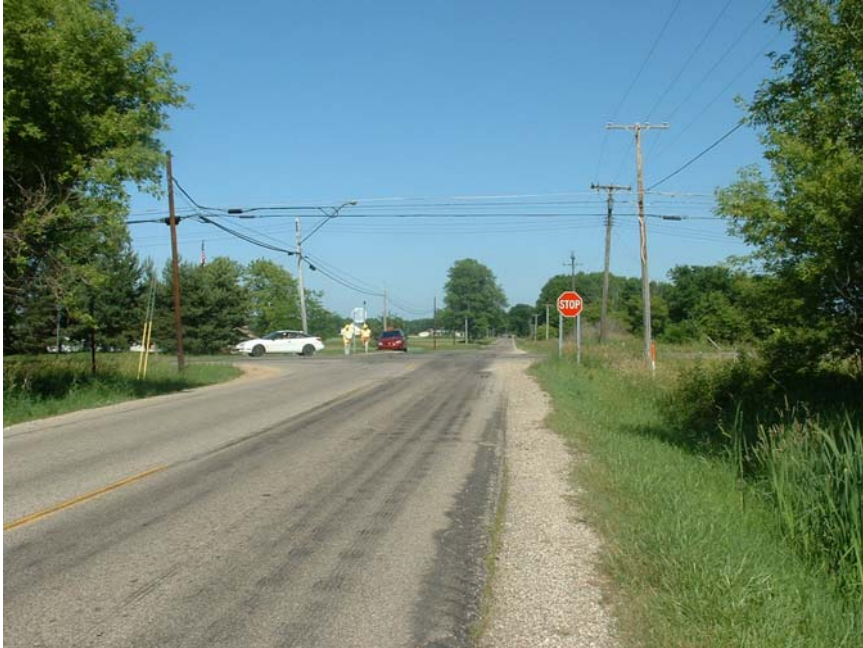
FIGURE 5-5 West Approach of Mount Hope Highway (Looking East)
