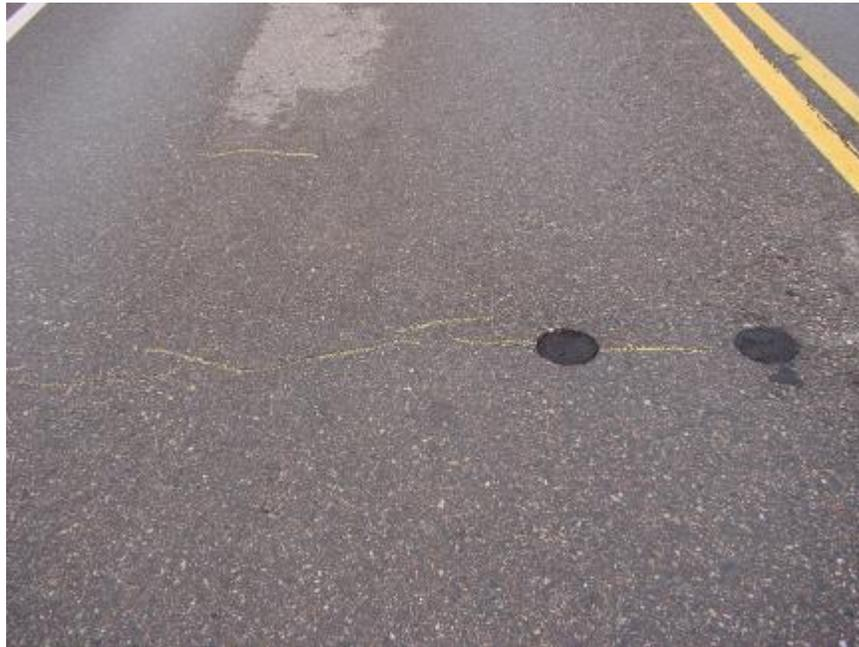
**Figure 1.6. Typical Transverse Crack in Superpave Cells**
