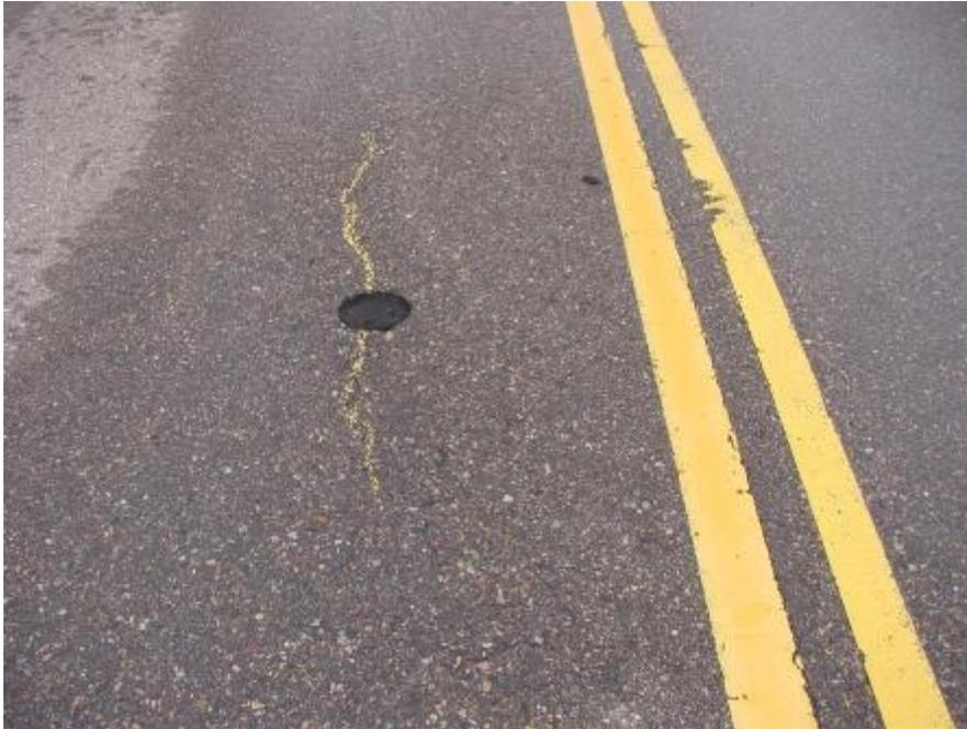
**Figure 1.7. Typical Longitudinal Crack in Superpave Cells**
