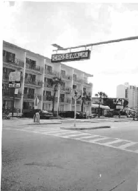
Figure 6.1. The use of overhead crosswalk signs at an intersection in Clearwater, FL.
