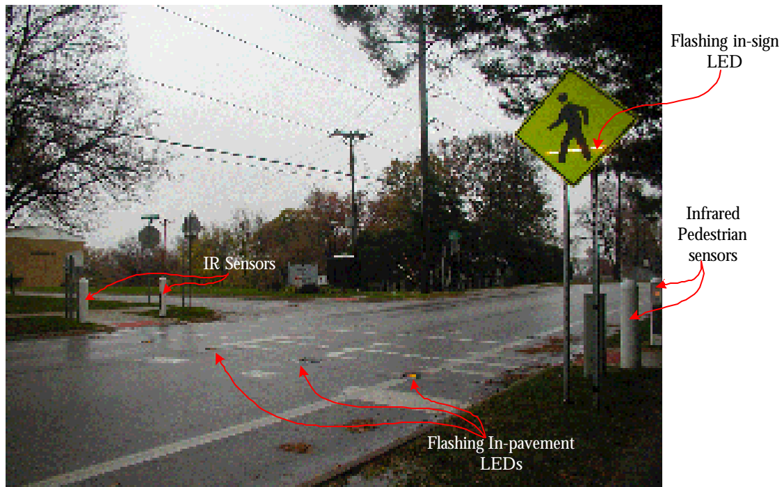
Figure 6.12. An in-ground and in-sign flashing LED crosswalk application in Iowa City, IA.
