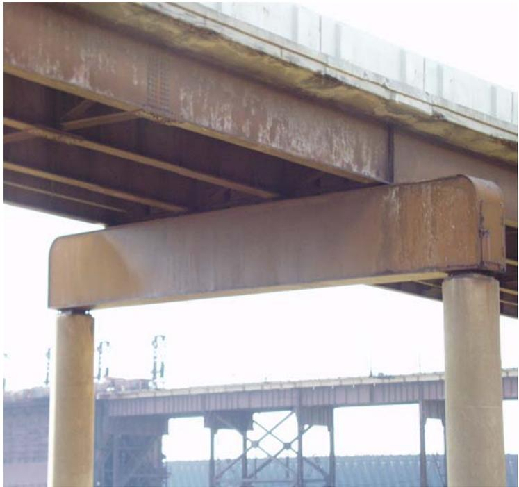
Figure 2.3: Steel pier cap with girders bearing on top
