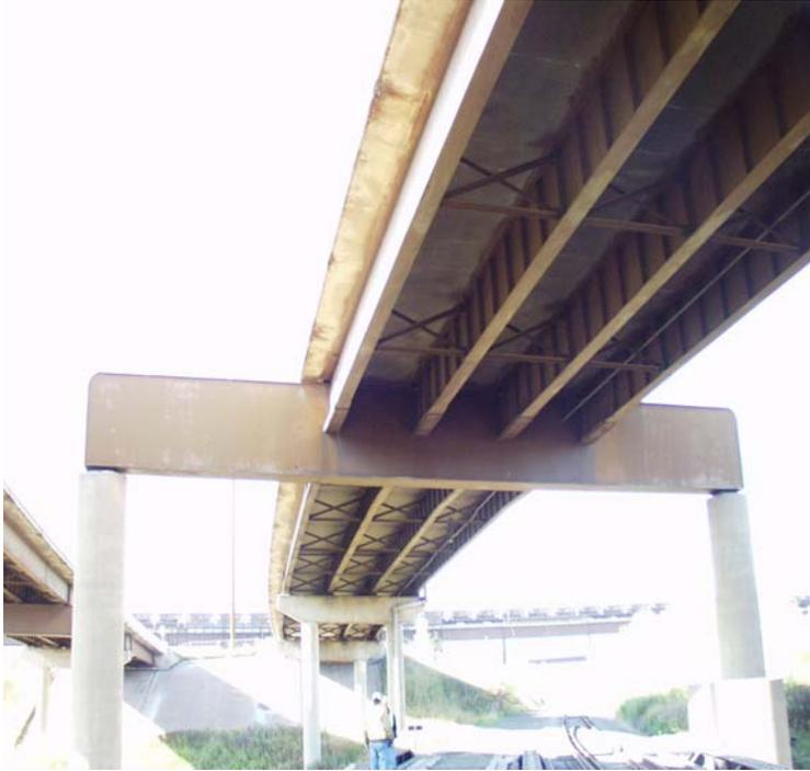
**Figure 2.4: Steel pier cap with girders continuous through pier cap**
