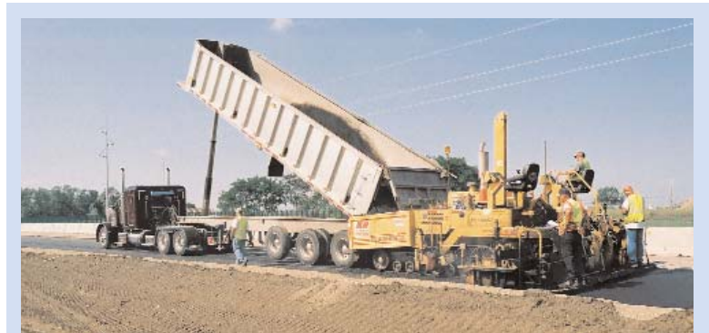
Bituminous Road Paving Crew
