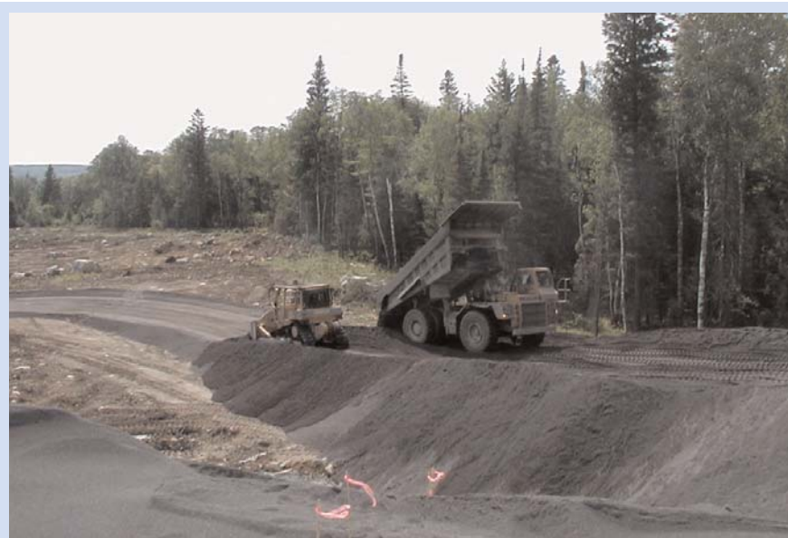
Construction on TH 53 North of Virginia
