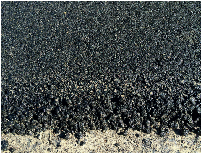
Pavement being constructed with 20% and 40% RAP (CSAH 18 in Lake County, MN)
