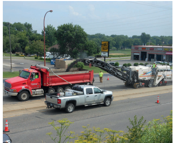
Road being milled and material collected for RAP use
