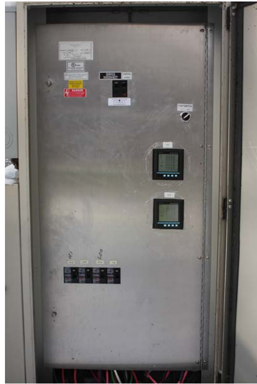
Figure 1.2 Cabinet Deadfront photo
