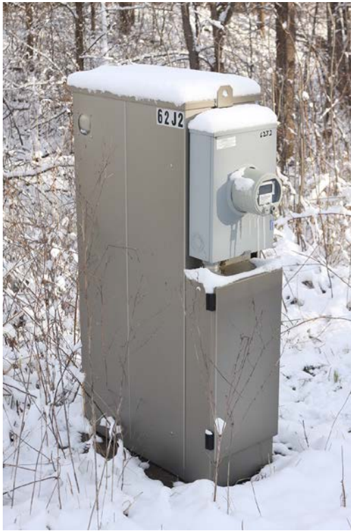
Figure 1.1 Service Cabinet photo
