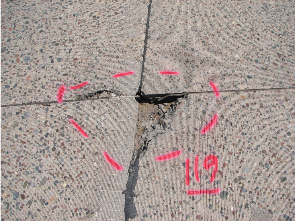
Figure 1.1 Distress near the surface of a concrete pavement at intersection of transverse and centerline joints.
