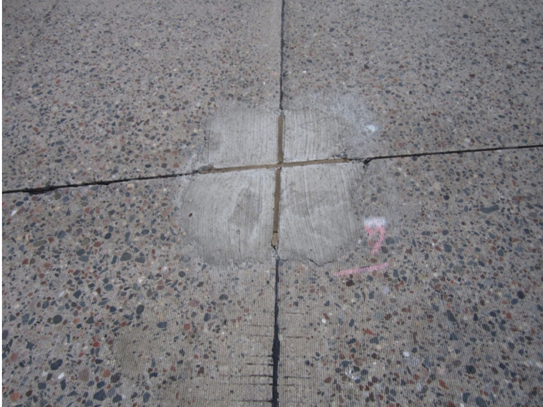
Figure 1.4. Typical MnROAD partial-depth repair with cementitious-based material.
