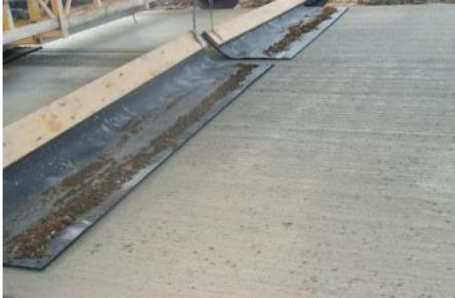
Figure 2.18: Turf Finish of Concrete Pavement
