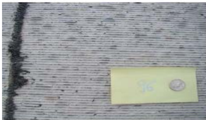
Figure 4.155: 2004 Drag, 2011 Grind Of Drag Surface, 2011 Grind of Tined Surface
