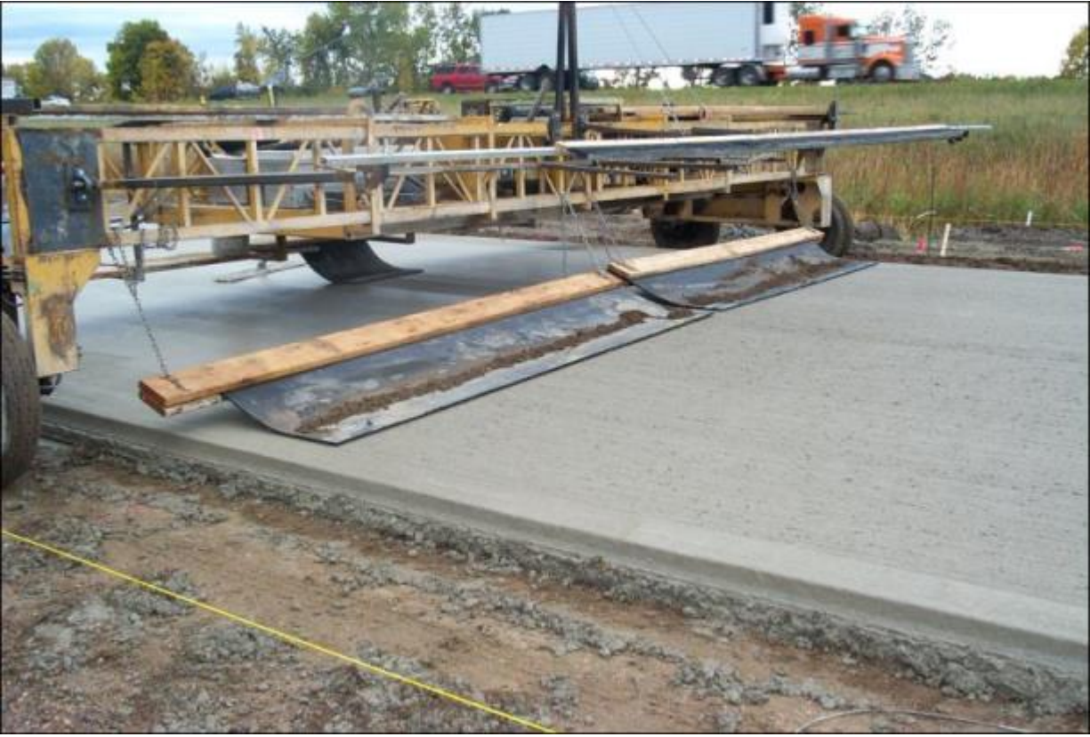
Figure 2.17: Broom Drag Texturing of Cell 13
