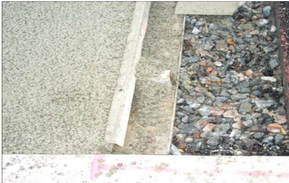
Figure 2.10: Cell 85 and Proximate Cross Drain Prior to Concreting (Rail Road ballast Base is exposed.)
