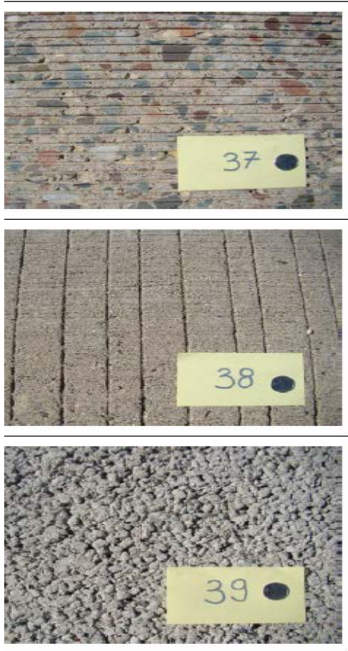
Figure 4.152: Innovative Grind, Transverse Tine, Pervious Concrete
