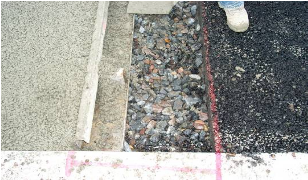
Figure 2.8: Cell 89 Pervious Concrete on Clay and Cell 88 Pervious Asphalt on Clay.
