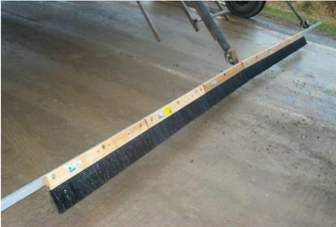
Figure 2.16: Broom Drag Used for Texturing of Cell 13 and Cell 53
