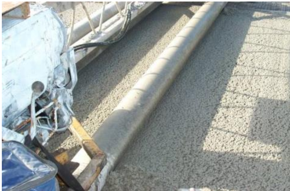
Figure 2.6: Pervious Overlay Multi-Drum Screed Compactor
