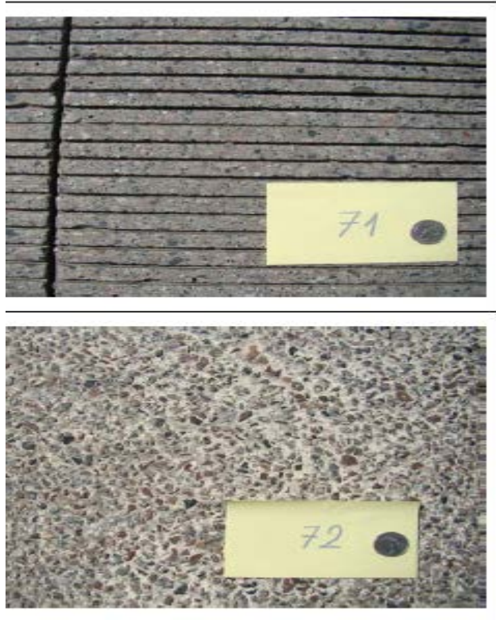
Figure 4.156: 2011 Innovative Grind, 2011 Exposed Aggregate
