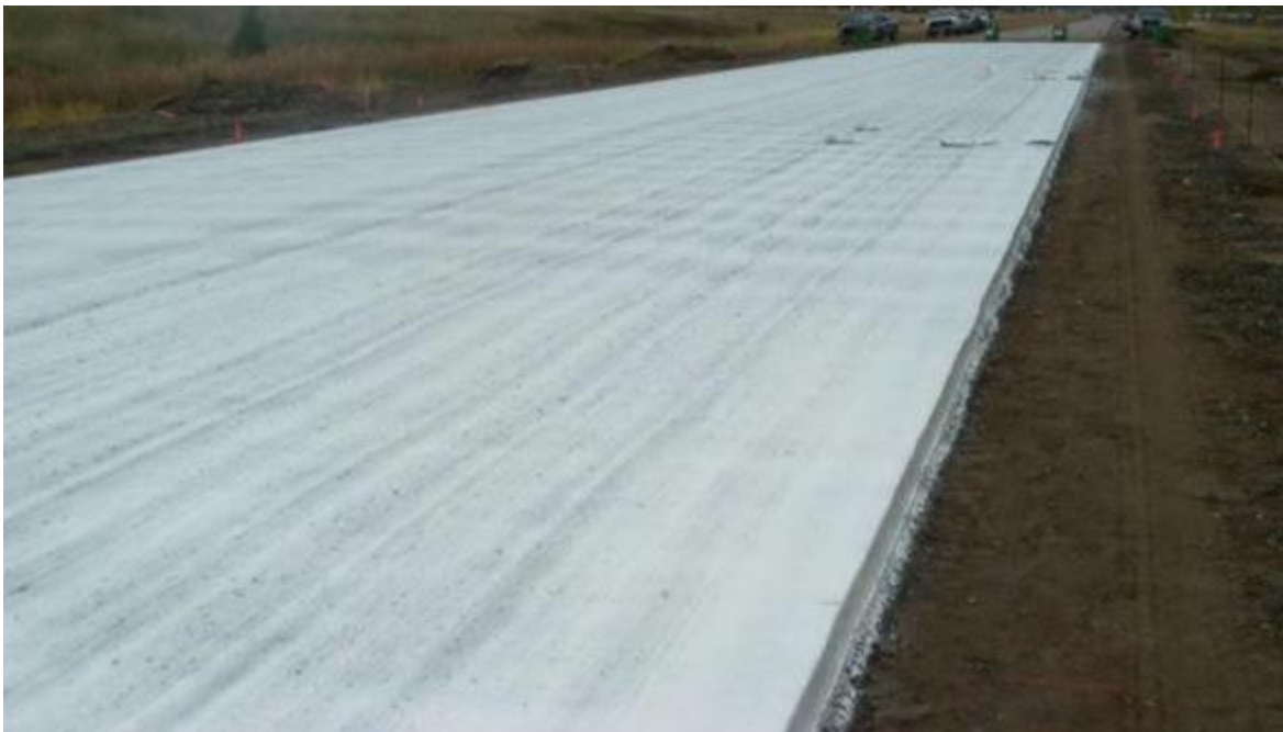
Figure 2.15: Finished Surface with Alpha Methyl Styrene (AMS) Curing Compound
