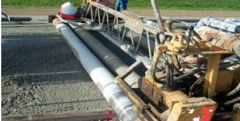
Figure 2.5: Pervious Concrete Placement and Vibration
