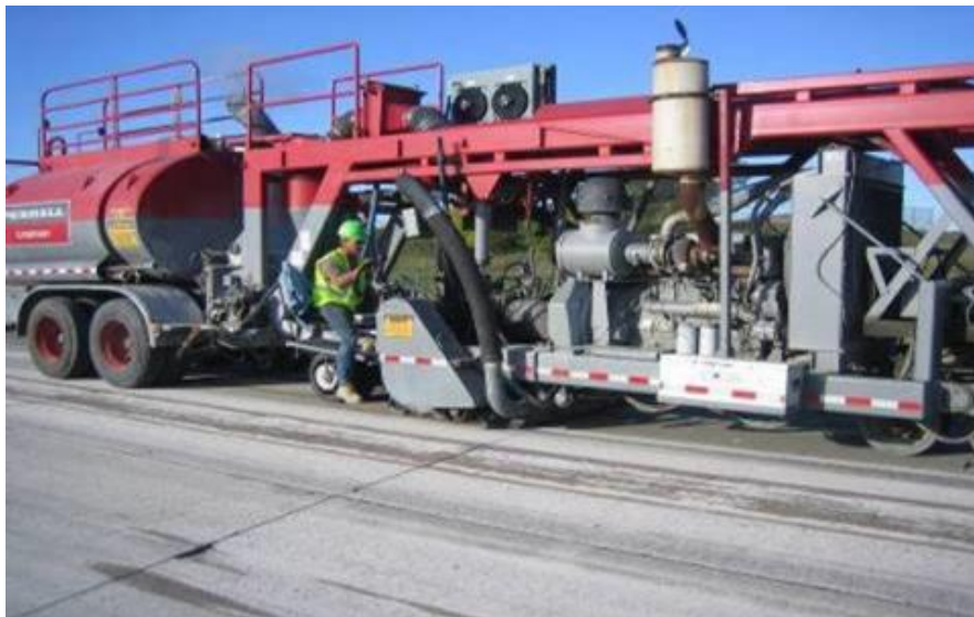
Figure 2.12: Grinding Process for Configuration of Cell 9: Ultimate Grind
