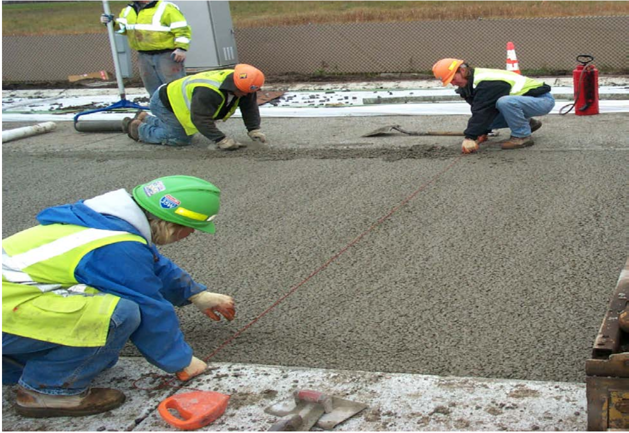
Figure 2.9: Establishing 10 ft. Joints in Cells 85 and 89
