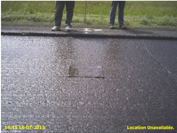
Figure - Site 1 - first tack on milled surface, NB Passing Lane.
