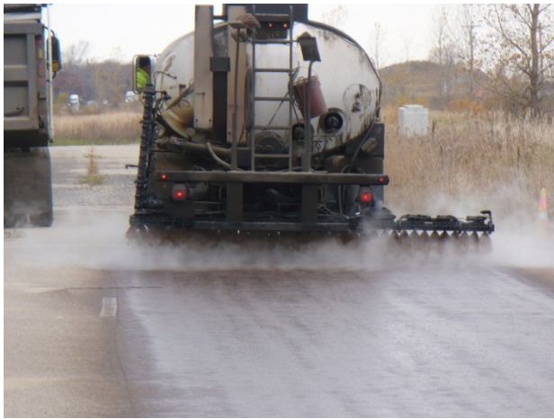
Figure 4 Distributor operations on the High Tack section.
