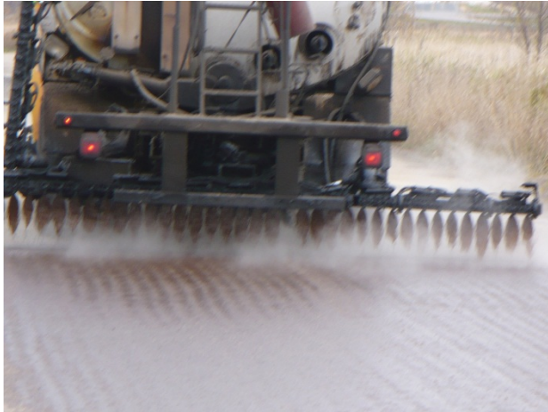
Figure 3 Distributor operations on the Standard Tack section.
