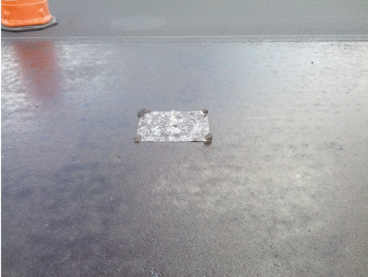
Figure - Site 2 - after 2nd tack, NB Passing Lane.
