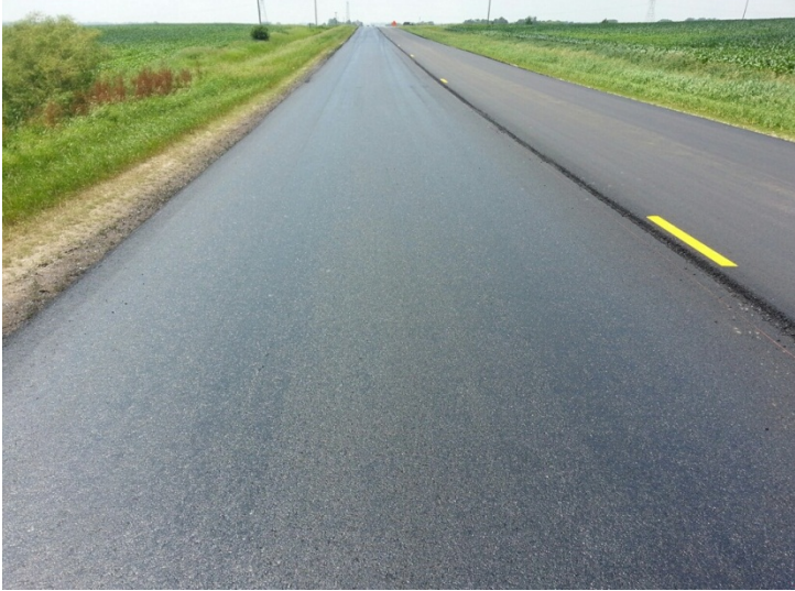
Figure - CSAH 11 STA 47+50 Left Lane on Tight Blade.
