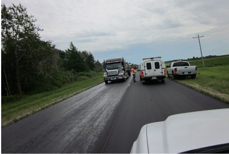
Figure - CR73 Paving Train.
