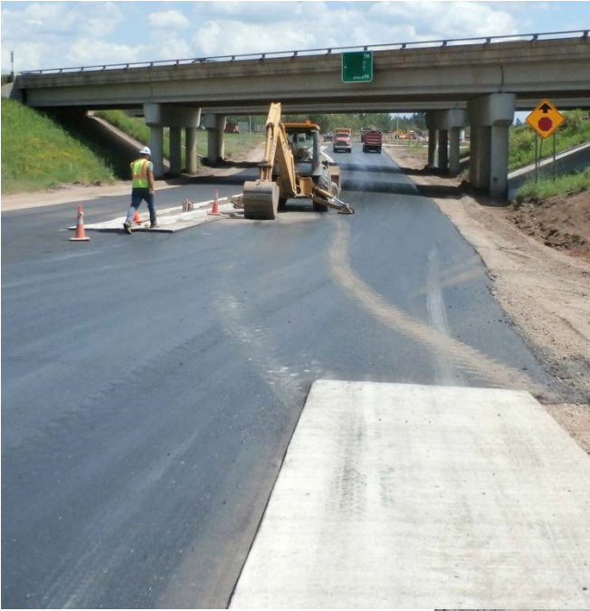
Left: Backhoe Operations at soft spot (notice dirt pile)
