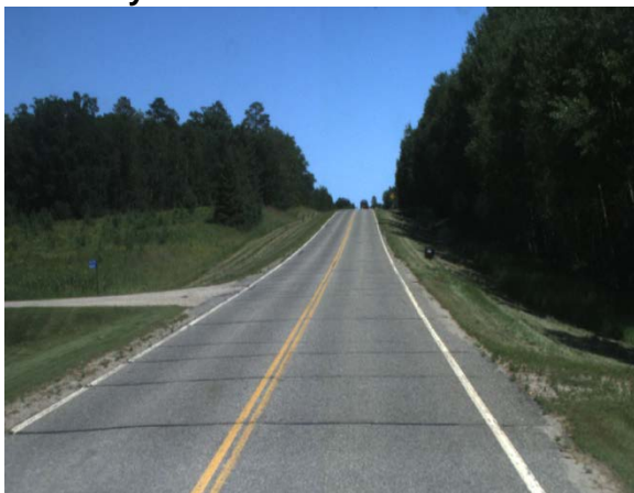
Figure - Preconstruction view of Beltrami CSAH 22 at RP 9.3, looking east. Image from PM video file.
