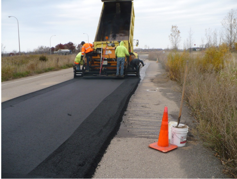
Figure 6 Paving the High Tack section.
