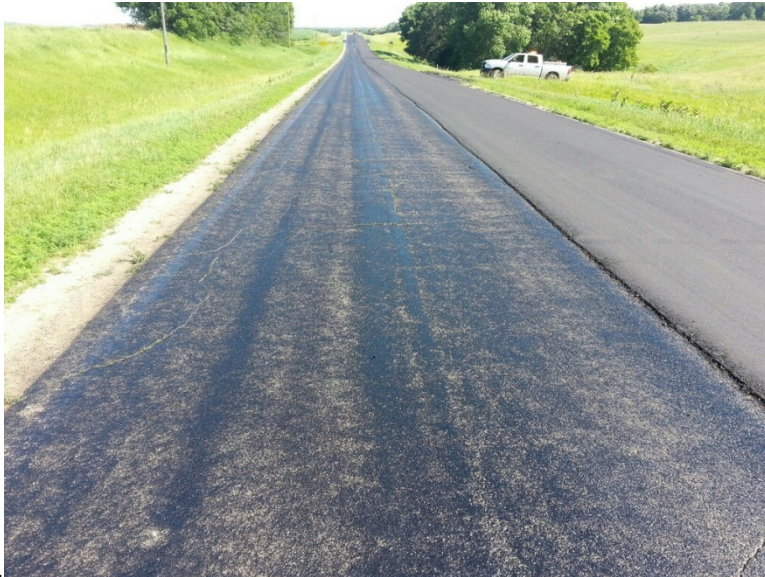
Figure - CSAH 21 STA 46+00 Left Lane on Existing Pavement.
