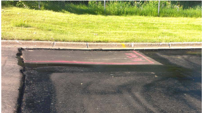
Figure - Ramp area with wand-applied tack.
