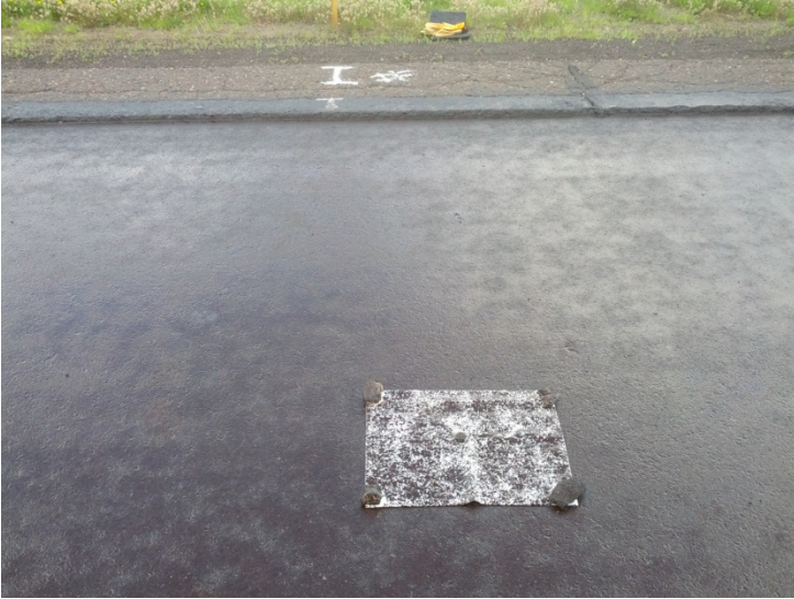
Figure - Site 1 - after 2nd tack, NB Passing Lane.
