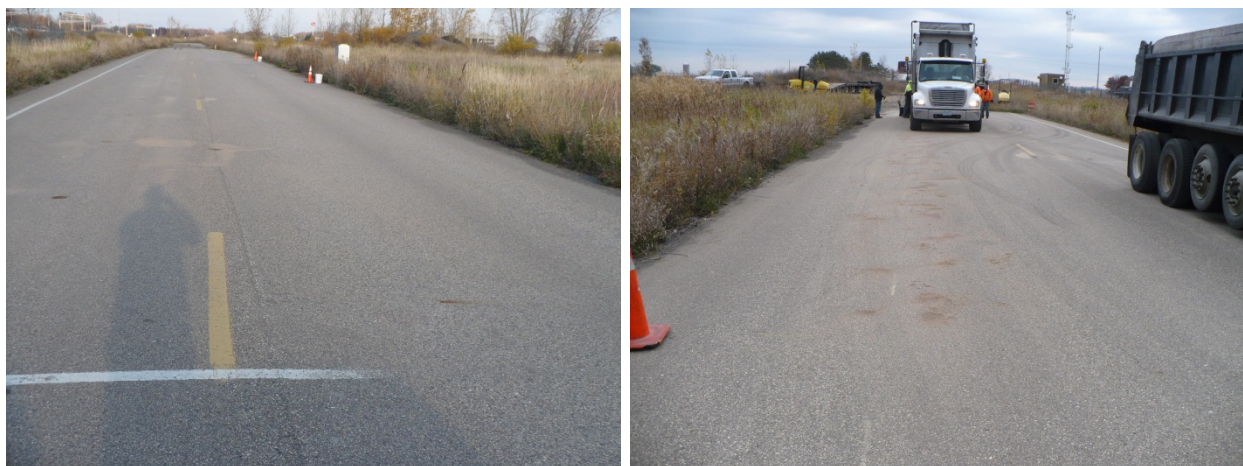
Figure 2 Appearance of the No Tack section before and after contaminant.
