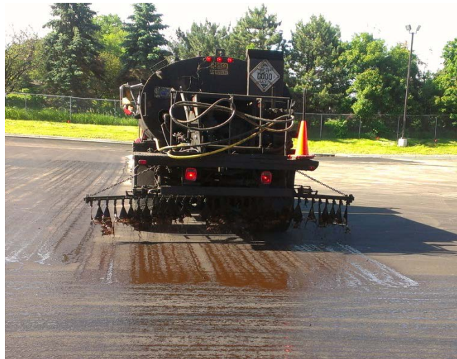
Figure - Distributor applying tack.
