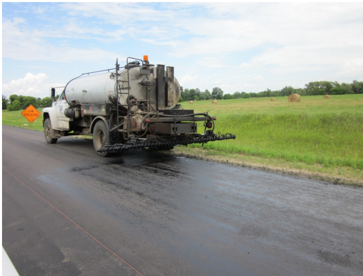
Figure - CR73 Distributor finishing application.
