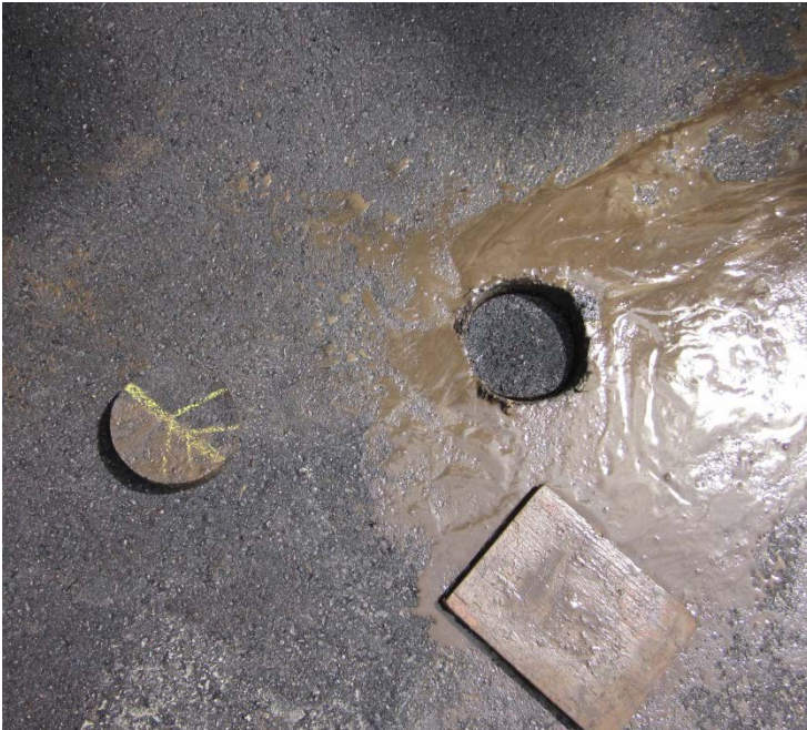
Figure - Core Bond to Base exceeds tight blade layer bond.
