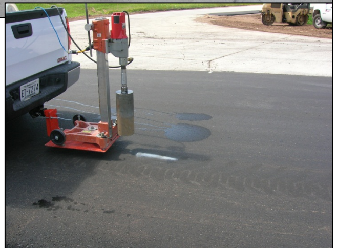
Figure – Top and Center: Haul Trucks dropping dirt Below: Coring LWP of area
