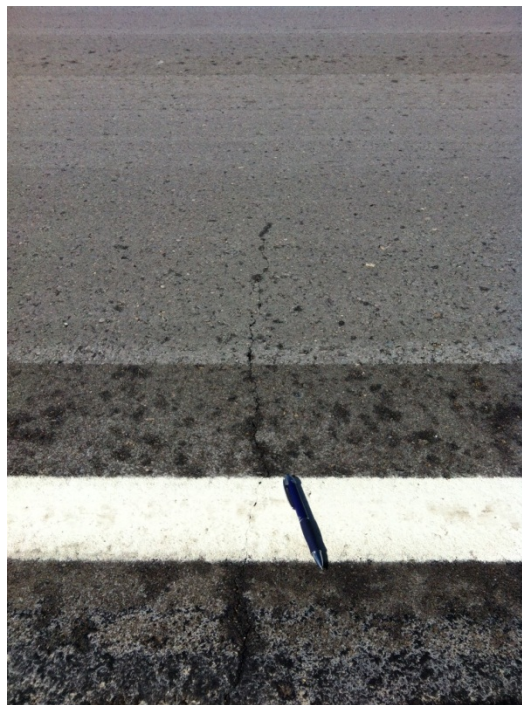
Figure 4.2: TH 56 SFDR (represents typical cracking on reclaims)
