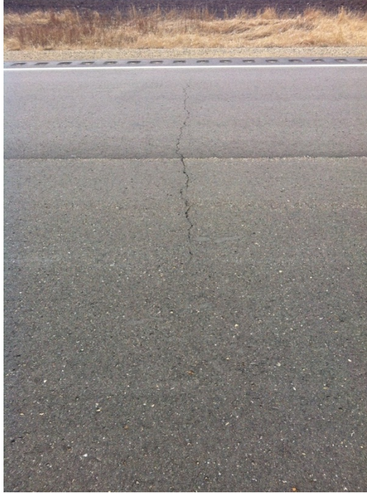
Figure 4.1: TH 69 Mill and Overlay (represents typical cracking on mill and overlay sections)
