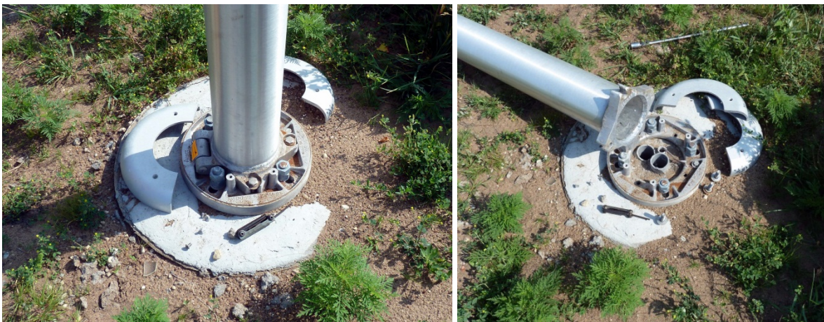
Figure 1.4 Hinged-Pole Base Mechanism
