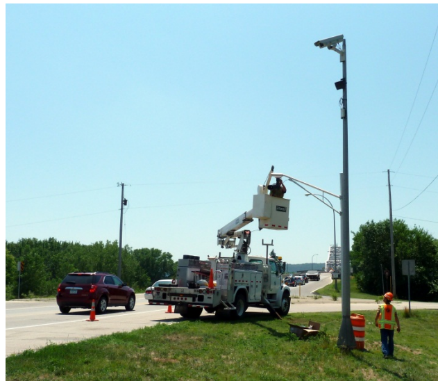
Figure 1.6 Camera Aiming with Bucket Truck
