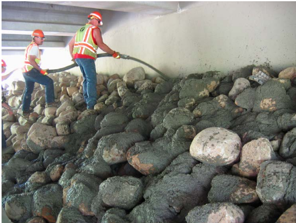
Figure 3.1 -Grout application at Bridge No. 48030, Milaca, MN
