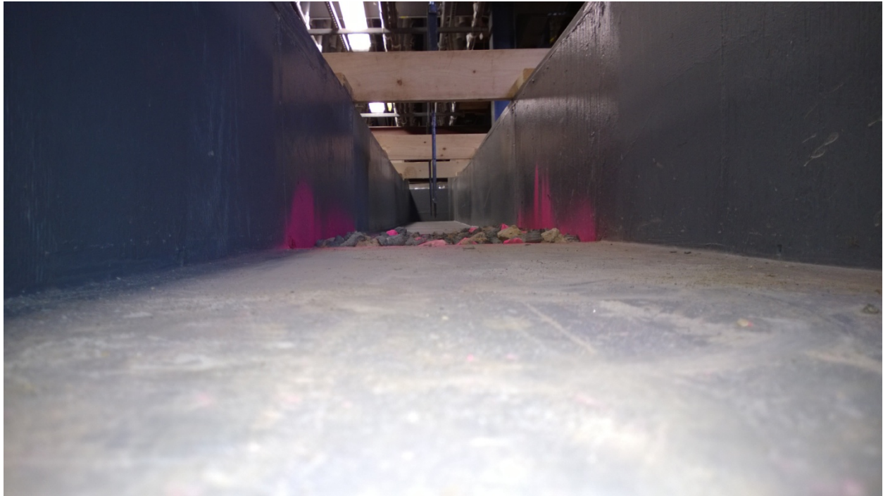
Figure 6.4. Flume floor from downstream to upstream.
