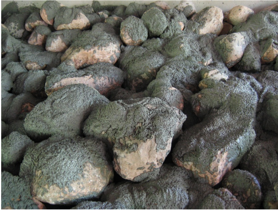
Figure 3.2 - Matrix riprap at Bridge No. 48030, Milaca, MN
