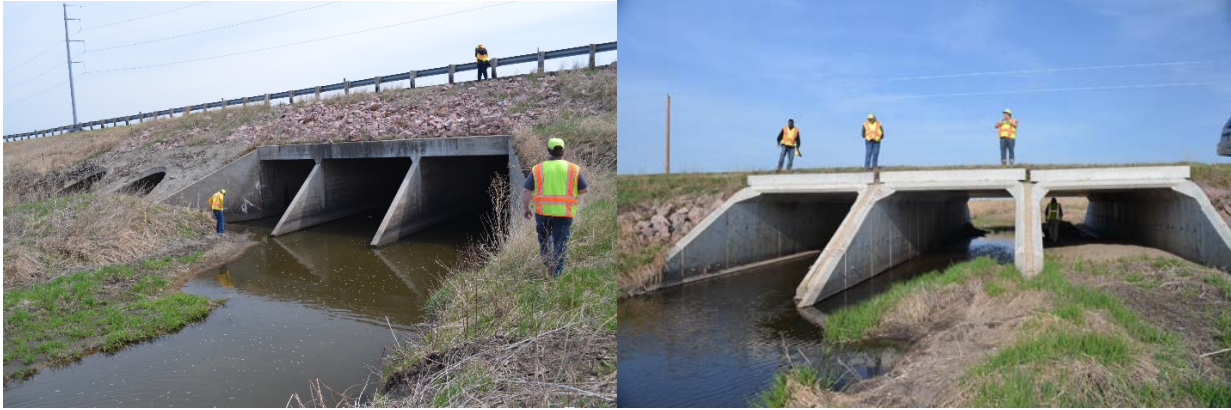
Figure 4.8. Sediment deposition and vegetation growth upstream of multibarrel box culverts: Beaver Creek and I-90 (left), and Kanaranzi Creek and Edwards Ave (right) in southwest MN.
