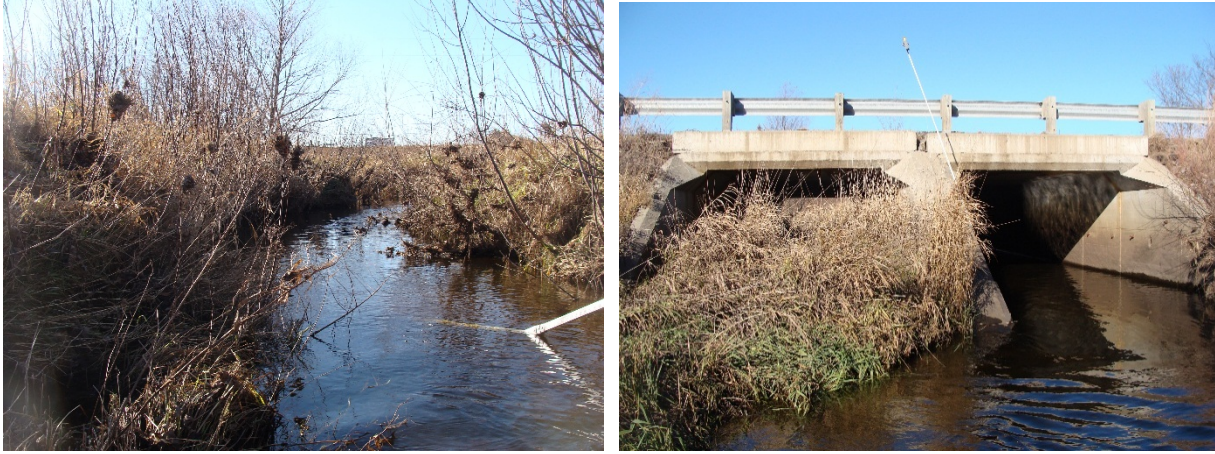
Figure 2.6. Photos of culvert on Stoney Brook.
