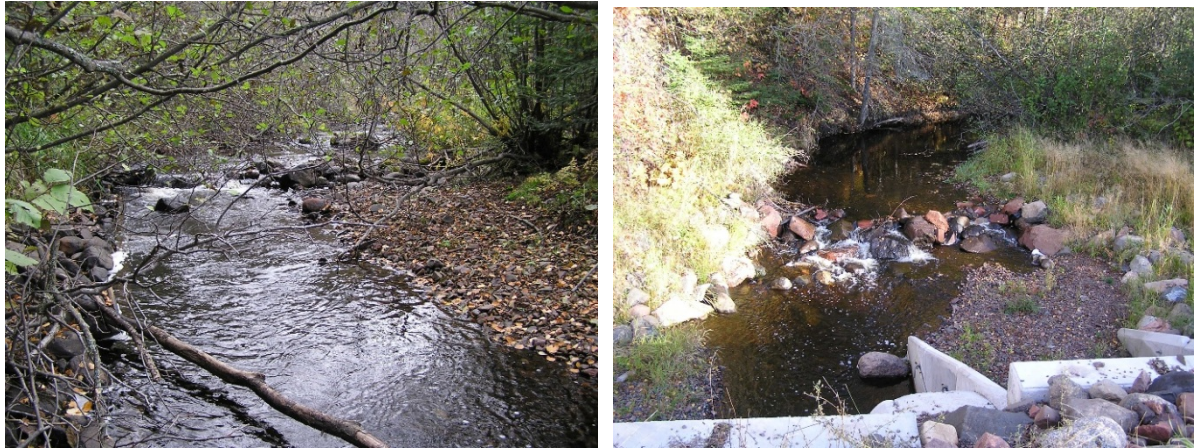
Figure 2.8. Photos of culvert on Kimball Creek (Hansen et al. 2011).
