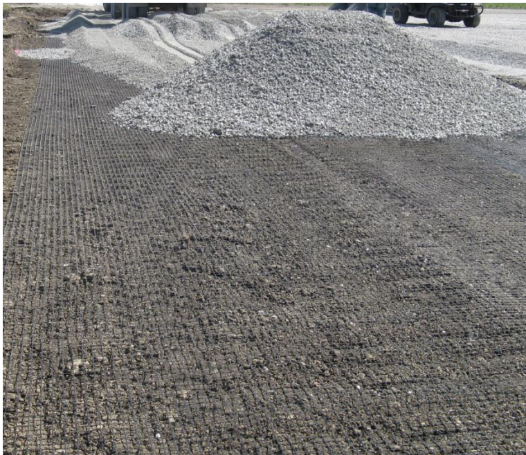
Figure 6. Biaxial Geogrid Placed at the Interface of Subgrade and Base Layers for Stabilization
