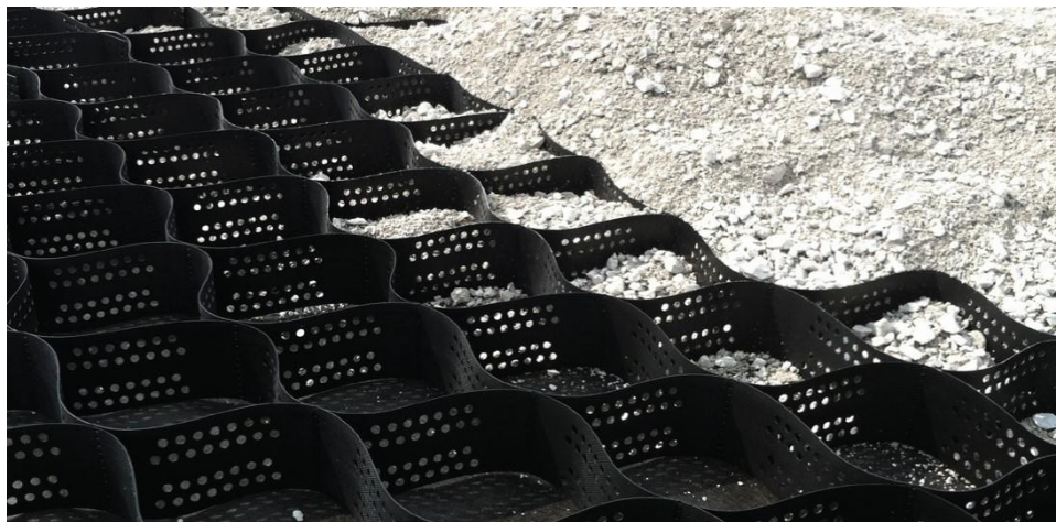
Figure 8. 6-Inch Geocell over Non-Woven Geosynthetic Layer Placed on Subgrade
