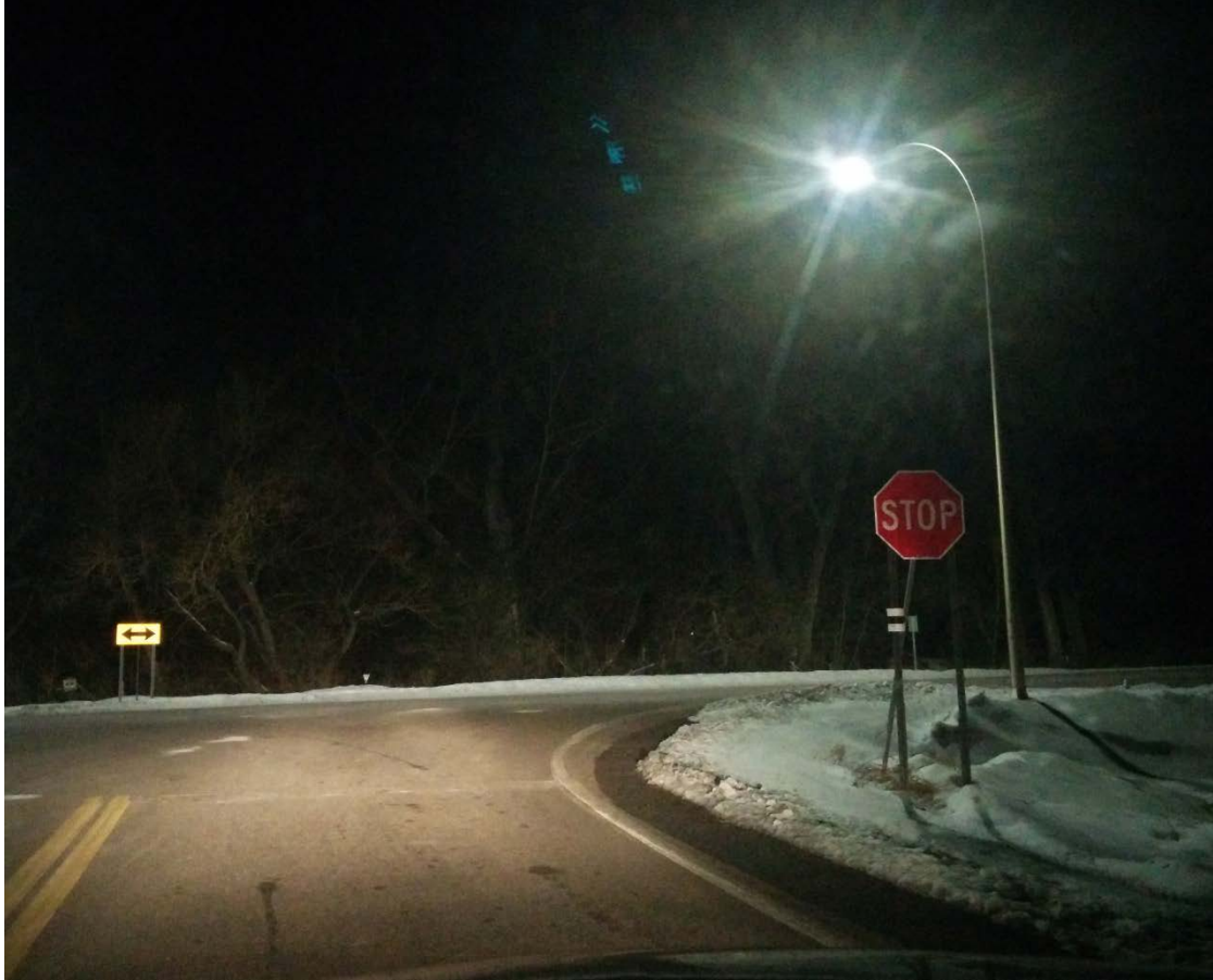
Figure 7. Rural through-stop intersection with Light Emitting Diode (LED)
